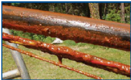
Figure 3. Biofilm on well wiring
