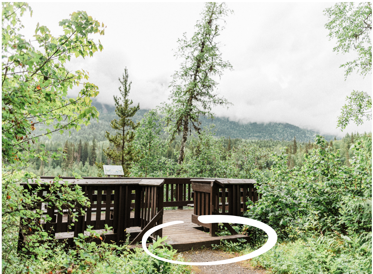
An example of a threshold where a trail transitions to another infrastructure surface.
