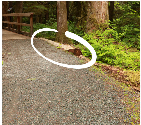
An example of stabilization at the corner of a bridge.
