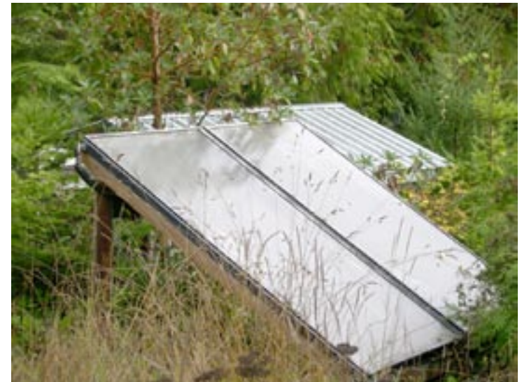
Above: Solar energy used to heat water. Photo: Secret Sea Resort
