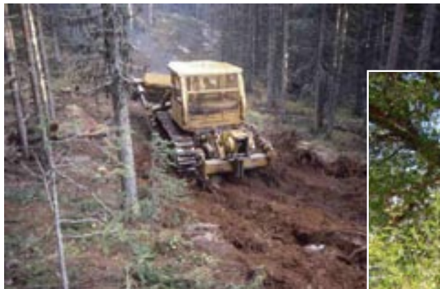
Above: Road construction using minimum width and routing to avoid impacts
