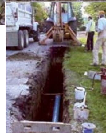
Above: Service line buried to blend into natural setting.
