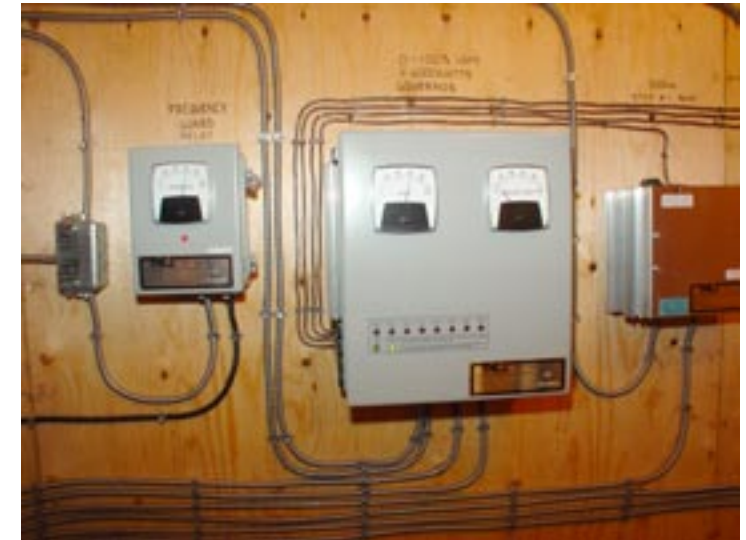
Above: Gauges to measure output from micro hydro generator
