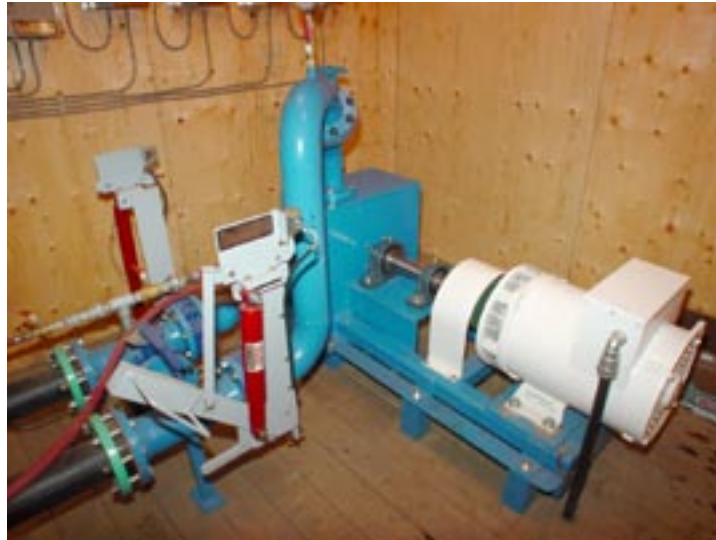
Above: Compact micro hydro generator
