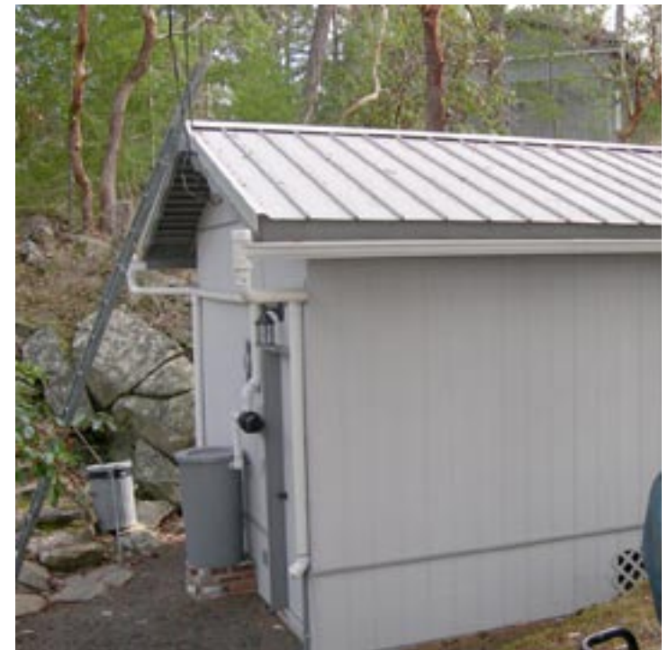
Above: Rain water collection system used as alternative water source Photo: Secret Sea Resort
