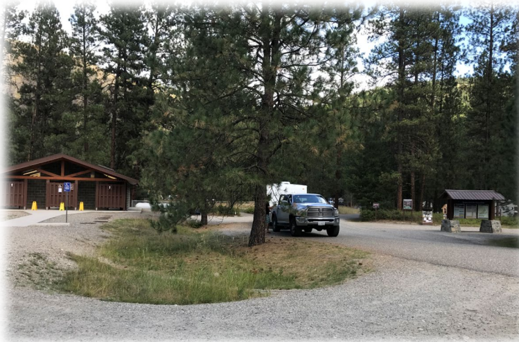
Plate 10: The toilet/shower building and main campground entrance at Kettle River Recreation Area
