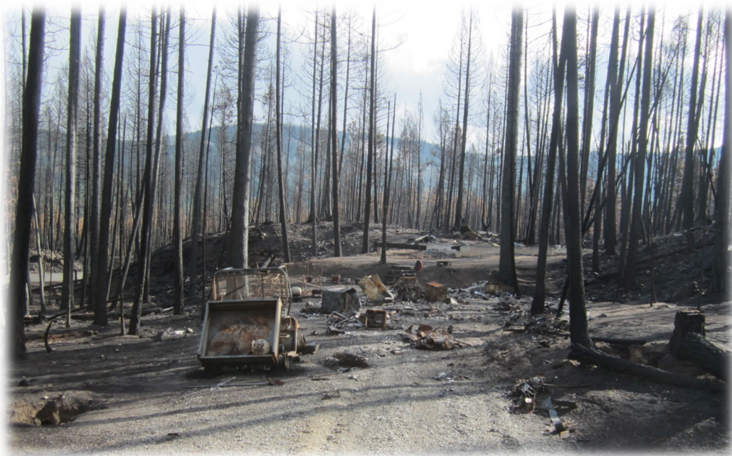
Plate 2: The 2015 post-fire remains of the park operator residence and maintenance facility
