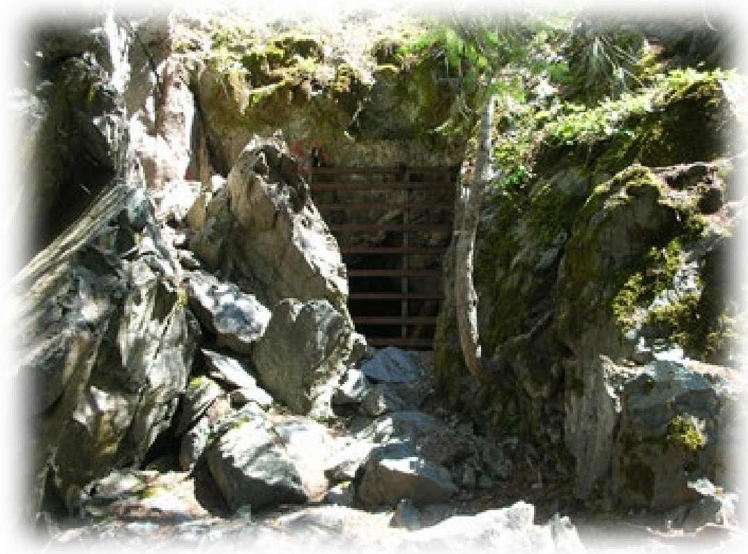
Plate 1: A mine shaft opening which has been permanently closed by BC Parks
