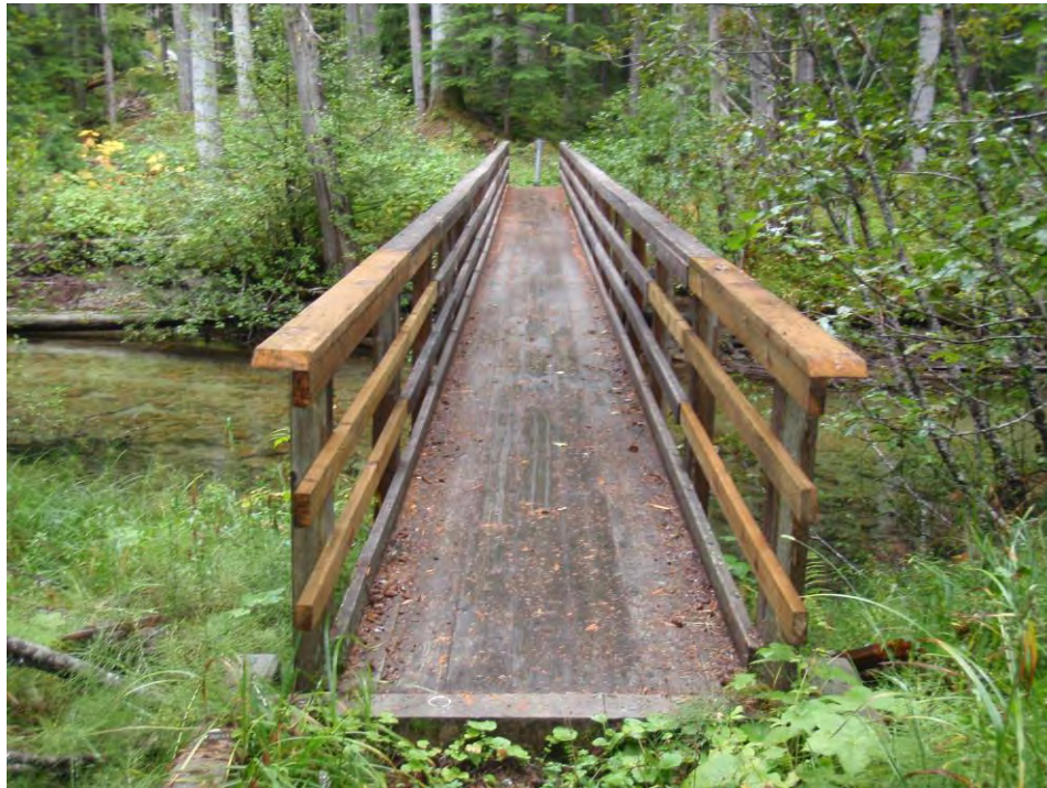
The Spectrum Creek bridge (50 metres from the trailhead parking lot)
