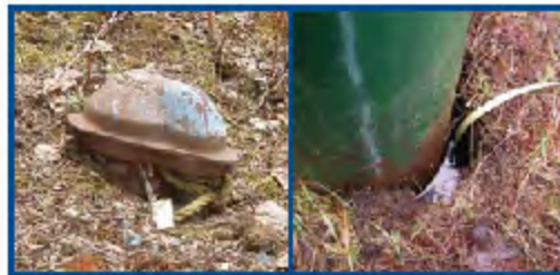
Figure 1. Well casing stick up less than 30 cm (12 inches) from the ground surface
