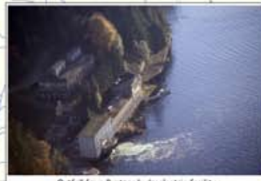
Outfall from Buntzen hydroelectric facility
