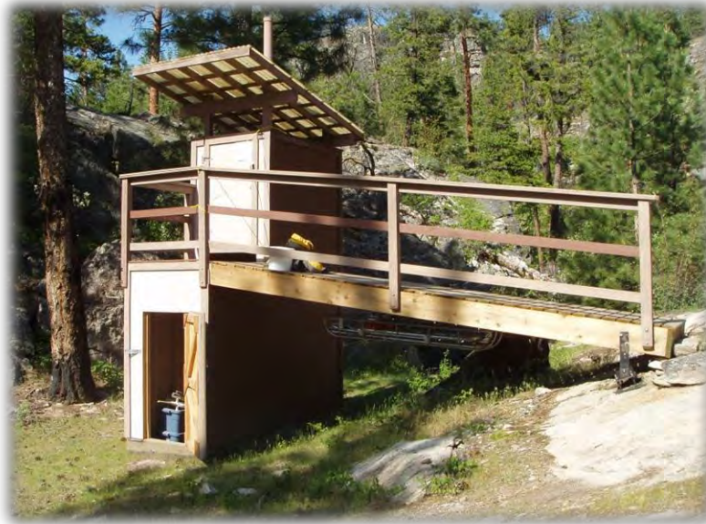
Plate 18: The composting toilet located within a high use climbing area of the park.
