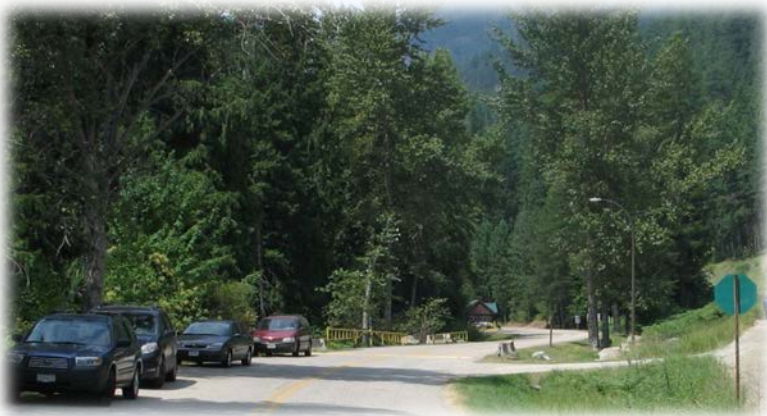
Plate 3: Broadwater Road at the intersection of Deer Park FSR (gatehouse in the distance).
