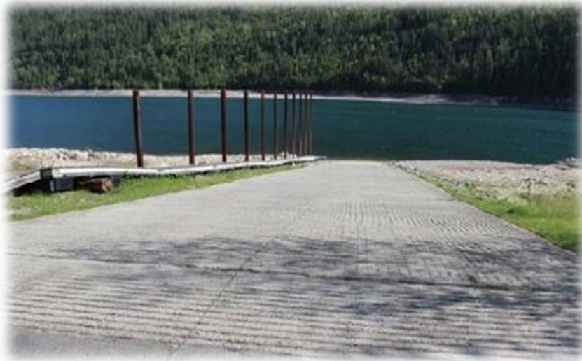
Plate 9: Concrete boat ramp within Syringa Park (maintained by BC Hydro).
