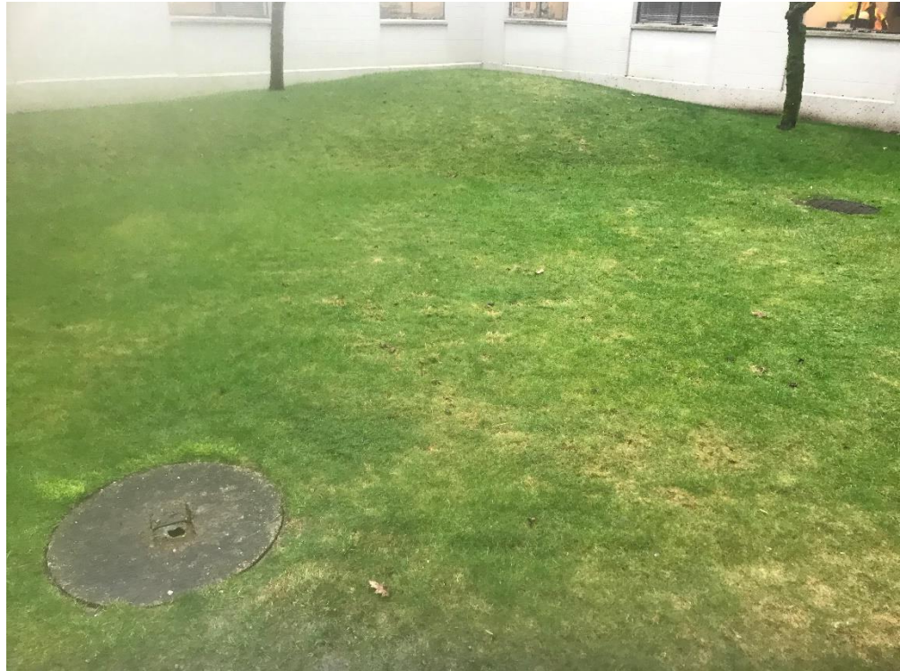
Photo 5: Location of septic tank not connected to the Site effluent system.
