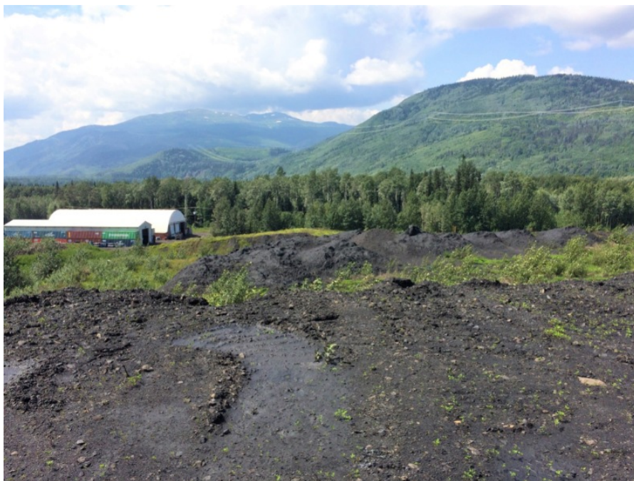
Photo 4 - The FCCR CCR Pile looking west from the top of the pile.
