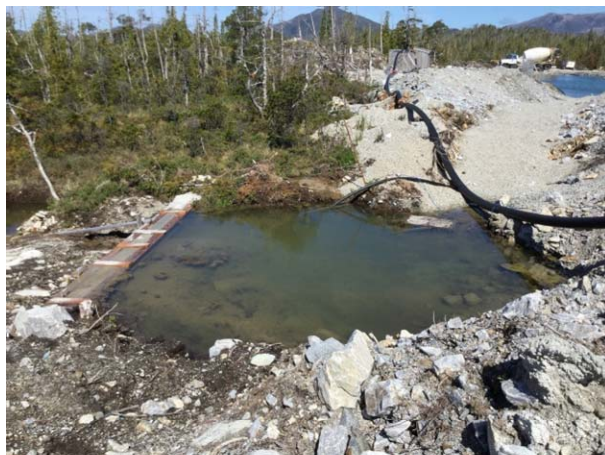
Photo 21: Small pond overflowing concrete dam.
