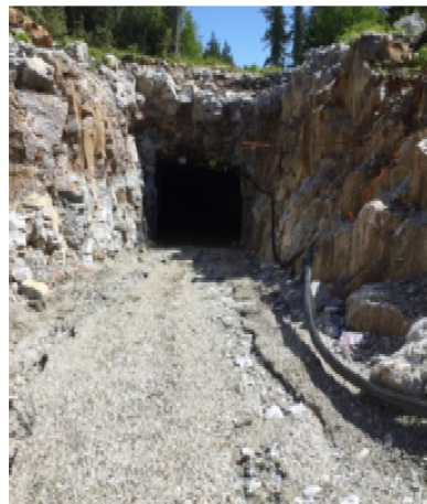
Photo 35: Riling of road surface at Tel portal
