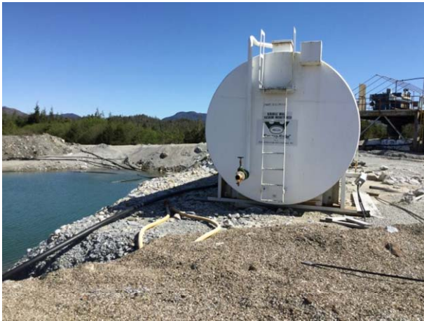
Photos 16 and 17: Leaking fuel tank adjacent to sediment pond. Note that the leak is on the far side of the fuel tank in the photo on the left. This photo is intended to show the proximity of the tank to the adjacent pond.
