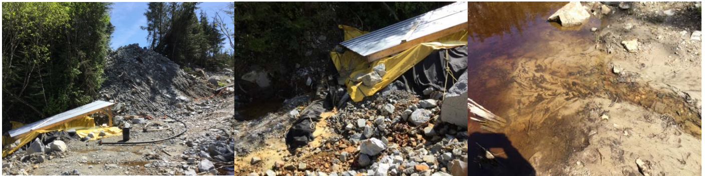
Photos 24, 25, and 26: The series above shows the seepage collection pond collecting water from the old Bob stope, seepage escaping out the back of the pond, and flowing to an adjacent wetland.
