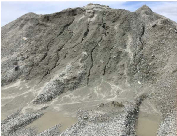
Photo 34: Erosion of the low grade ore stockpile
