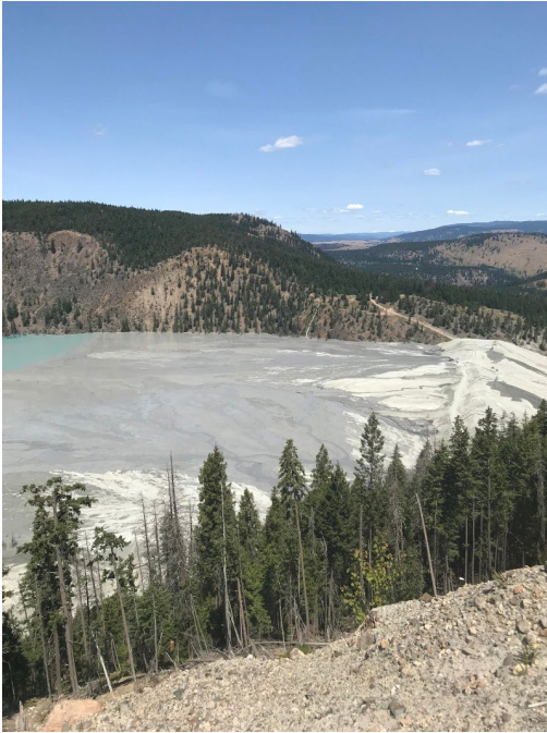
East end of TSF tailings beach. The small waterfall in the mid-background on the forested slope is the seepage return circuit.
