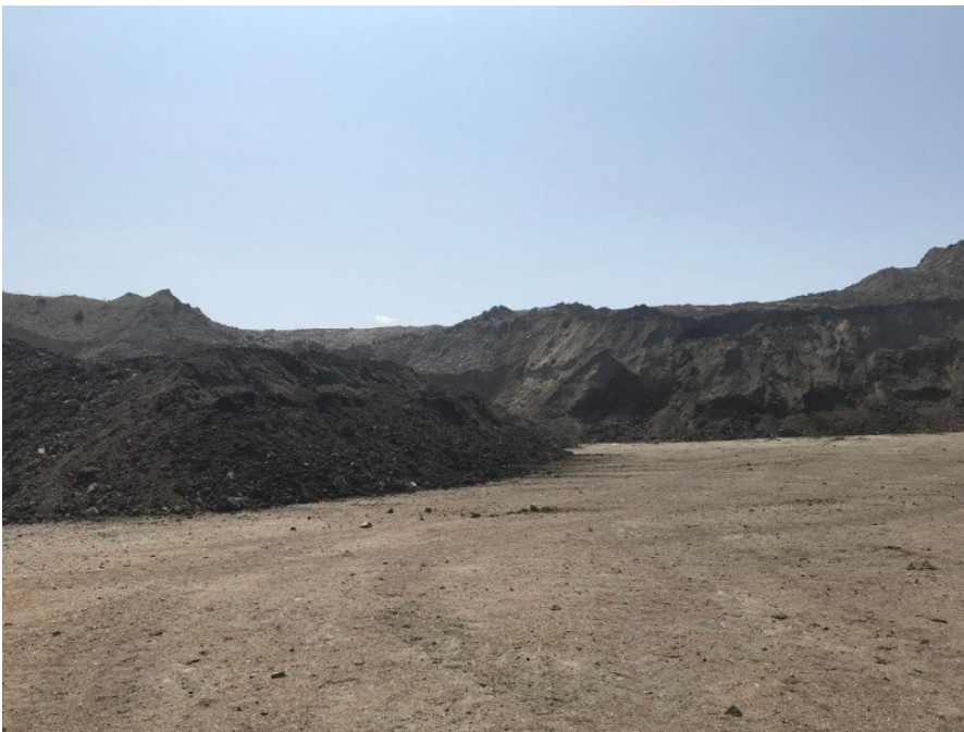
On the right is the South Soil Stockpile and on the left is the finished soil stockpile made of a mix of amendment and salvaged soil
