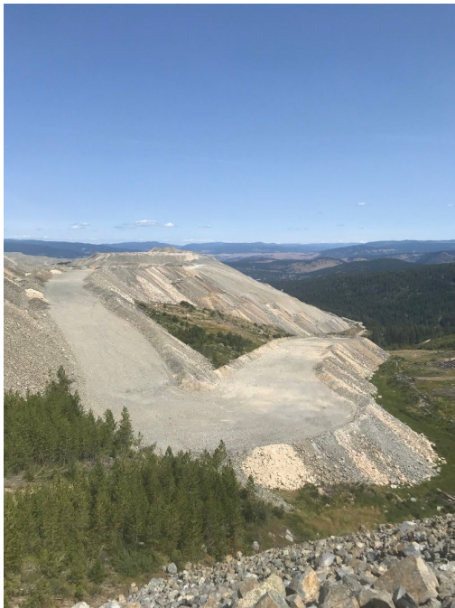
The long slope in the background as been resloped with a rough surface texture and will be seeded in 2019
