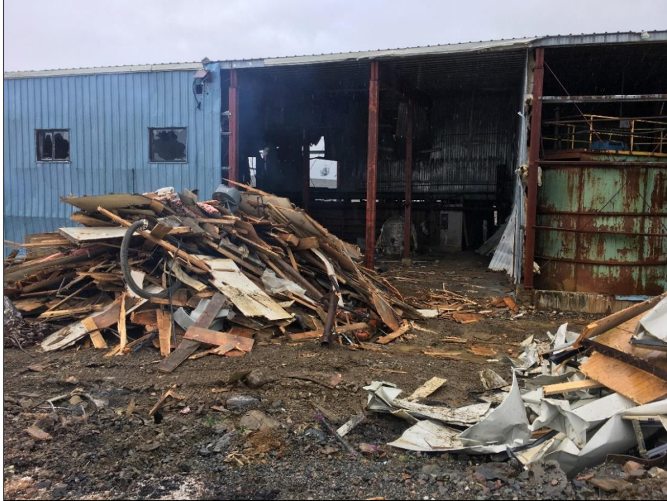
Photo 4.1-3: Construction waste sorted and disposed of appropriately.
