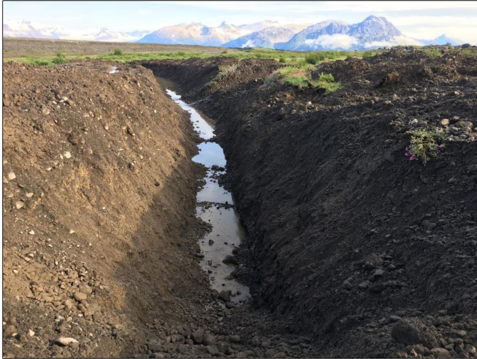
Photo 3.1-1: Diversion ditch excavated on east (higher elevation) side of Old Tank Farm in 2019.
