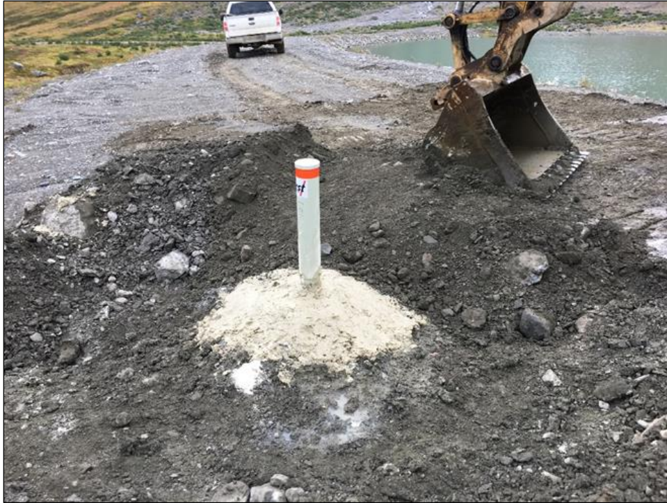
Photo 4.1-17: Bentonite added at base of DH17-05.
