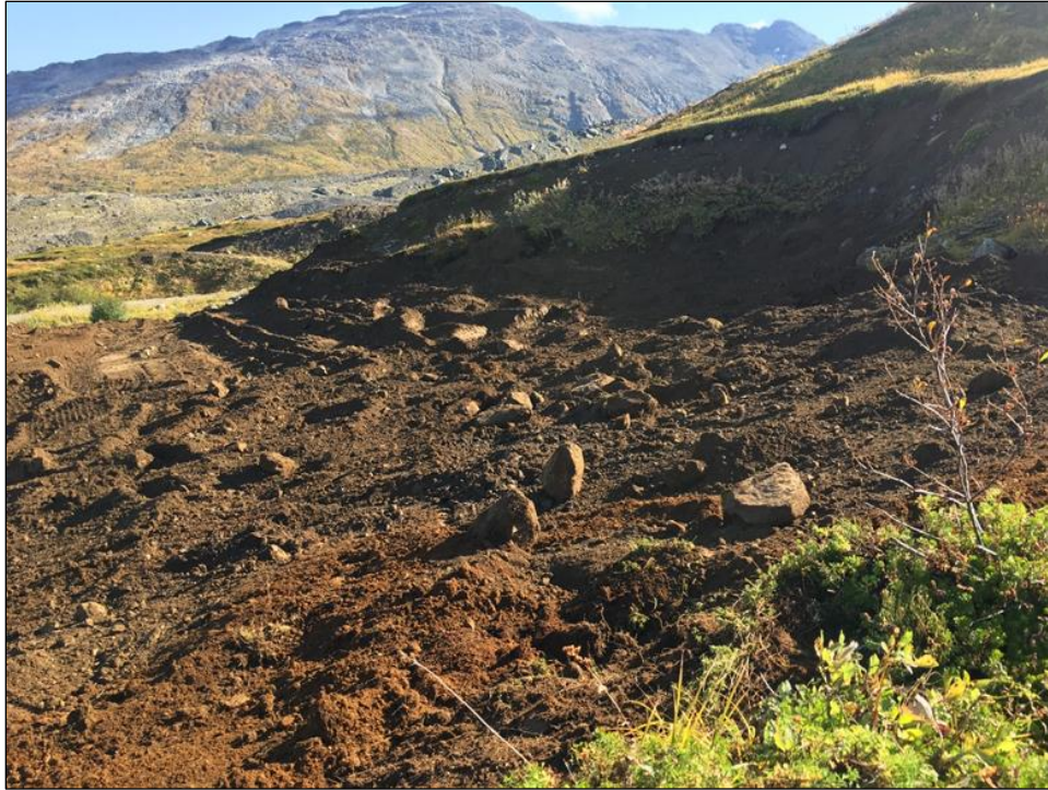
Photo 4.1-16: Portal 11 - Surface left rough and loose - seeded with reclamation seed mix.
