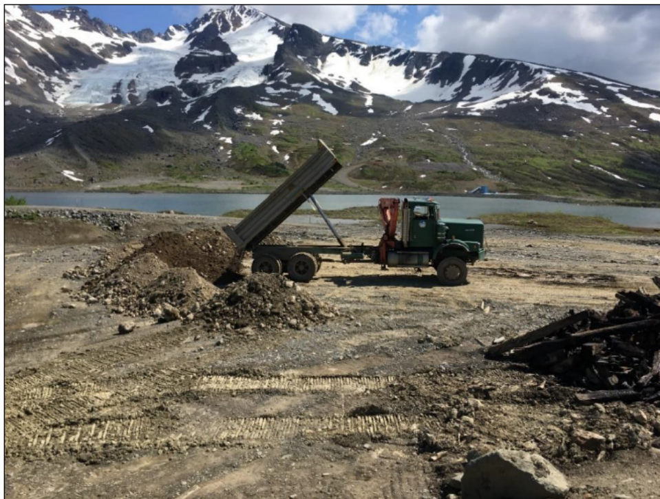
Photo 4.1-11: Gravel placed in Cell 2 for base levelling course (July 1, 2019).
