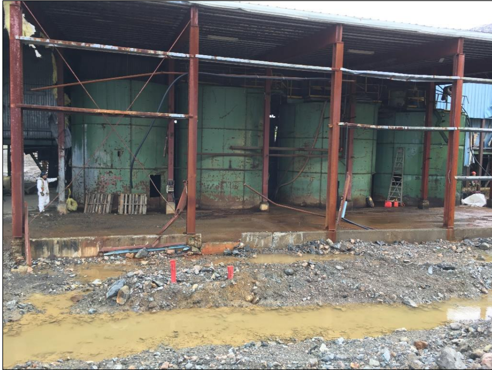
Photo 4.1-6: Cyanide tanks being deconstructed inside Mill Building.
