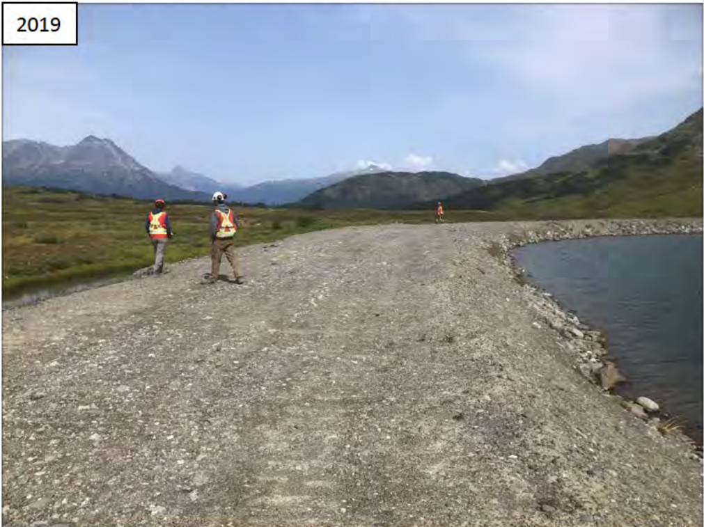
Photo I-7 Northwest Dam Crest (NW-4)
