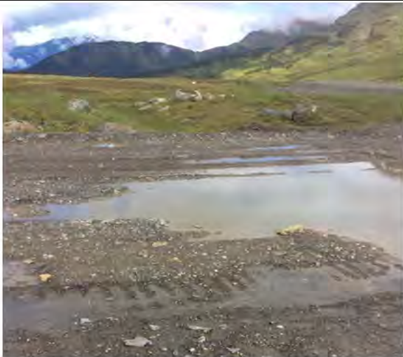
Photo 6: Vantage point photo along northern access road of the Main Landfill. Ponding of water was observed in this area.
