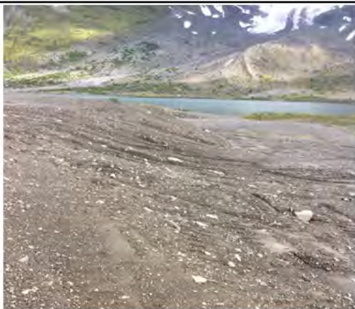
Photo 10: Vantage point photo of south edge of Main Landfill looking east. Minor erosion was noted on south slope of Main Landfill.
