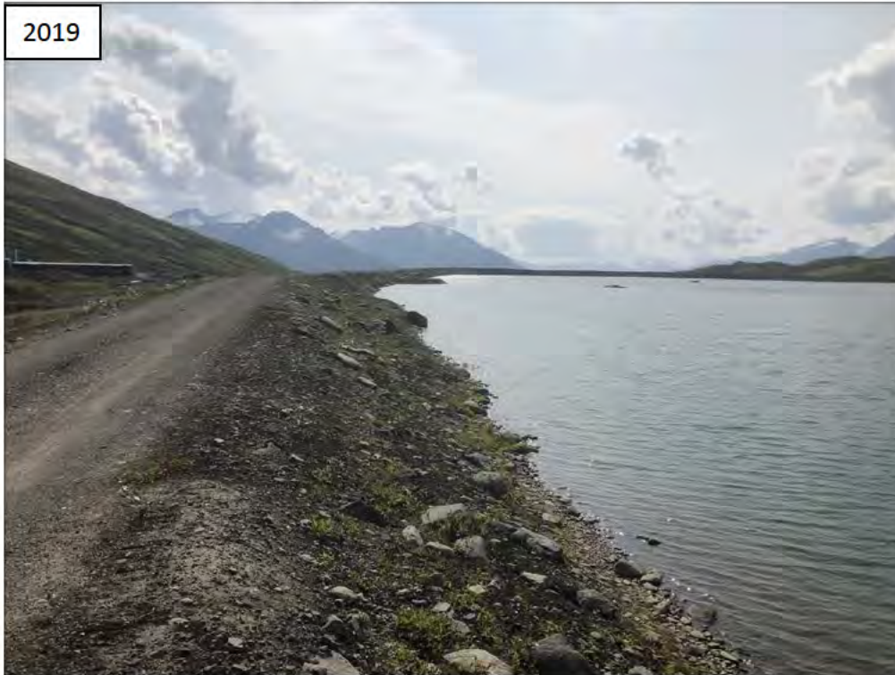
Photo I-15 Southeast Dam Upstream Slope (SE-3)
