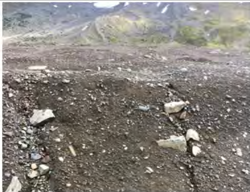
Photo 8: Vantage point photo along western slope of the Main Landfill looking east. Minor rill erosion was noted.
