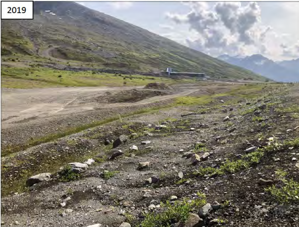
Photo I-13 Southeast Dam Downstream Slope and Ditch Line (SE-1)
