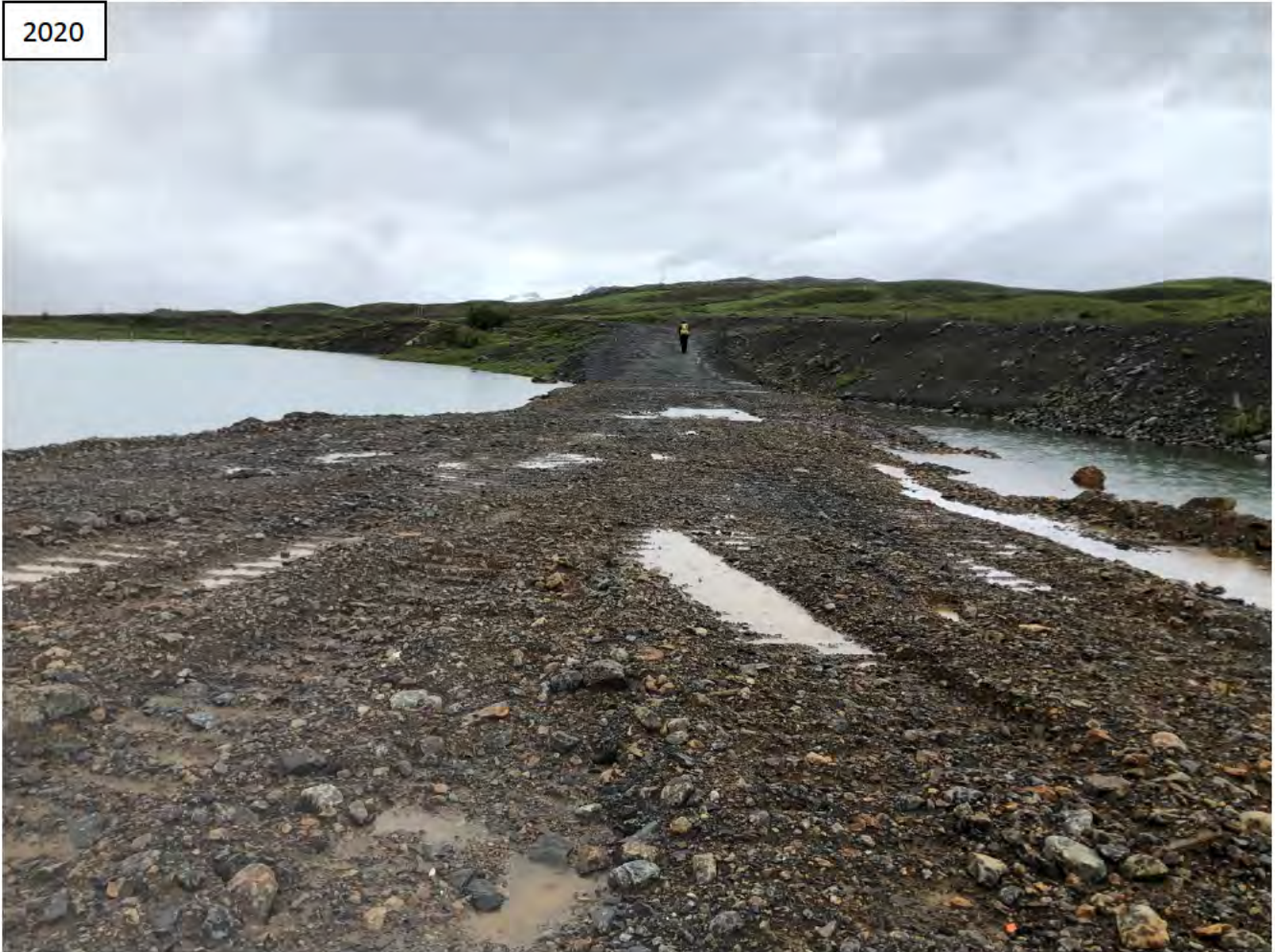
Photo I-2 Test Ramp onto TSF Surface from Northwest Dam (G-12)
