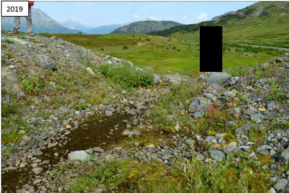
Photo I-11 Northeast Dam Spillway Looking East (NE-4)
