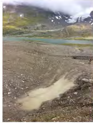
Photo 13: Vantage point photo of southwestern edge of Main Landfill looking east towards the culvert. Ponding water was observed in this area.
