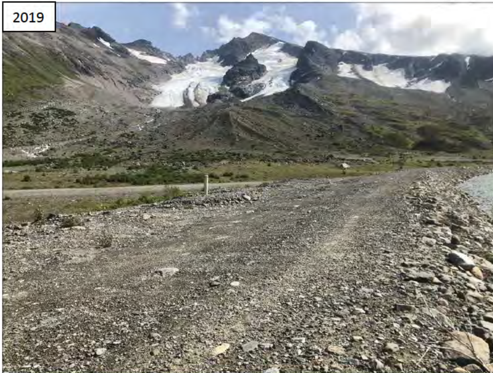
Photo I-12 Northeast Dam Crest by DH17-01 (G-2)
