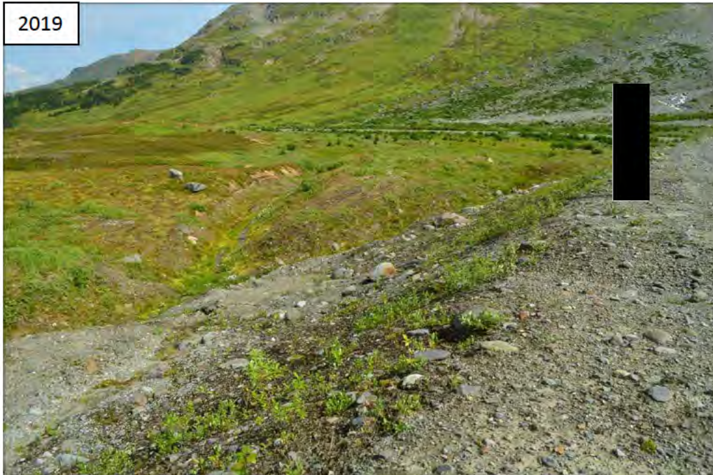
Photo I-8 Northeast Dam Ditch and Toe Line (G-1)
