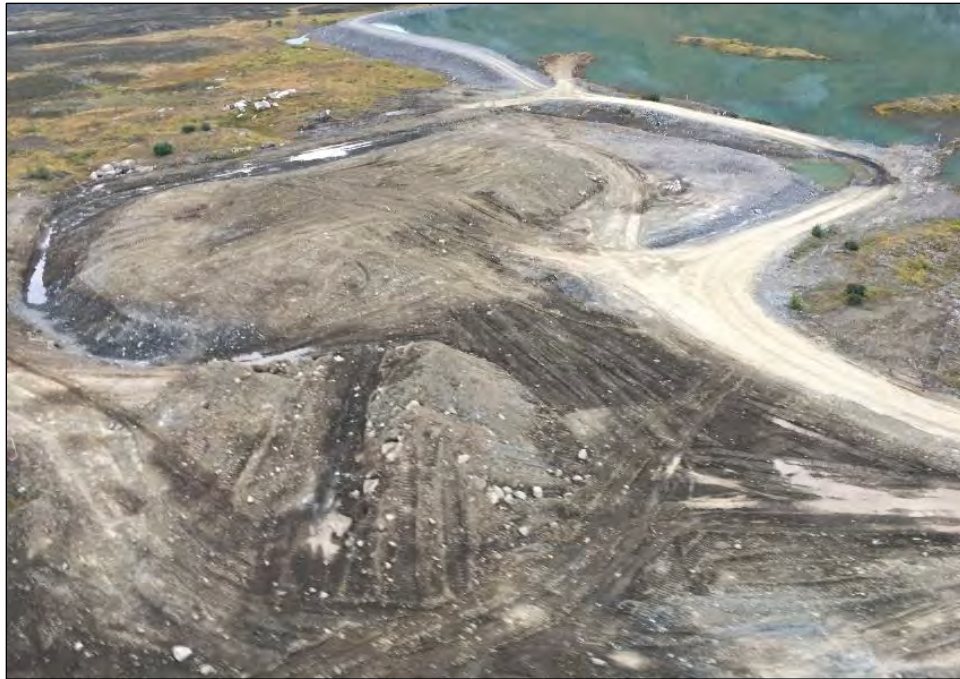
Photo 1.2-1: Johnny Mountain Mine Main Landfill in 2019 - after the addition of waste material gathered from the JMM area and the covering with mineral soils.
