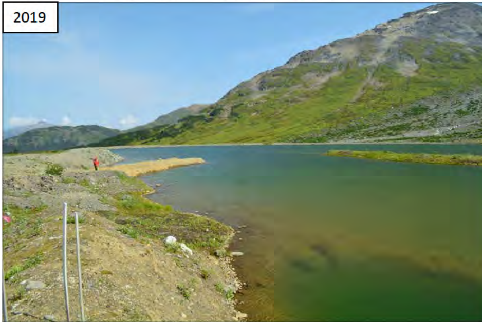
Photo I-1 Northwest Dam Abutment by Landfill (NW-1)
