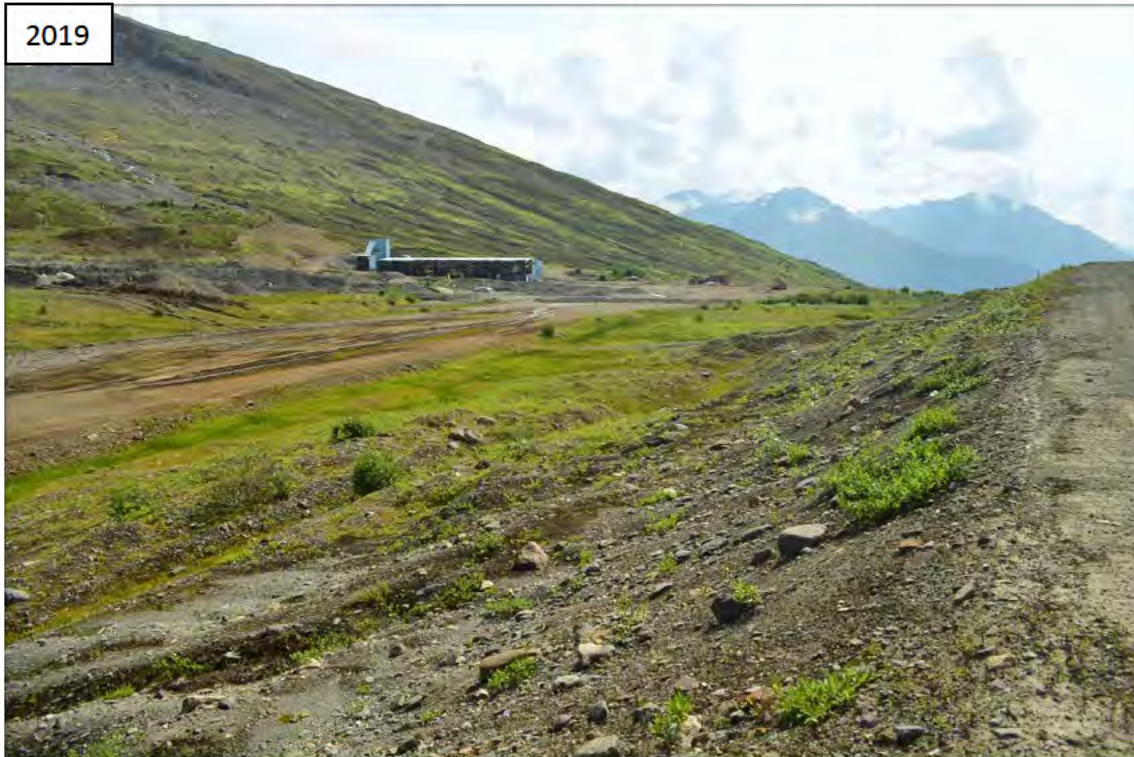
Photo I-18 Southeast Dam Downstream Slope and Ditch (SE-6)
