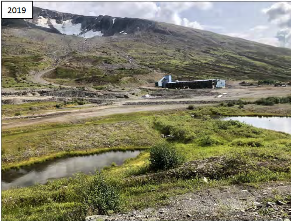
Photo I-26 Seepage Collection Pond at Southeast Corner (G-6)
