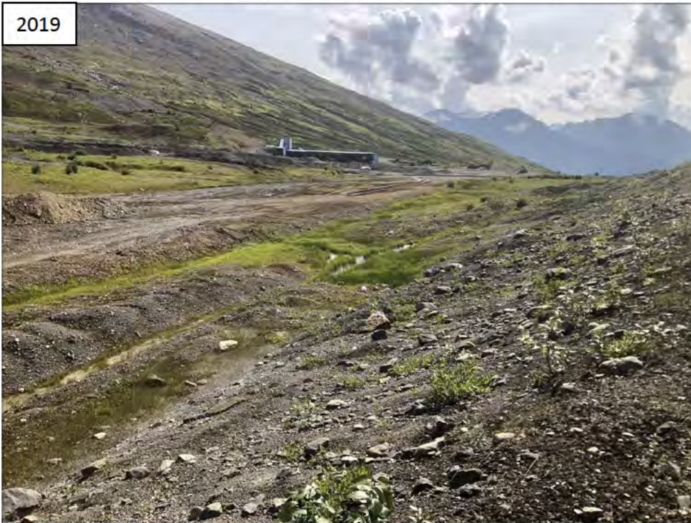
Photo I-19 Southeast Dam Downstream Slope and Ditch (G-3)
