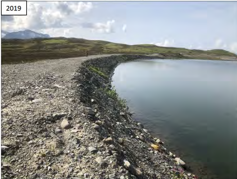
Photo I-22 Southwest Dam Upstream Slope (SW-1)
