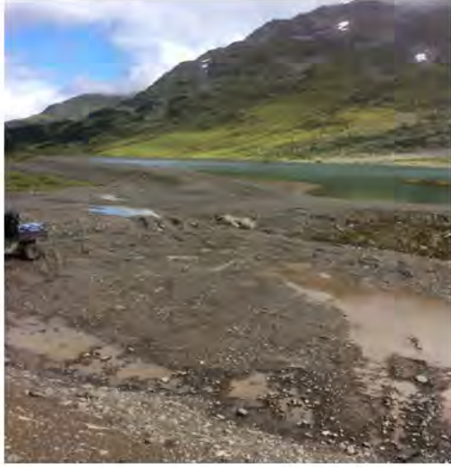
Photo 12: Vantage point photo of northeast corner of Main Landfill looking northeast. Minor ponding water was observed in this area.
