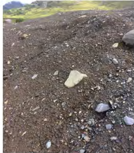
Photo 7: Vantage point photo along western slope of the Main Landfill looking northeast. Minor rill erosion was noted.
