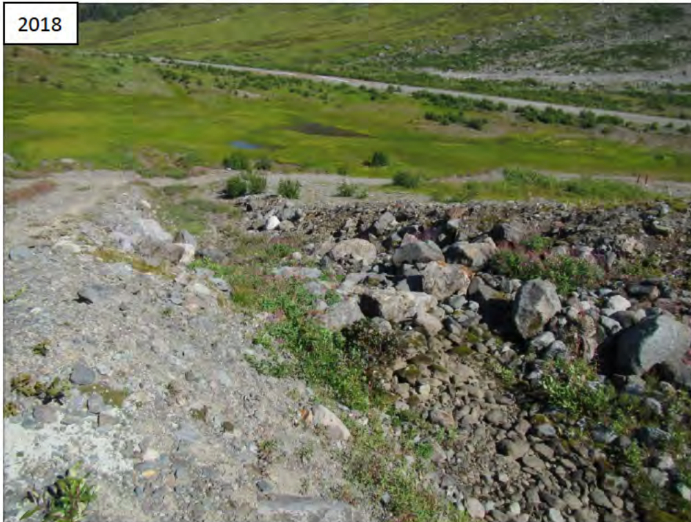
Photo I-34 Spillway Channel Outlet (S-2)
