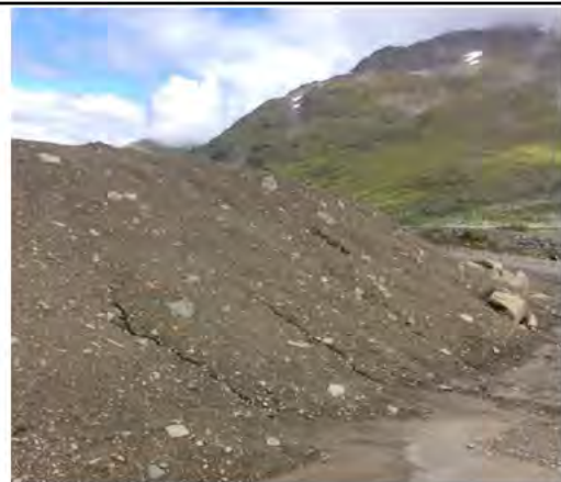
Photo 11: Vantage point photo of south edge of Main Landfill looking northeast. Minor erosion was noted on south slope of Main Landfill.
