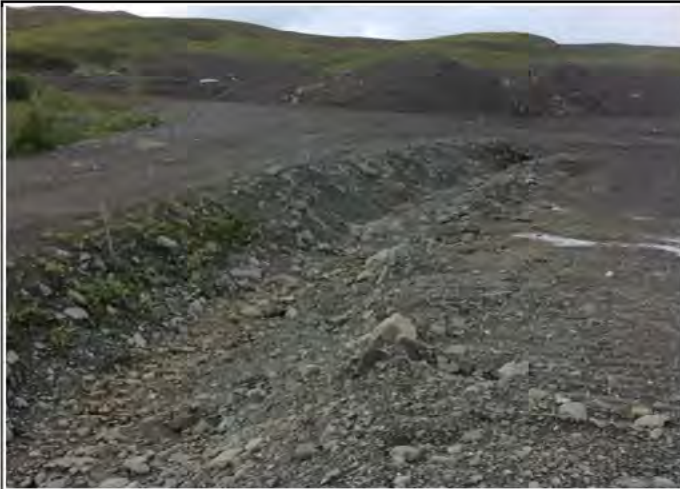
Photo 2: Vantage point photo of southeast Corner of Cell-2 looking northwest. South ditch east of culvert observed to be dry.
