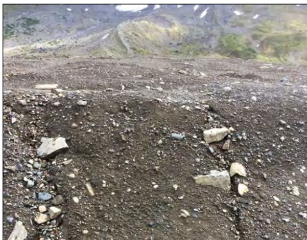
Photo 8-3: Vantage point photo along western slope of the Main Landfill looking east. Minor rill erosion was noted.
