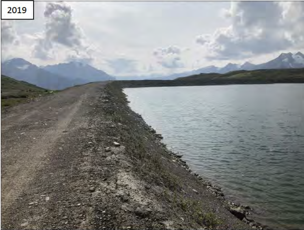
Photo I-20 Southeast Dam Upstream Slope Looking South (G-4)
