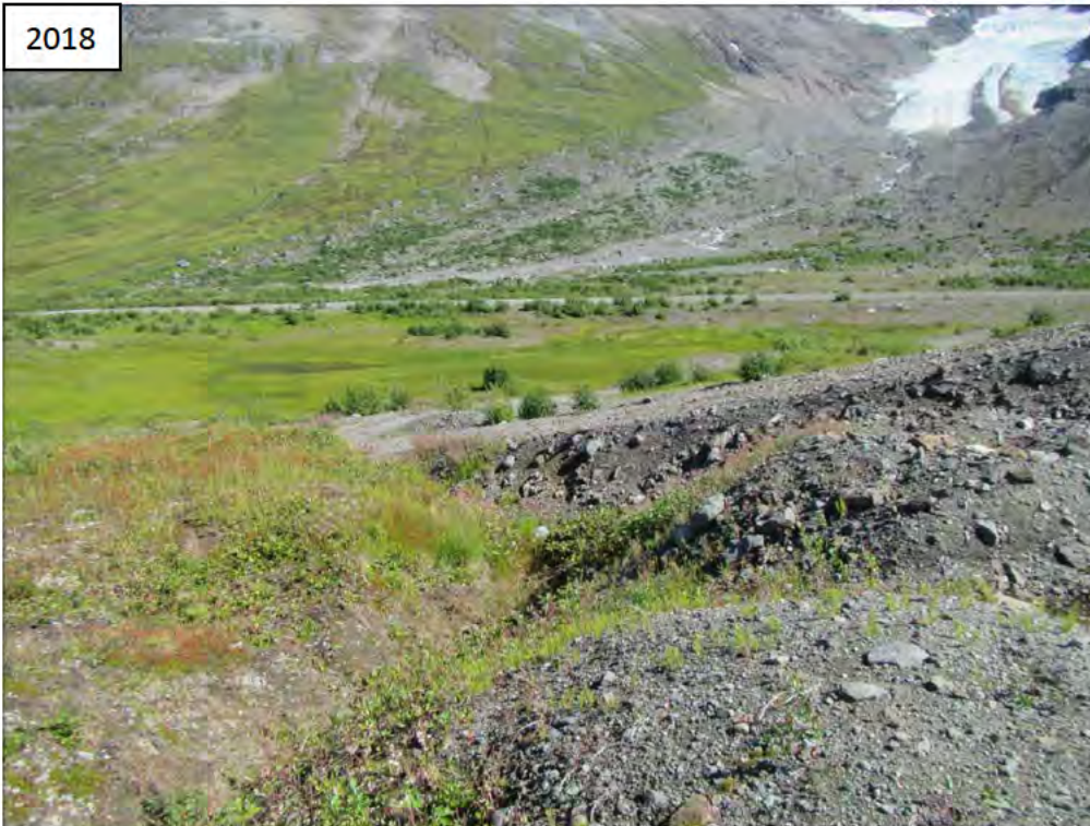
Photo I-10 Northeast Dam Downstream Slope Approaching Spillway (NE-3)
