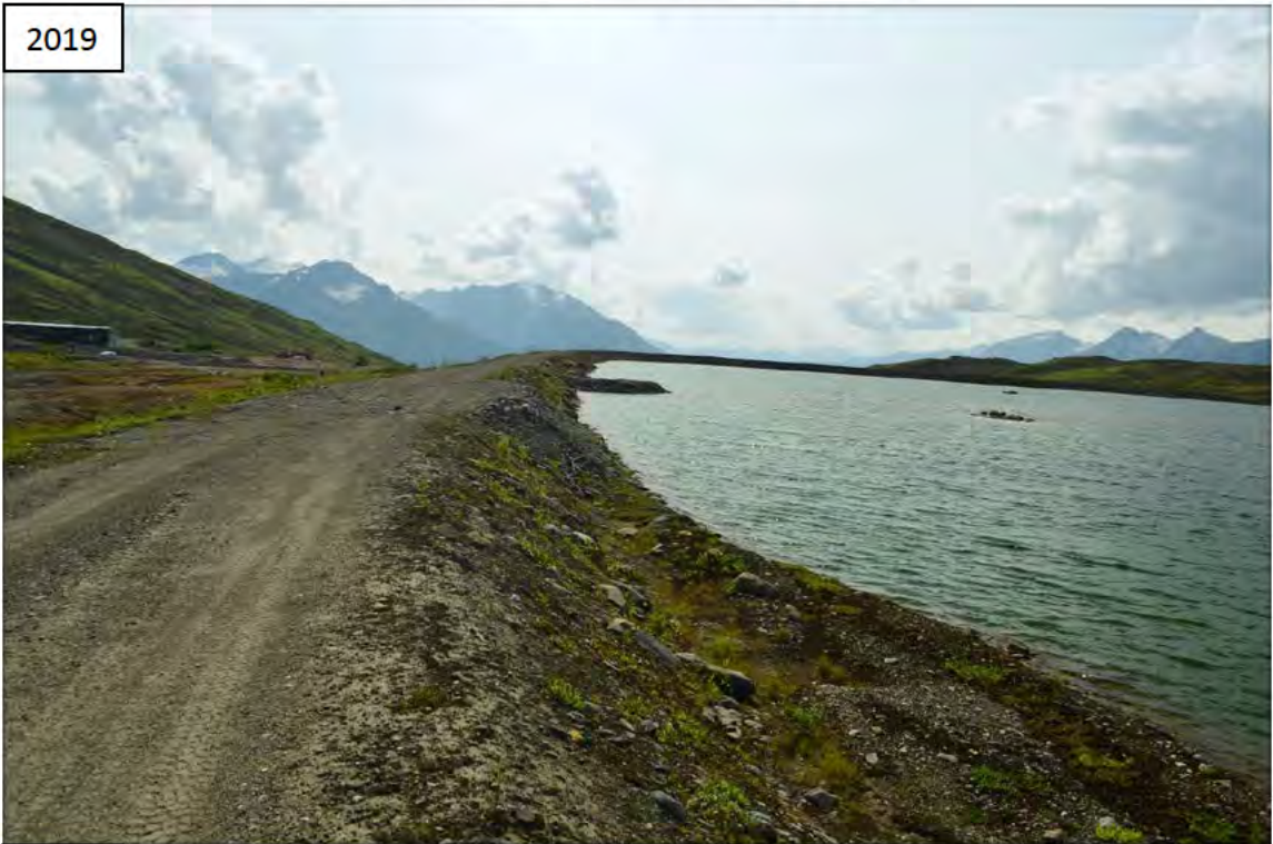
Photo I-16 Southeast Dam Looking South at Test Fill (SE-4)
