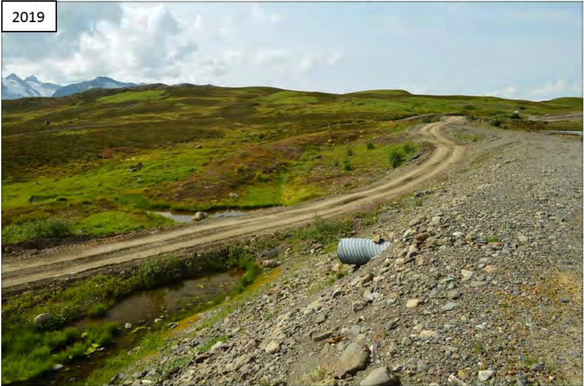
Photo I-25 Southwest Dam Downstream Slope and Access Road at Toe (SW-4)
