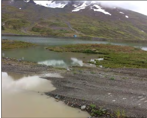
Photo 8-1: Vantage point photo of southeast corner of the Main Landfill looking east. Ponding water over low section of TSF where drainage from Main Landfill enters TSF.
