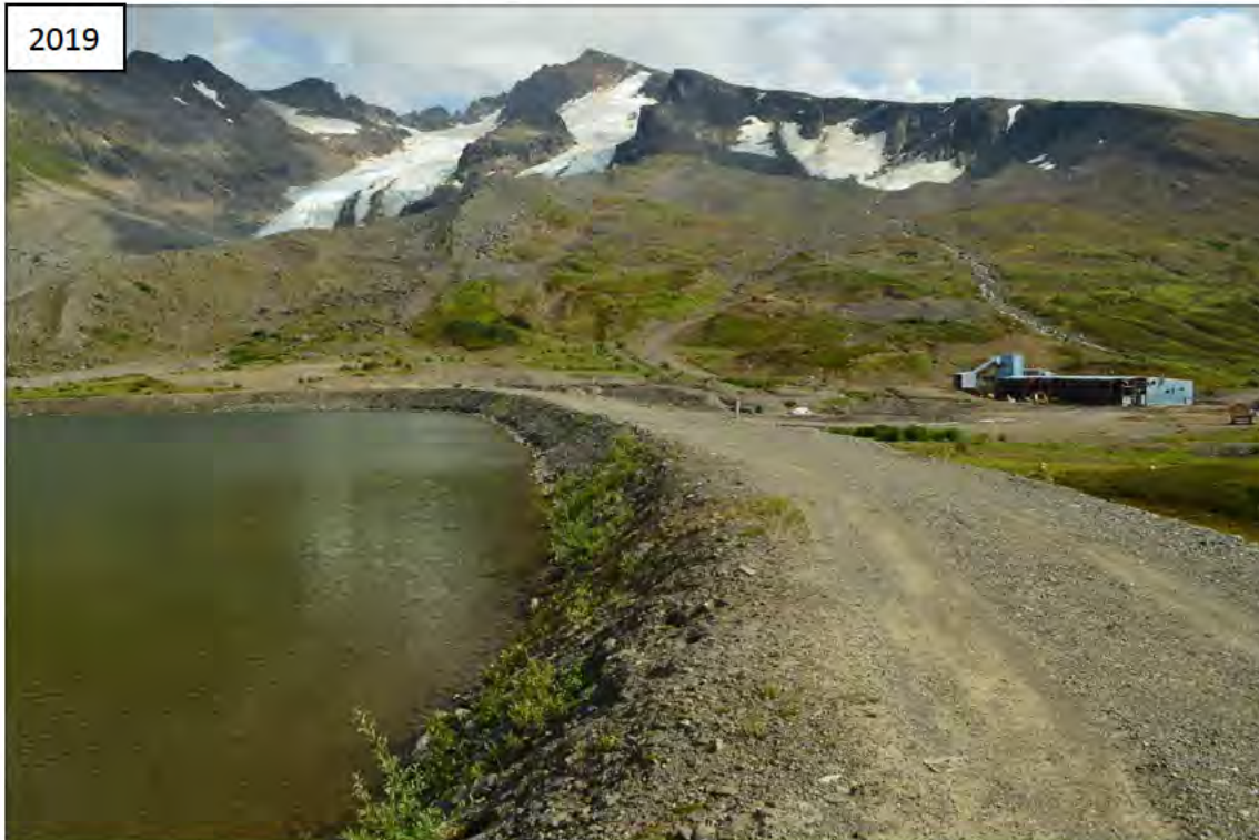
Photo I-23 Southwest Dam Crest Looking East (SW-2)
