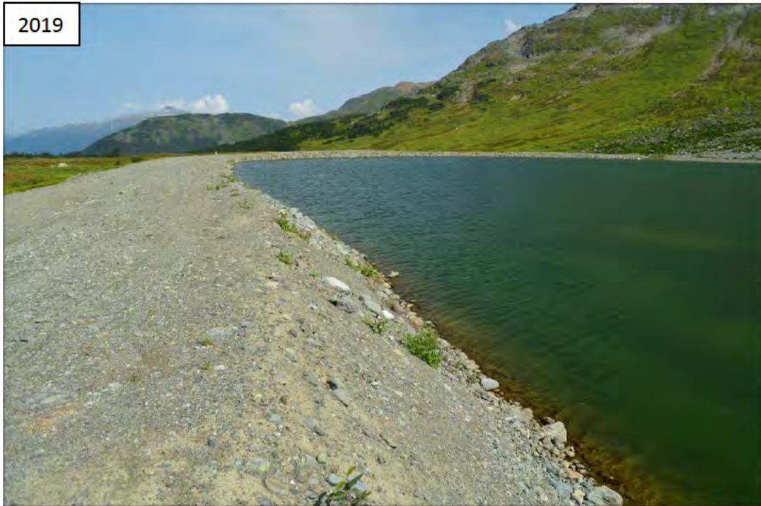
Photo I-6 Northwest Dam Upstream Face and Crest (NW-3)
