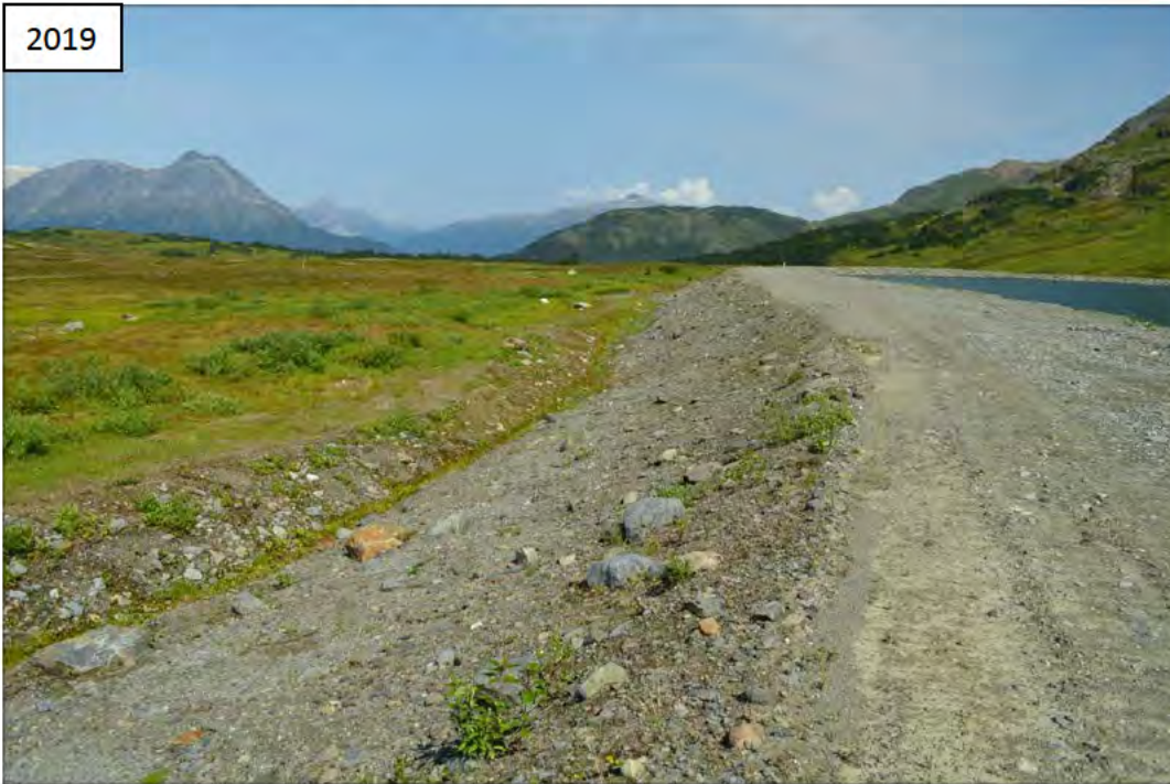
Photo I-3 Northwest Dam Downstream Face (NW-2)
