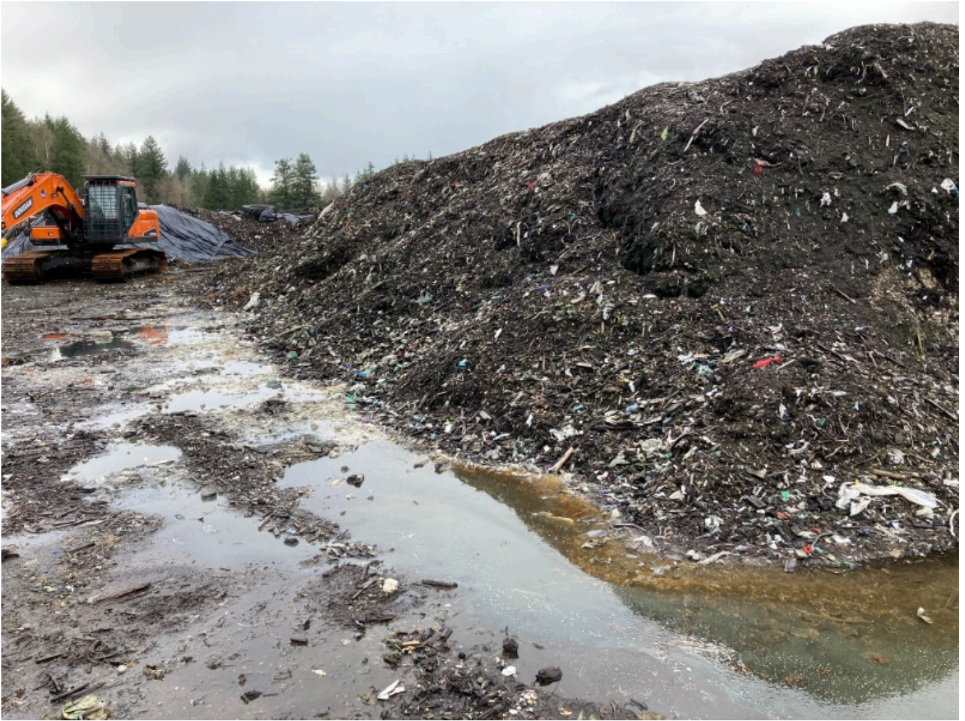
Photo 5: Viewing east towards leachate discharging to ground at the base of an unscreened pile of waste
