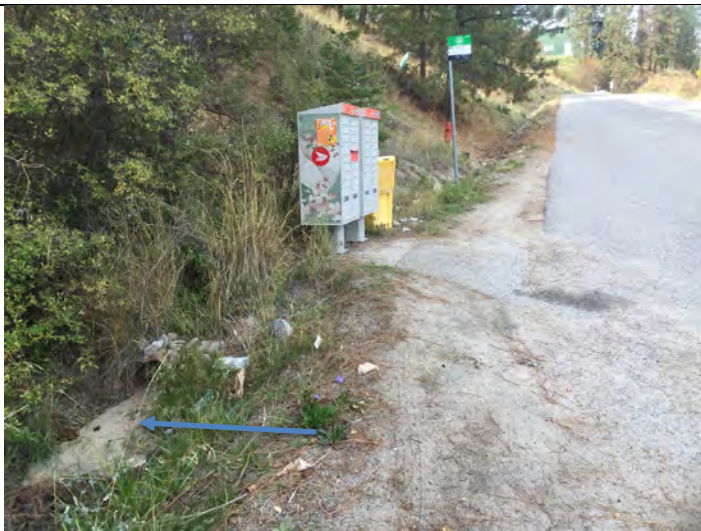
Photo 5: Shallow ditch along Bear Creek Rd (at McNaughton) with small culvert under mailbox. Note recent sediment in ditch (arrow) (Keefe-1)
