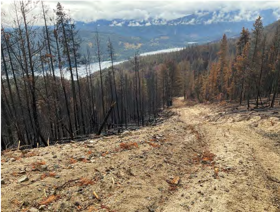
Photo 11. Firebreak road running straight downslope over moderate (30-50%) sloping terrain.
