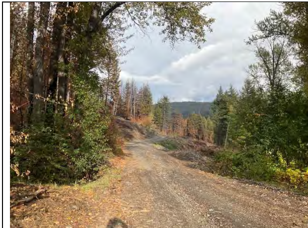
Photo 22. WP DK103. View campside past Penrose Creek crossing on Road R06128 28-713-220. Ensure culvert is clear and sag is maintained.
