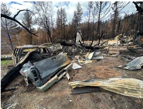
Photo 9. Burnt structure on 13770 Gun Ck Rd West, affected by fire tornado. Note thrown and snapped trees and thrown roofing metal.
