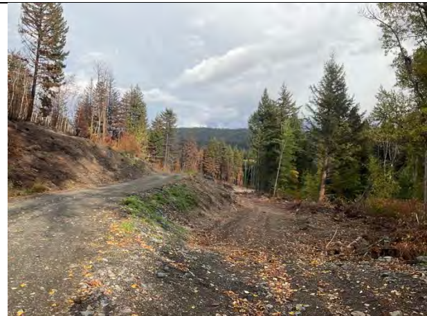
Photo 23. WP DK103. View campside past Penrose Creek crossing on Road R06128 28-713-220 to lower side of road where avulsion could impact.
