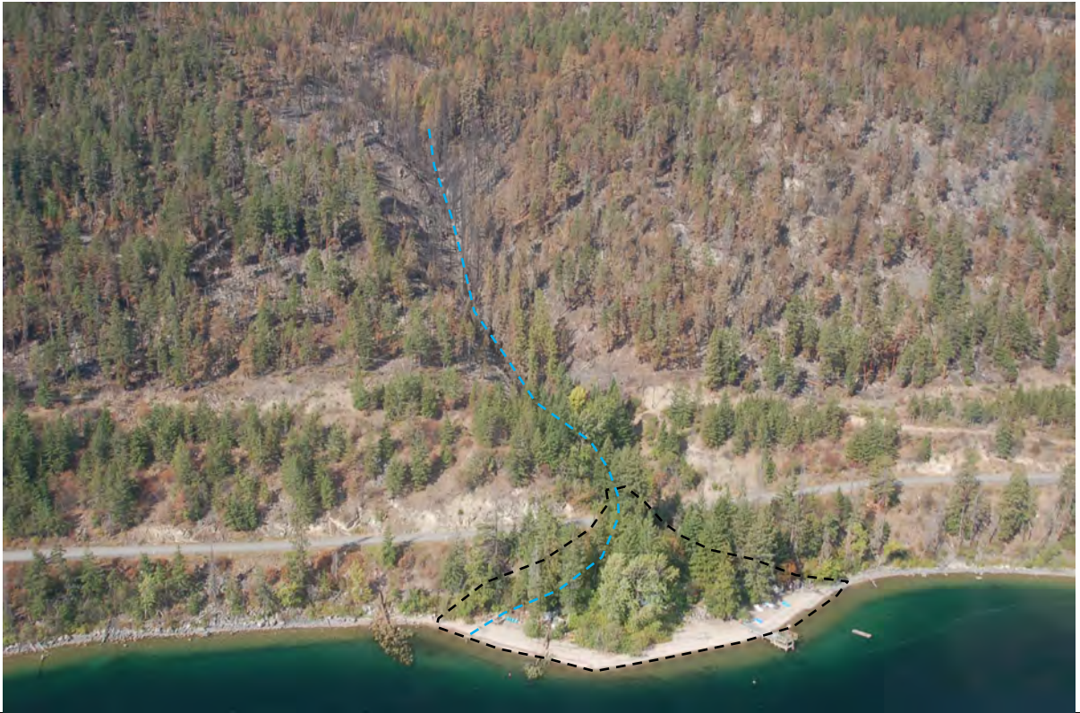
Photo 7: Lower Quilpituk Creek and fan area situated below Westside Road (outlined). Note the burned canyon slopes upslope of Westside Road. Note the private property on small fan below Westside Road.
