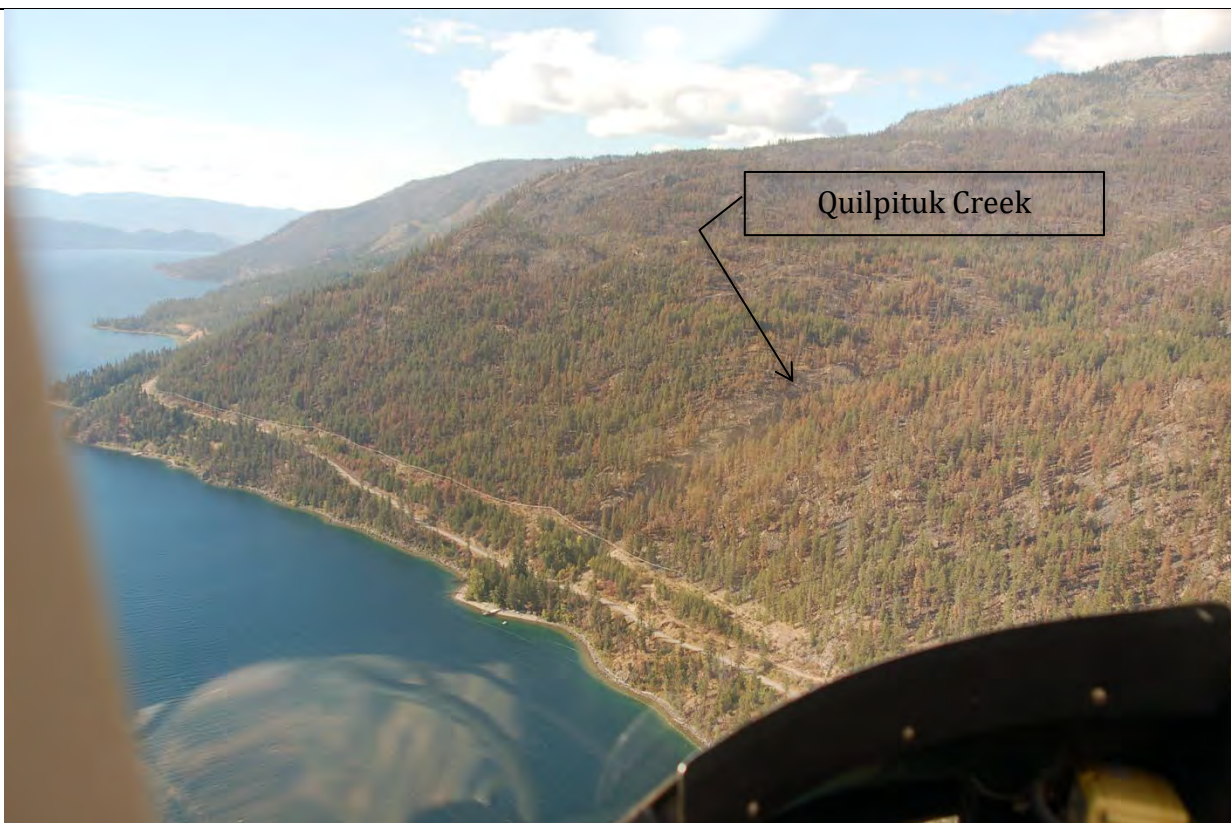
Photo 1: View (south) of Quilpituk Creek gully extending down to Westside Road and the small fan area on Okanagan Lake. Linear feature upslope of Westside Road is the Fortis power transmission line.
