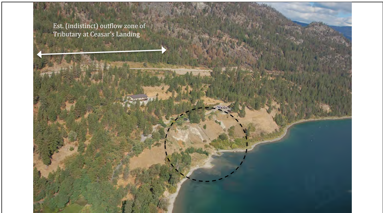
Photo 9: Private property downslope of Westside Road near undefined outlet of Tributary at Ceasar's Landing. There were no observed culverts along Westside Road at the mapped channel path. However, there are nearby culverts that could be receiving runoff from the upslope catchment. Note the large landslide slump features along the shoreline (circled).
