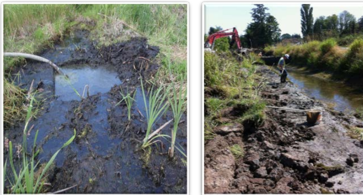
Figure 4. Sump creation and/or pump installation [left; photo credit N. Sands], and dipnetting during dewatering [right; photo credit S. Sloboda]
