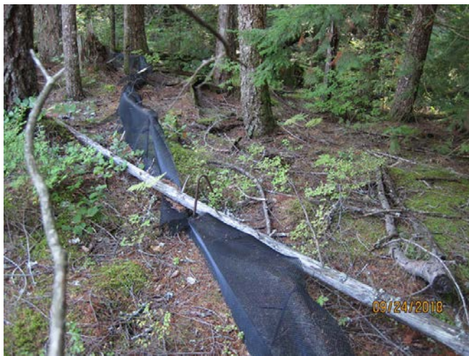
Photo 64. Maintenance monitoring is required to check for storm damage to fencing such as this fallen tree at Highway 99, Pinecrest. Photo credit: Barb Beasley.
