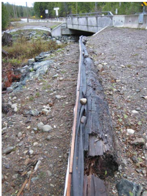
Photo 6. Bridge structure with connected guiding fences that guide animals around bridge abutments – Highway 4 Lost Shoe Bridge. Photo credit: Barb Beasley.
