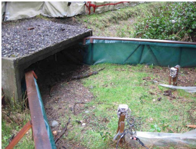
Photo 69. Digital camera mounted outside the entrances of crossing structure to monitor the effectiveness of the fences in leading amphibians into the tunnel at Highway 4 near Ucluelet. Photo credit: Barb Beasley.
