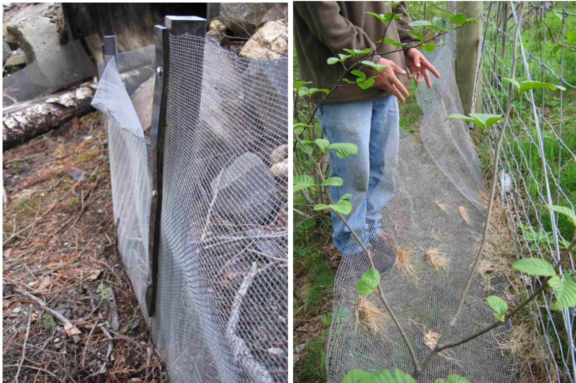
Photo 39. Hardware cloth torn off fence post 3 years after installation on Highway 99 at Pinecrest (left) and ungalvate fencing on Highway 19 near Courtenay (right). Photo credit: Barb Beasley.
