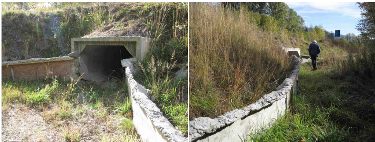
Photo 45. Concrete fencing guiding amphibians to tunnel under Highway 6, Summit Lake. Photo credit: Barb Beasley.
