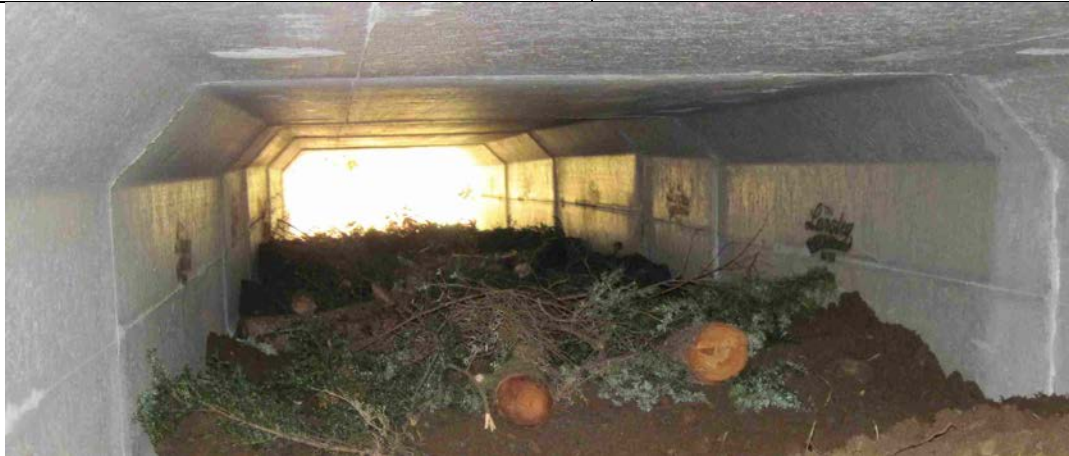
Photo 14. Soil and branches inside bottom of tunnel provide amphibians with moisture and places to hide from predators, Highway 4. Photo credit: Barb Beasley.
