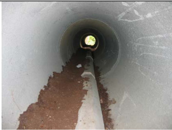
Photo 23. Round concrete tunnel with raised concrete strip and dirt to provide a bench for amphibians to use as water levels rise at Laburnum Road, Qualicum. Photo credit: Barb Beasley.
