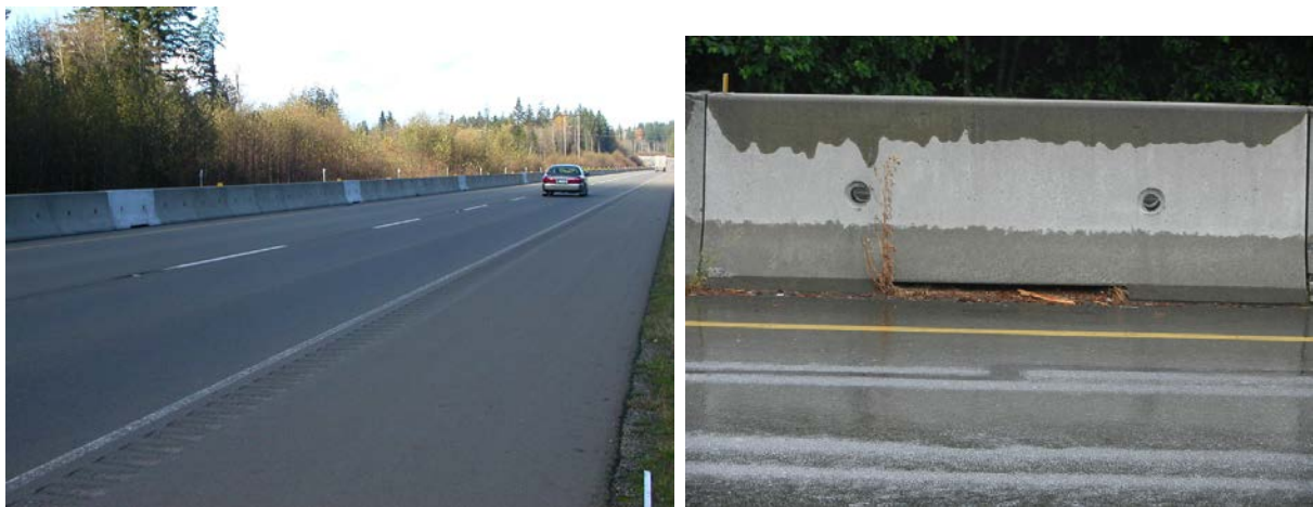
Photo 61. Scuppers under precast concrete barriers placed in the middle of a divided highway allow toadlets to escape the road. Photo credit: Elke Wind.
