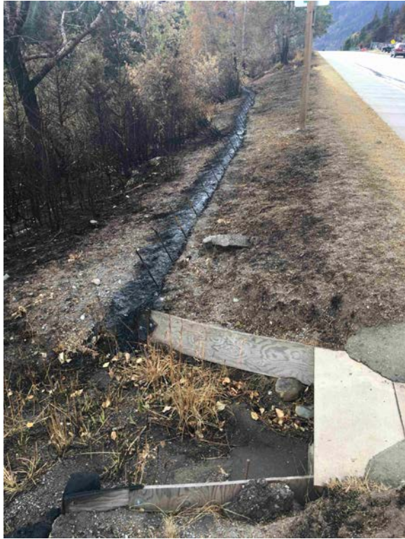
Photo 42. Waterton Lakes National Park's curved plastic fencing (sections of pipe) melted down after the 2017 fire. Photo credit: Kim Pearson, Parks Canada.
