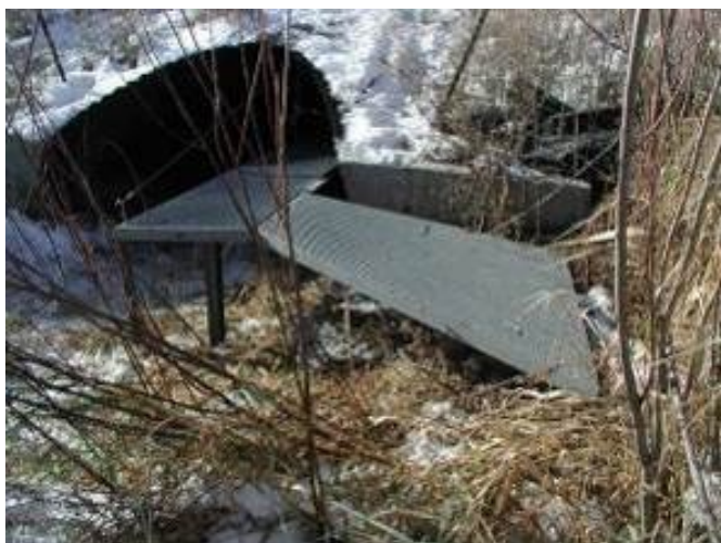
Photo 26. Existing culvert retrofitted with entryway ramp and inner shelf/bench. Photo credit: K. Foresman.
