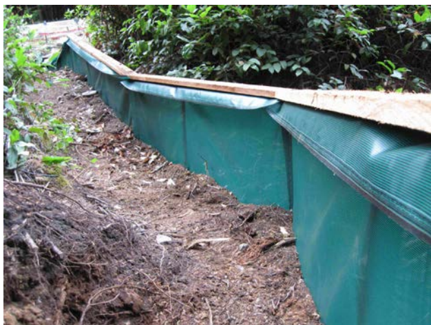
Photo 46. UV-resistant polypropylene fabric (pool cover fabric) installed with plastic wood posts and cedar rails over uneven terrain at Highway 4 near Ucluelet. Photo credit: Barb Beasley.
