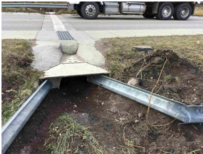
Photo 43. Metal curb sheeting used to replace plastic fence after it melted in the 2017 fire at Waterton Lakes National Park. Photo credit: Kim Pearson, Parks Canada.
