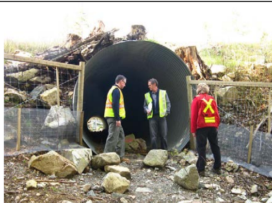
Photo 24. Very large corrugated metal culvert crossing Sea to Sky Highway at Pinecrest. Photo credit: Elke Wind.
