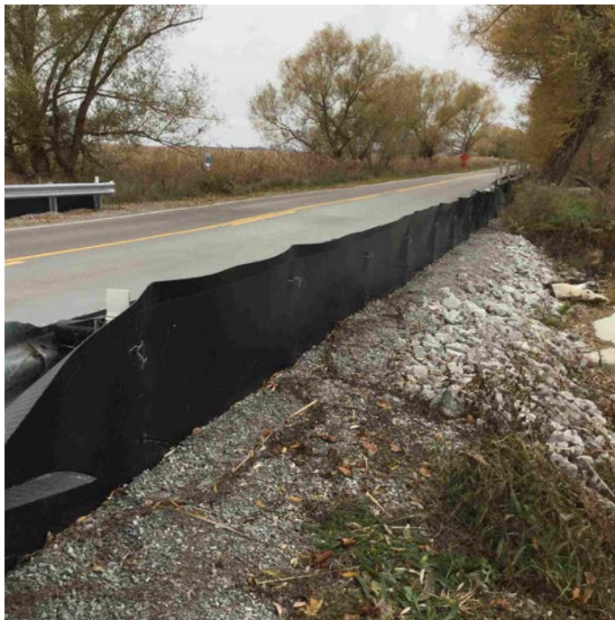
Photo 41. Animex UV-resistant HDPE straight-sided plastic with a scored top that can be bent over to form a top lip, Long Point Causeway, Ontario. Photo credit: Barb Beasley.
