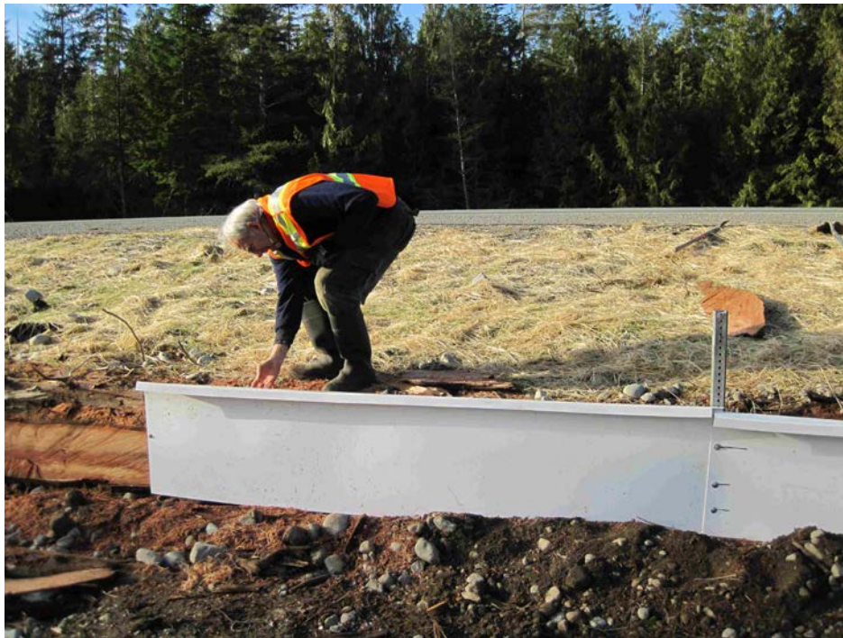
Photo 35. Rigid plastic fencing installed below road level along Highway 4, Vancouver Island. Photo credit: Barb Beasley.
