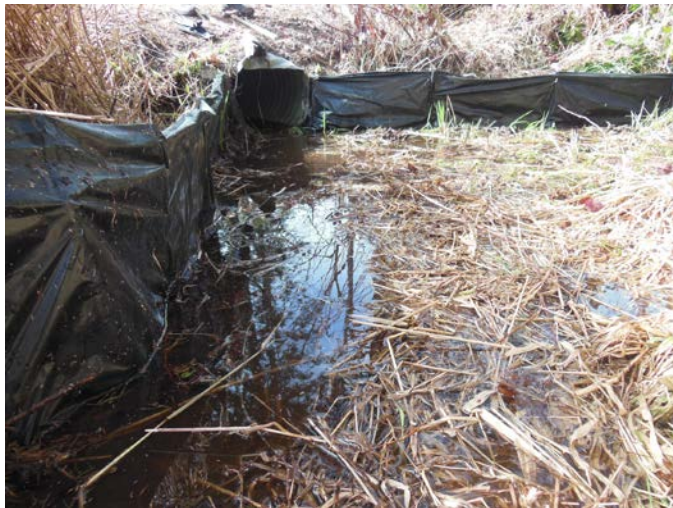
Photo 25. Existing culvert retrofitted with temporary directive fencing. Photo credit: Elke Wind.
