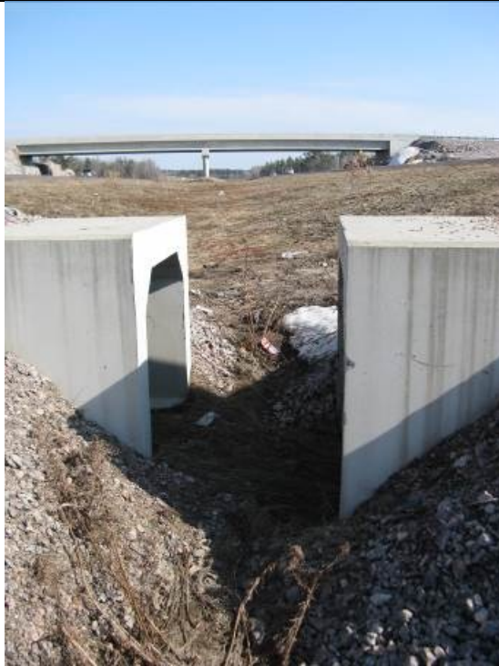
Photo 12. Box tunnels in the median that should be connected with a fence when intended for wildlife passage. Photo credit: K. Gunson.
