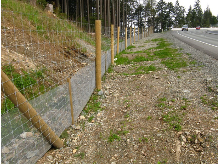
Photo 40. Amphibian and reptile fencing attached to the bottom of large animal chain link fencing. Photo credit: Elke Wind.
