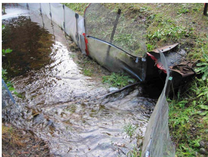
Photo 33. Temporary fencing used along Highway 4 near Ucluelet included mesh fencing to allow for drainage and a slippery plastic cover (not buried) to impede climbing by amphibians. Photo credit: Barb Beasley.
