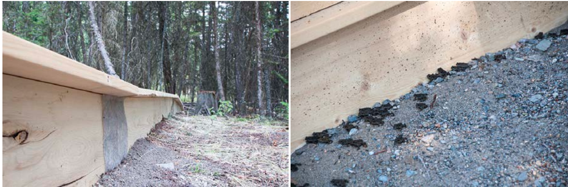
Photo 44. Wooden fencing installed at Kentucky-Alleyne Provincial Park to keep Western Toads off road. Photo credit: Kristiina Ovaska
