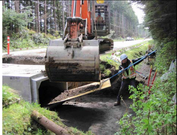
Photo 13. Filling sections of amphibian tunnel on Highway 4 with natural substrate during the installation. Photo credit: Barb Beasley.
