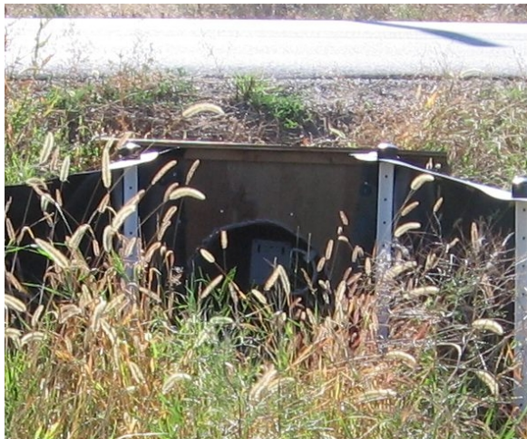
Photo 48. Pressure treated plywood was used to make a semi-permanent and low cost fitting for round and oval culverts to provide a firm and gapless attachment structure for direct fencing in a dry environment. Photo credit: Mike Sarell.
