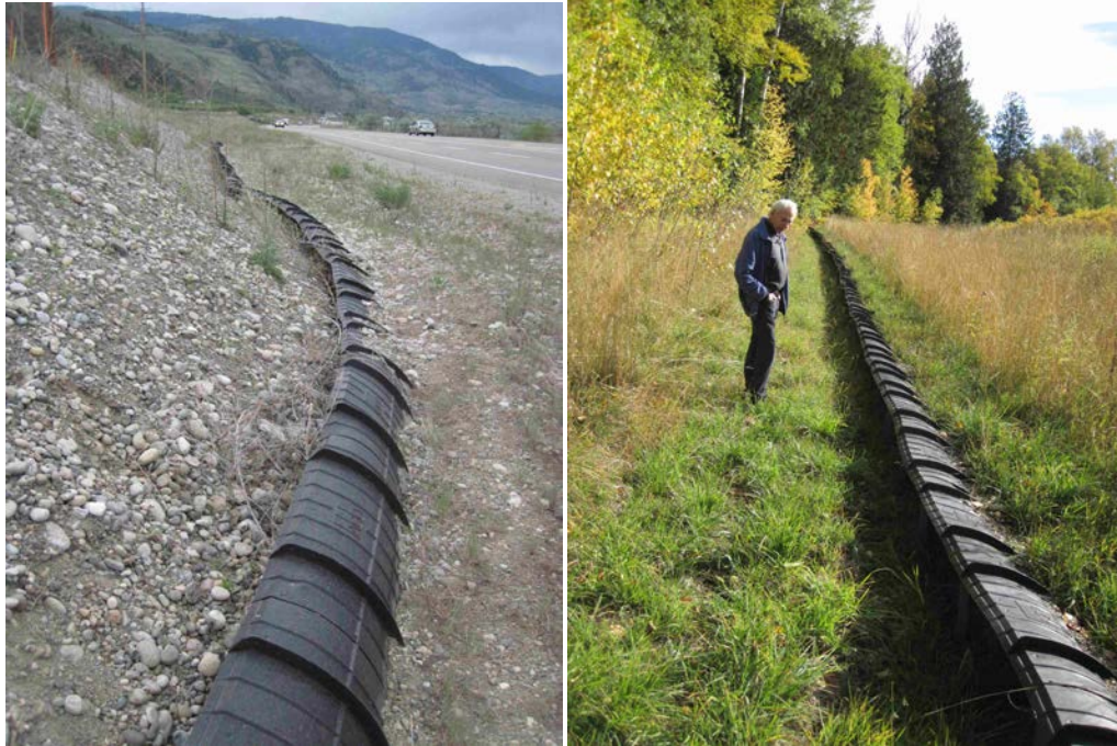
Photo 36. Curved backside of ACO fencing allows animals to climb over along its entire length at Highway 97 Osoyoos (left) and Highway 6 near Summit Lake (right). Photo credit: Barb Beasley.
