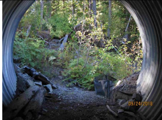
Photo 18. Water diverted down slope away from tunnel entrance at Highway 99 near Pinecrest, although too little water may make tunnels too dry for amphibians. Photo credit: Barb Beasley.
