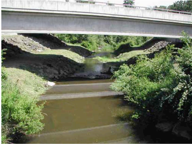
Photo 5. Bridge crossings need to be wide enough to allow dry passage for terrestrial animals along stream banks with vegetation to provide safety cover, Millstone River Bridge, Nanaimo. Photo credit: Richard Eliassen.
