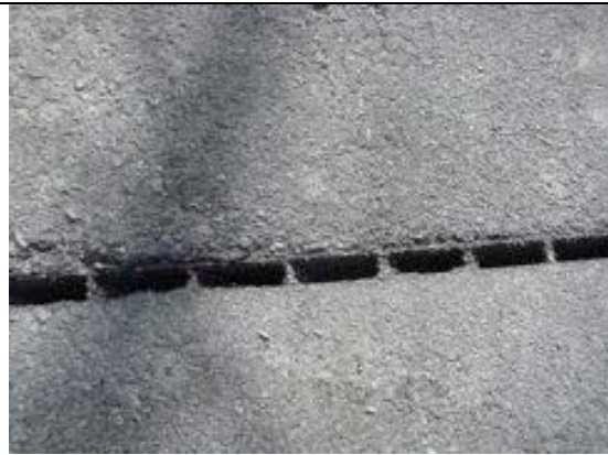
Photo 22. Zoom-in of open-top pipe culvert installed at road for Timber Rattlesnakes in Illinois, U.S. Photo credit: S. Ballard.
