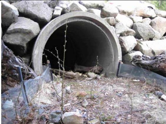
Photo 17. Round concrete tunnel partially filled with material so that the entrance is even with ground level, Laburnum Road in Qualicum. Photo credit: Barb Beasley.
