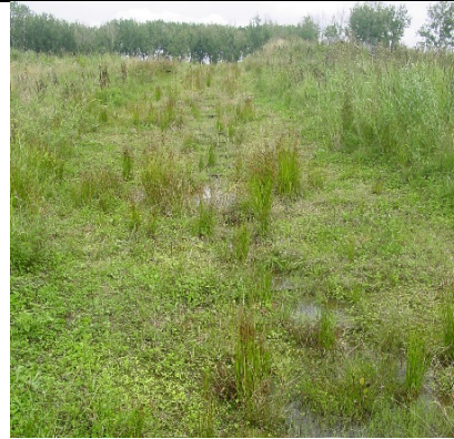
Photo 28. Wetland zone on wildlife overpass Groene Woud, consisting of a series of small ponds on loamy soils supplied by water pumped up to the top of the overpass. Photo credit: Rijkswaterstaat.
