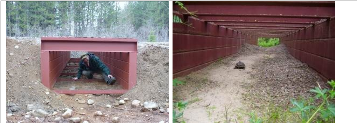
Photo 15. Sediment baffles hold natural substrate inside tunnels with water flow. Photo credit: B. Steinberg (left) and A. Mui (right).
