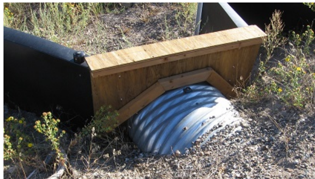
Photo 48. Pressure treated plywood was used to make a semi-permanent and low cost fitting for round and oval culverts to provide a firm and gapless attachment structure for direct fencing in a dry environment. Photo credit: Mike Sarell.
