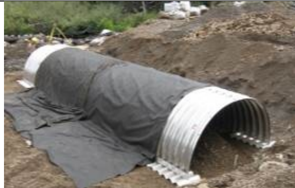
Photo 20. Aluminum arch culvert on metal footings. Photo credit: K. Williams.
