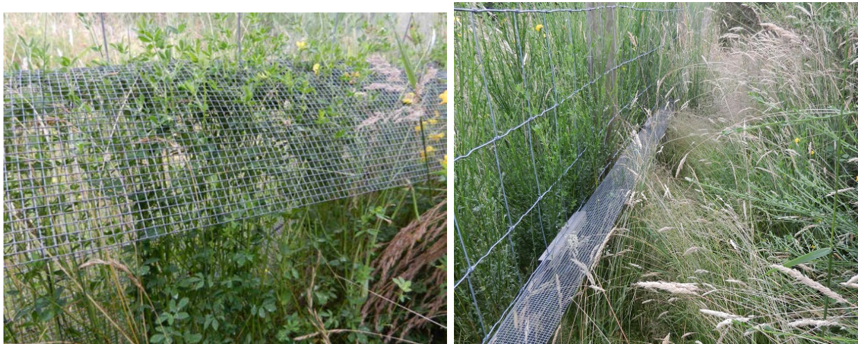
Photo 4. Vegetation along barrier and directive fencing needs to be carefully and regularly cleared to avoid having amphibians and reptiles climbing over it. Photo credit: Elke Wind.
