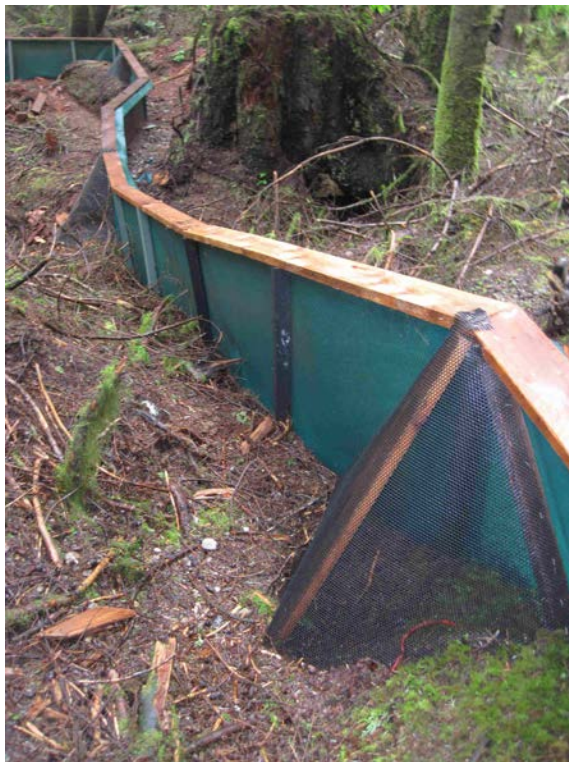
Photo 37. Mesh ramp on back/road side of exclusion fencing along Highway 4 near Ucluelet allows amphibians and other small animals caught on the road to escape. Photo credit: Barb Beasley.
