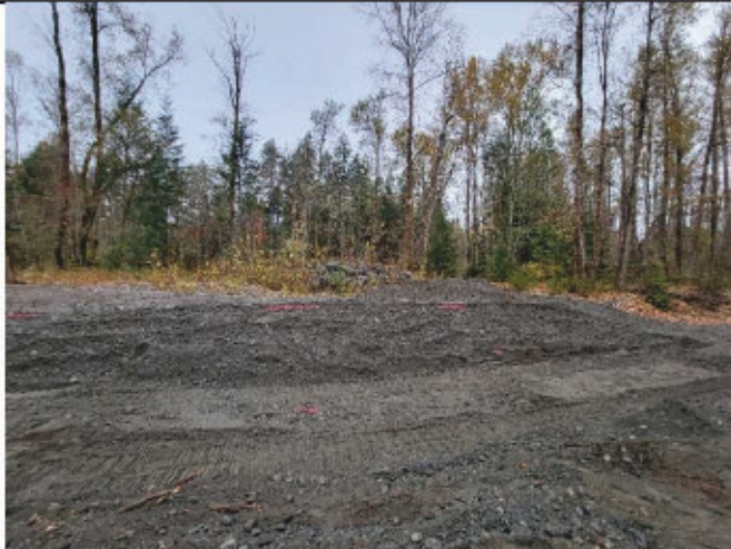
Photo 1: Area in front of downstream well head that will require riprap
