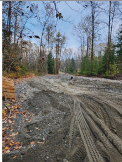
Photo 2: End of day progress looking downstream.
