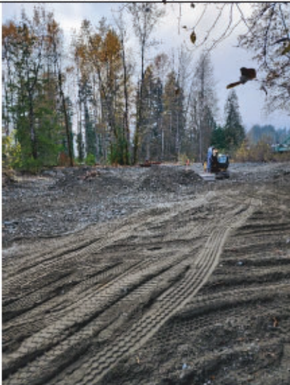
Photo 3: Remainder of bulk removal at end of day.
