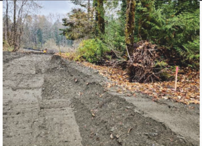
Photo 4: Looking downstream, right channel extents may impact tree nearest to top of bank.
