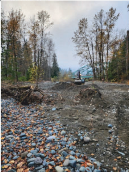
Photo 1: End of day, excavation remaining
