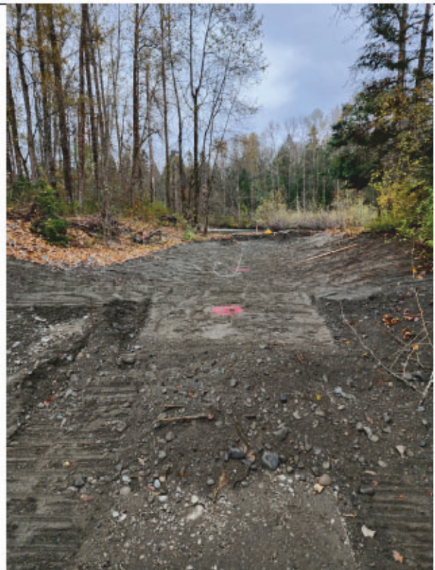
Photo 6: End of day progress downstream.
