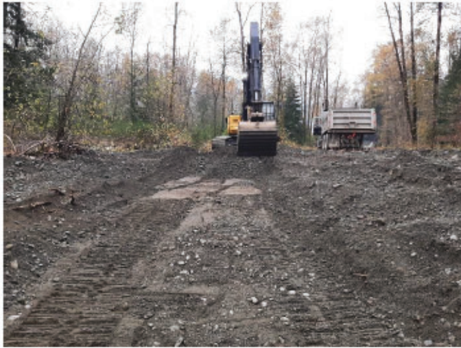
Photo 4: A dump truck being loaded by an excavator on accreted sediments of the historic side channel on Nov. 9, 2022.
