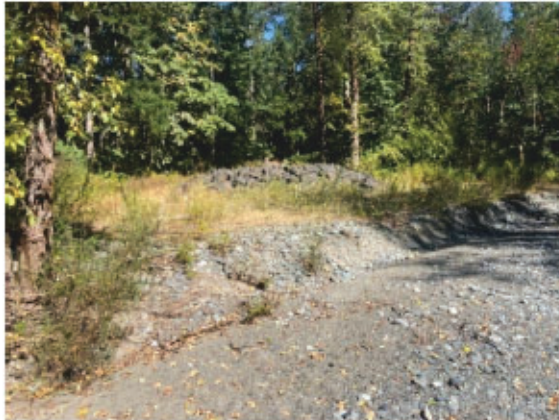
Photo 1: DNC Water Supply Well Head Protected by Riprap Adjacent to Side Channel
