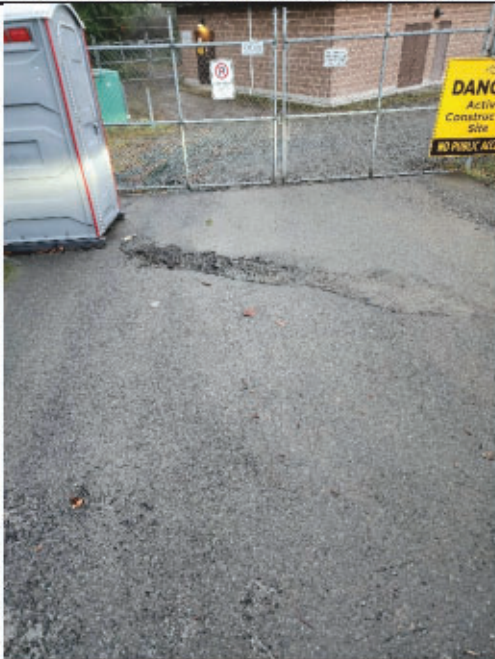
Photo 3: Asphalt drainage curb after demob.
