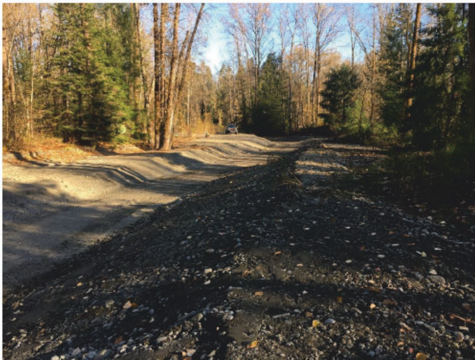
Photo 10: Walls of newly excavated left bank side channel after compaction with excavators.
