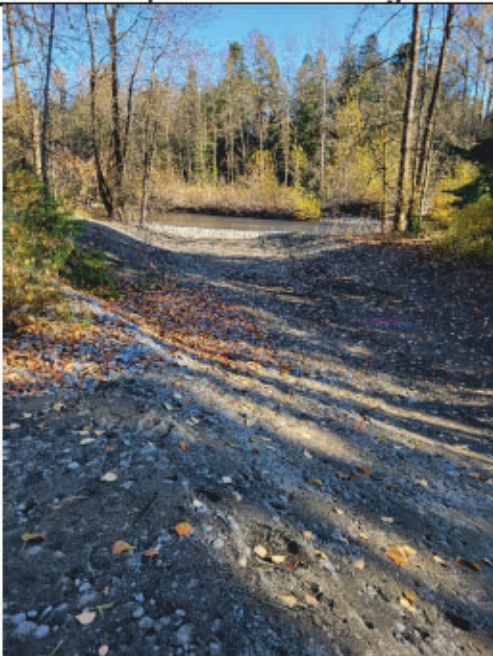
Photo 3: Downstream fill berm removed
