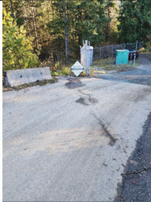
Photo 2: Drainage curb from another angle.
