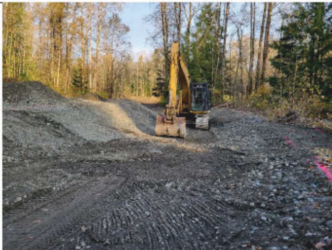
Photo 3: End of day progress at downstream end, looking downstream
