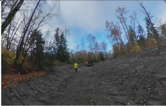
Photo 3: Grading continued towards upstream end.
