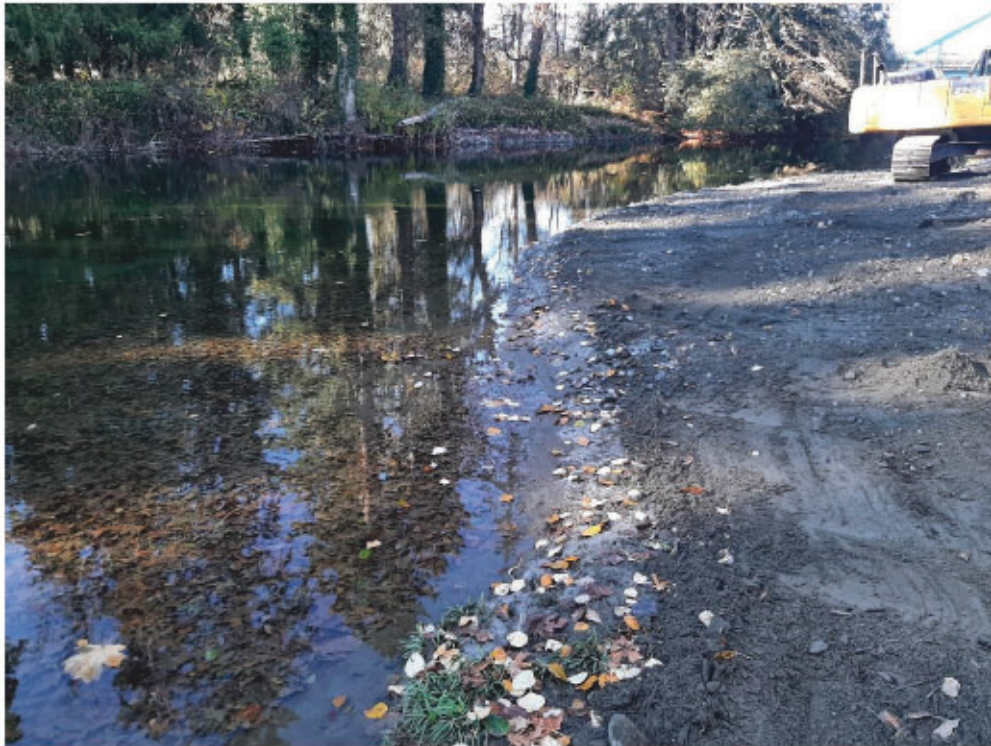
Photo 11: Point bar after bulk excavation was complete, while shaping and compacting was ongoing. No sediments were introduced to the river, and turbidity levels remained well within acceptable ranges.
