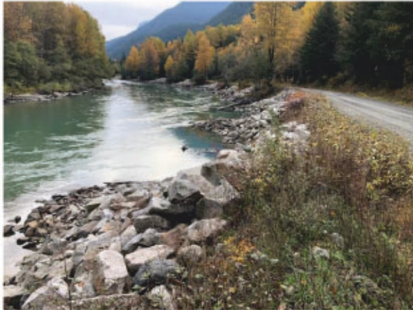
Photo 15: Example of Combination of Riparian Habitat with Rock Hard Points for Erosion
