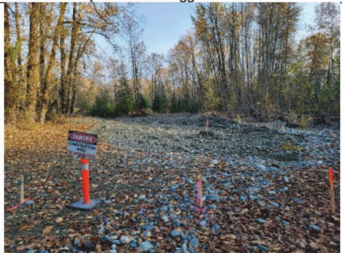
Photo 4: End of day progress at upstream end, some excavation remains at the access road
