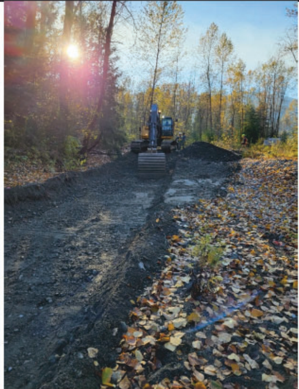
Photo 2: Overflow channel excavation beginning
