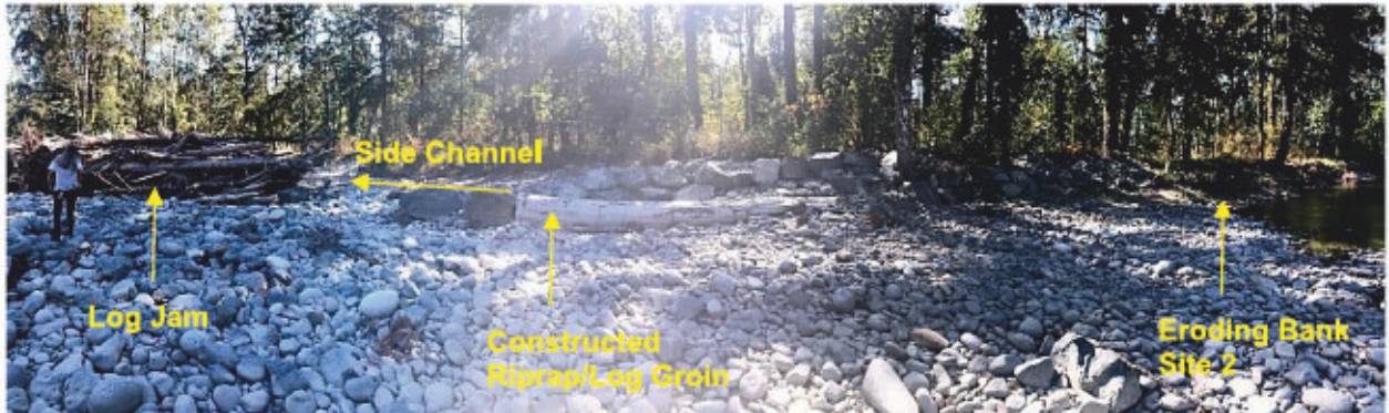
Photo 7: Entrance to Right Bank Side Channel Showing Eroding Bank, Riprap/Log Groin, Log Jam
