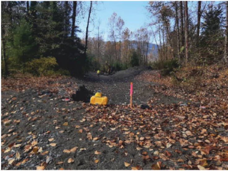
Photos 8 and 9: Sediment berms at the downstream (left) and upstream (right) end of the side channel excavation.
