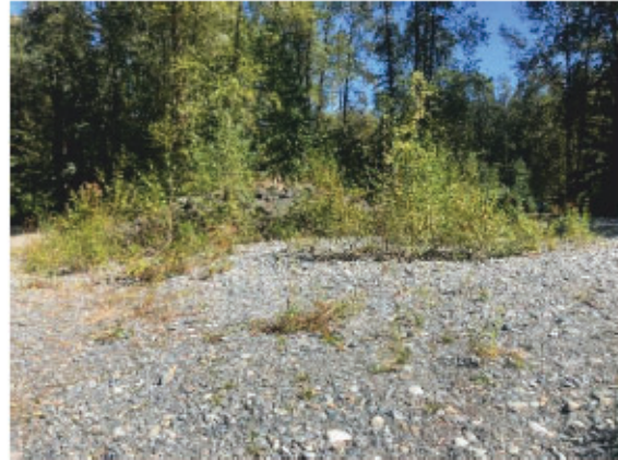
Photo 2: DNC Water Supply Well Head Protected by Riprap Adjacent to Side Channel
