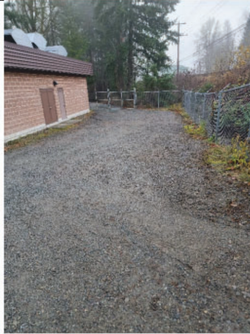
Photo 2: Pump house lot after demob.
