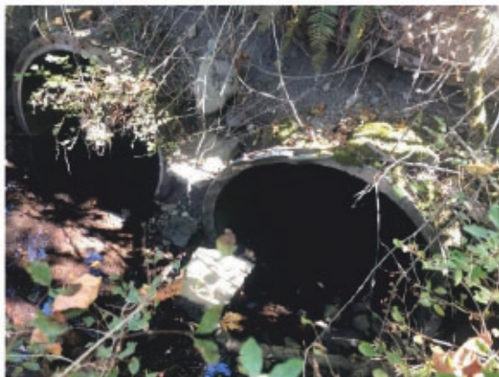
Photo 13: Swallowfield Access Road Culverts
