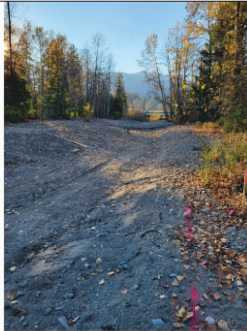
Photo 2: Channel excavation complete
