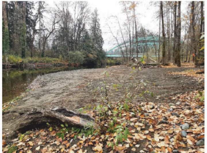
Photos 2 and 3: Looking upstream at the point bar of Site 1 before (left) and after (right) removal. The point bar lies at the inside of a sharp bend in the river and forces flow towards the opposite bank and causing erosion during high flows.
