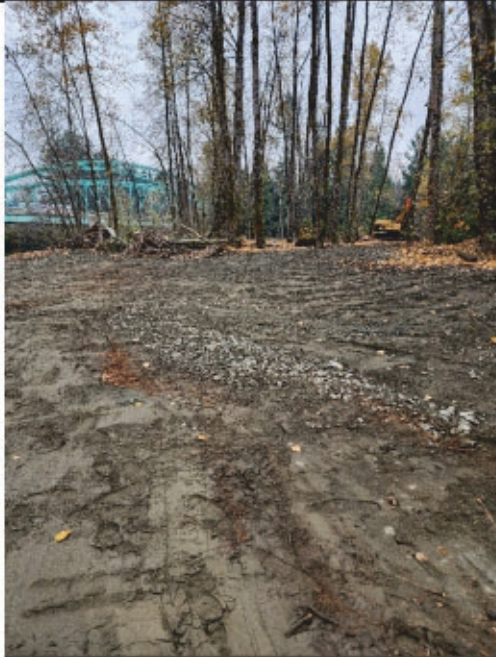
Photo 3: Point bar at completion mid-day.
