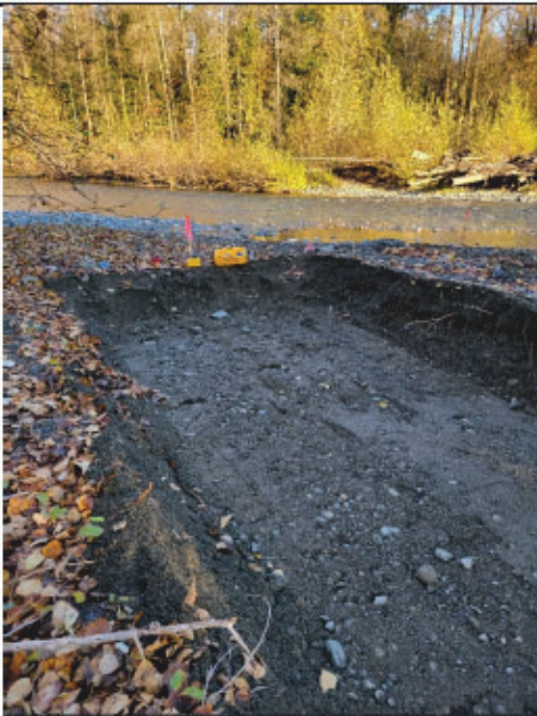
Photo 3: Unexcavated "berm" at downstream end of channel.
