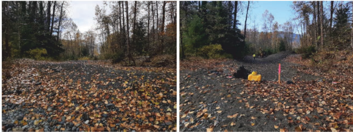
Before and during photos of the downstream end of the left bank side channel excavation.
