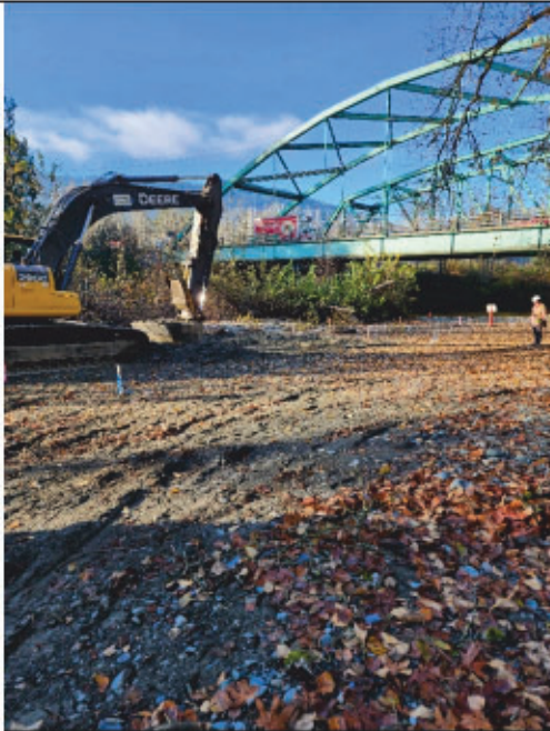
Photo 1: Excavation starting at upstream end.
