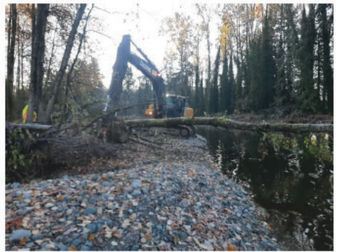
Photo 5: Excavator removing downed cottonwood from the mainstem channel immediately upstream of the point bar.
