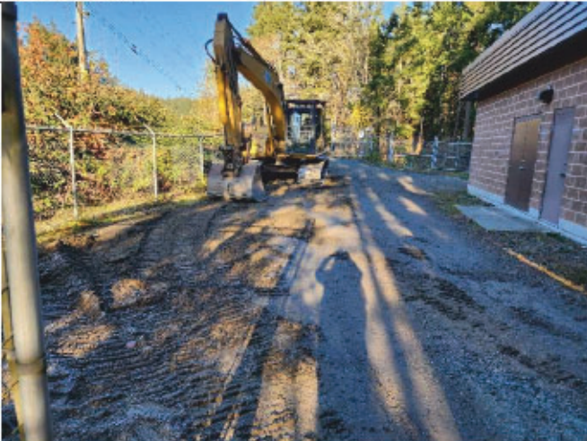
Photo 3: Stone Pacific to tidy pump house lot during demob.
