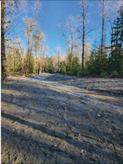
Photo 5: End of day, construction wrapped up.
