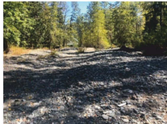
Photo 4: Sediment Accumulated Inside Channel on Right Bank of Chemainus River Note TCH Bridge in background
