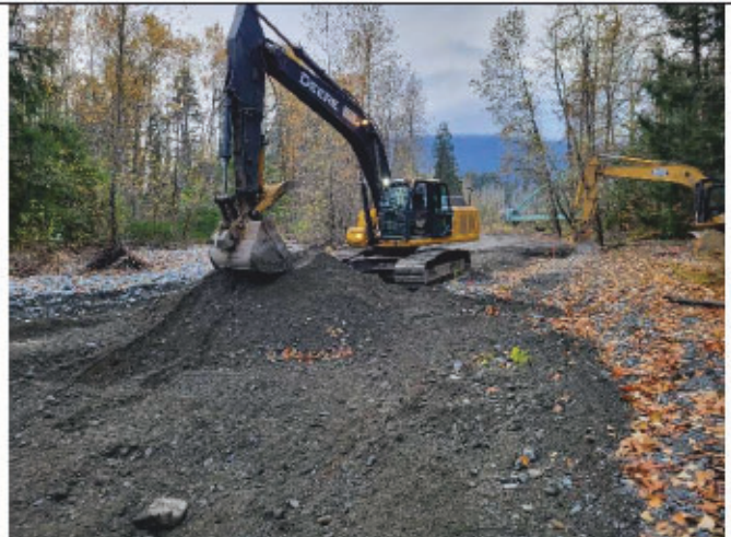
Photo 4: End of day progress – excavation has nearly reach the access road
