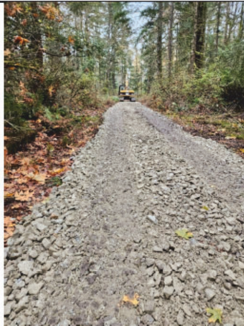
Photo 2: Material trucked in for access road.
