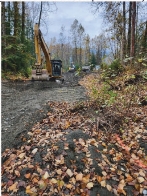
Photo 5: Looking upstream, one operator performing bulk material removal while grading commences at the downstream wedge.
