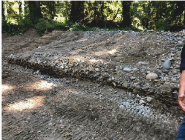
Photo 8: Opening Through the Berm for Smaller Right Bank Side Channel
