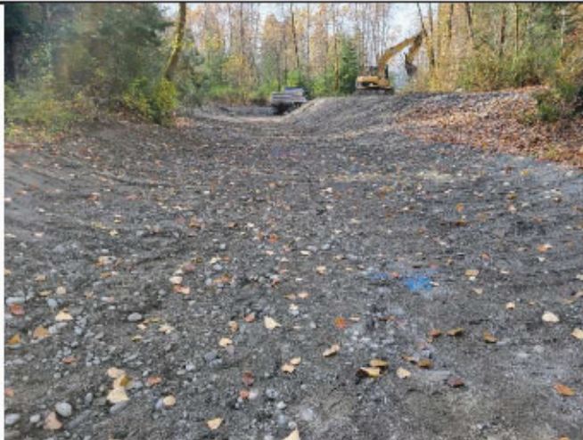
Photo 1: Initial shaping of 3:1 side slopes at the downstream end
