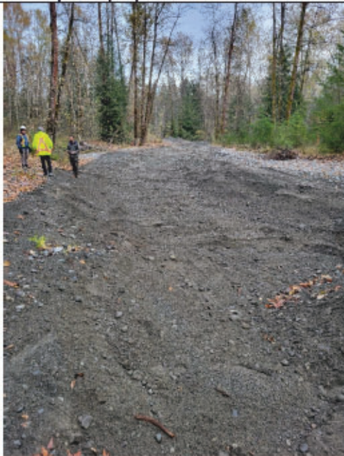
Photo 3: End of day channel extents, looking downstream
