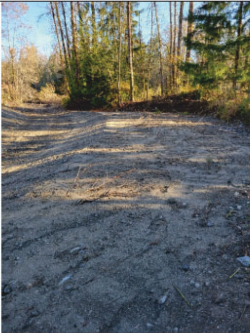
Photo 1: Overbank on right bank near downstream end filled to prevent fish stranding
