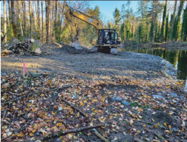
Photo 1: Bar topping nearing completion with removed tree
