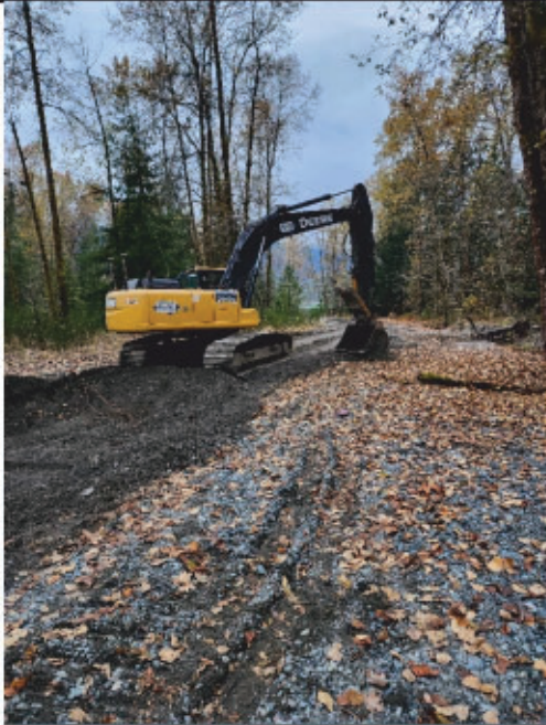
Photo 7: Looking upstream, end of day progress.
