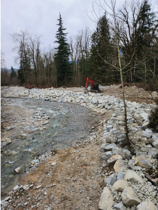
PHOTO #3 – Channel widened below bridge and rip rap armored
