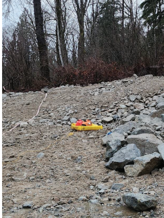
PHOTO #4 – Fuel and generator sitting in spill tray adjacent to wetted diversion channel
