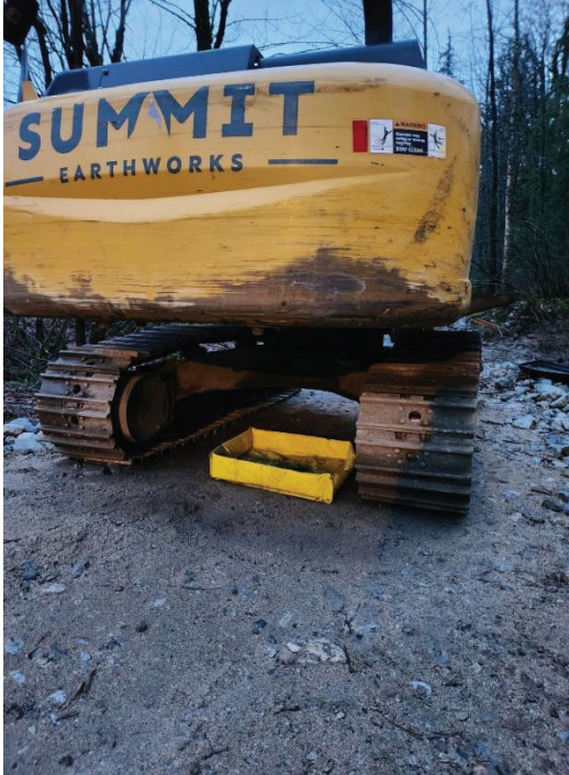
PHOTO #1 – Spill trays in use onsite
