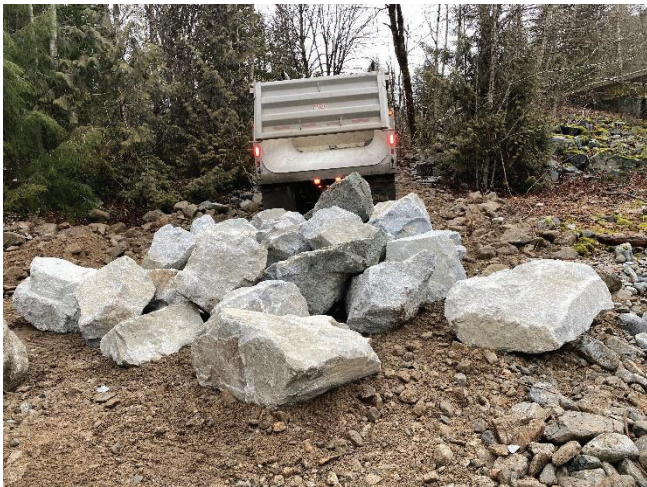
Figure - Looking northerly at 00kg being delivered
