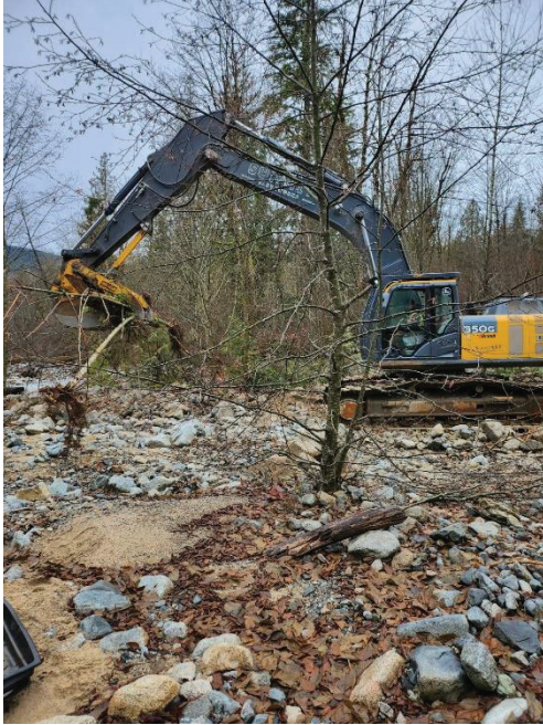
PHOTO #3 – Boney material used to armor eroded root mass
