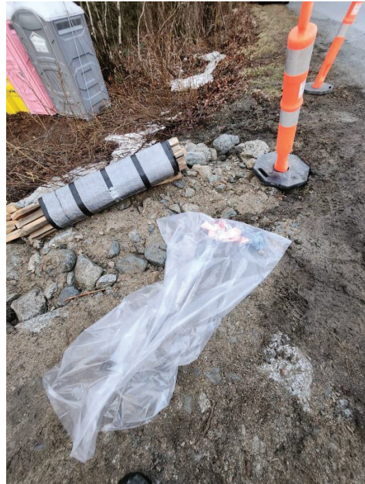
PHOTO #4 – Silt fencing onsite and trash bag in use for refuse
