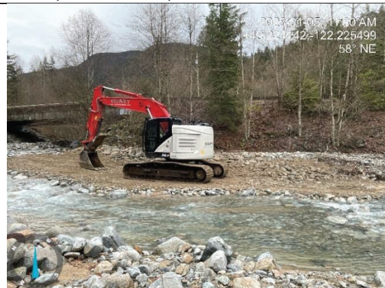
Photo 4. Grading and start of embankment stabilization. (Jan. 5, 2023).
