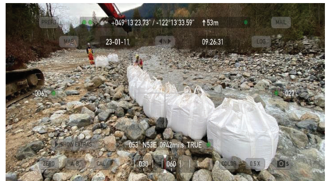
Figure -2 Looking northerly at meg bags in place
