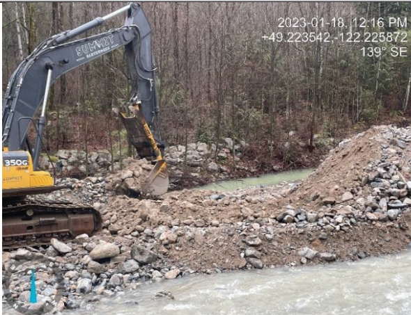
Photo 11. Backfilling at the head of the old creek channel (Jan 18, 2023).
