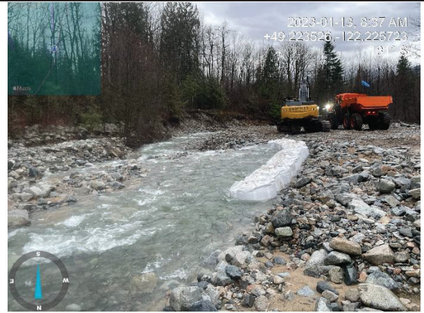
Photo 10. Downstream facing view of the deflection berm gravel bags in river-right margins of Pattison creek (Jan. 13, 2023).
