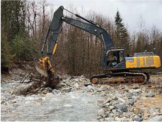
Figure - Looking southerly at debris removal at 0 100
