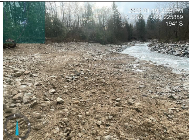
Photo 20. East embankment stabilized (Jan 19, 2023)
