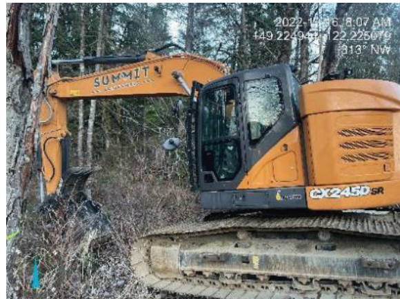
Photo 4. View of tree clearing for access road clearing (Dec. 16, 2022).
