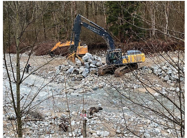
Figure -2 Looking westerly at the building of rock bridge
