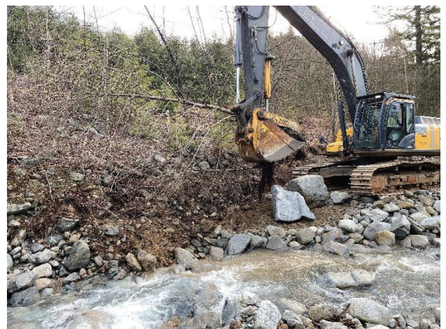
Figure -4 Looking at tree removal
