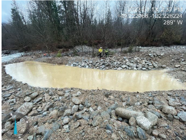
Photo 17. Turbid water within the excavated diversion channel was contained and left to settle over the weekend. (Jan 13, 2023).
