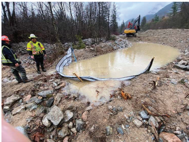
Figure -11 Looking northerly at installed settlement fencing
