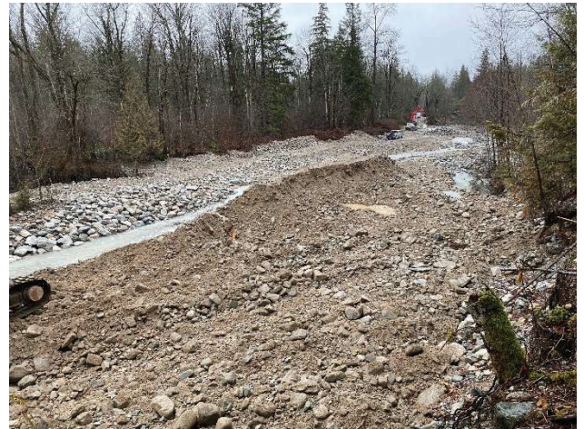
Figure -4 Looking northerly at infill at 50% complete
