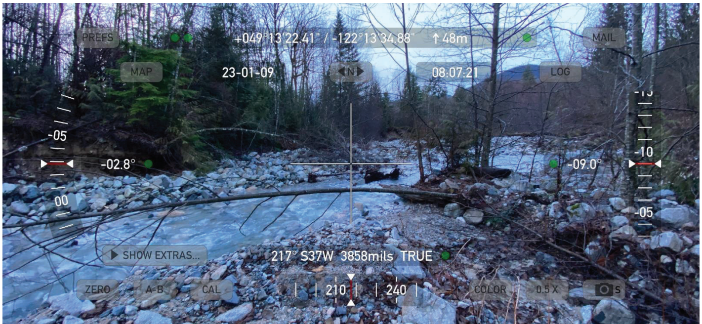
Figure - Looking at 0 200 before tree removal at creek edge
