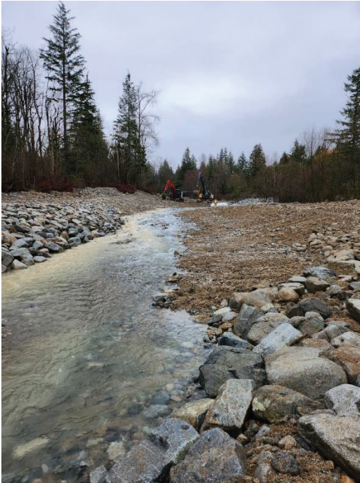
PHOTO #3 – Pulse of turbid water during channel widening and sand bag removal
