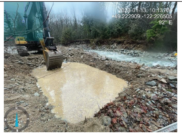
Photo 12. Pic of the excavation for the creek diversion channel. Turbid water was allowed to settle and has not yet been released from containment (Jan 13, 2023).
