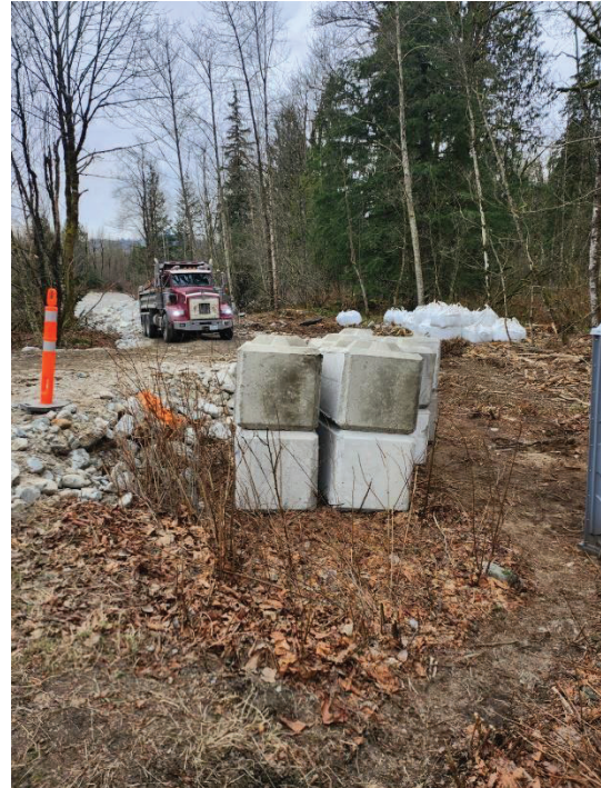
PHOTO #4 – Sang bags stockpiled for removal; lockblocks onsite ready for placement
