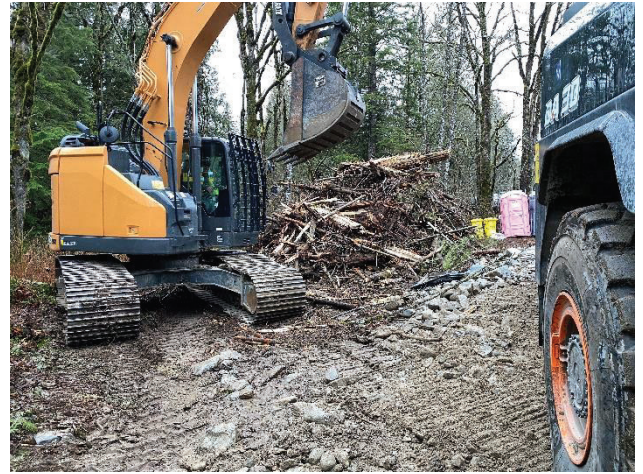
Figure - Looking at wood stockpile
