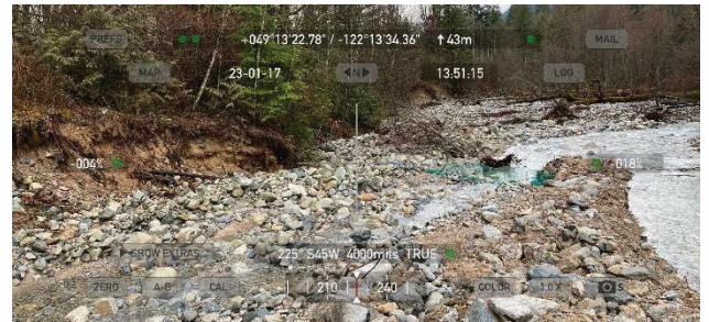
Figure -4 Looking southerly at downstream section creek - infill section -east bank
