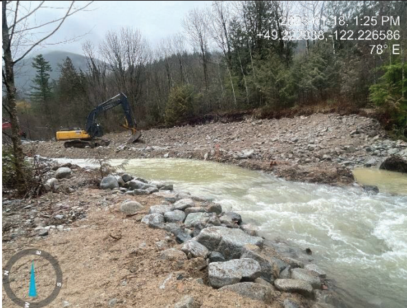
Photo 15. Grading of streambanks outside of the wetted stream perimeter and armoring with coarse material. Note that background flows were elevated, however, the EM observed the origin of the sediment to be upstream of the site (Jan. 18, 2023).
