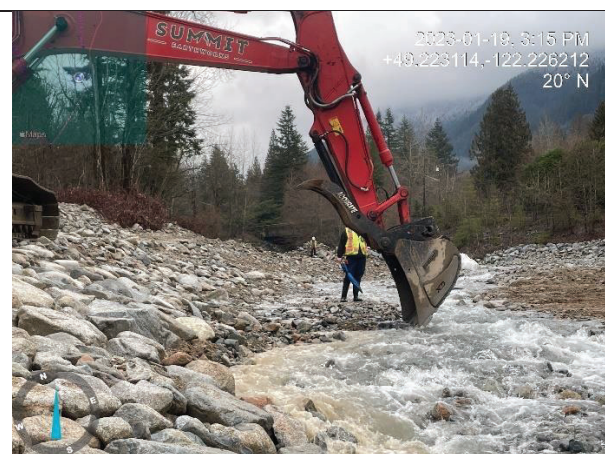
Photo 22. Sediment deposit removal from creek causing high turbidity monitoring (Jan 19, 2023).
