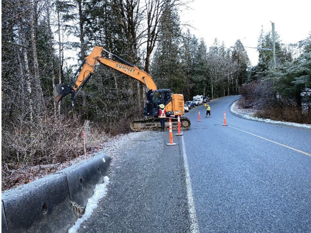
Figure -1 Looking northerly at the start of the clearing
