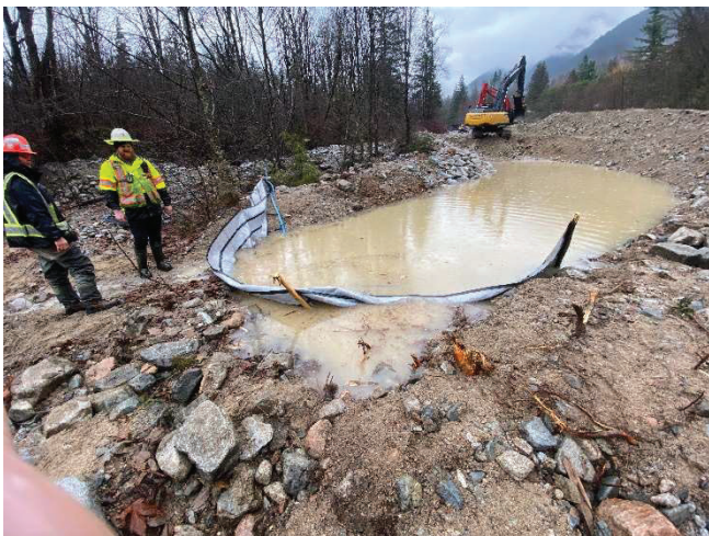
Figure -11 Looking northerly at installed settlement fencing
