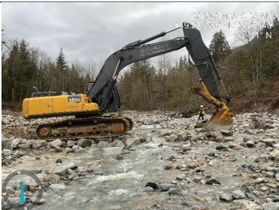
Photo 5. Creek crossing to access embankment stabilization works (Jan 6, 2023).
