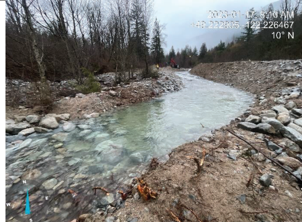
Photo 8. 75% of available flow diverted to the diversion channel (Jan 17, 2023)
