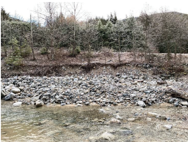
Figure - Looking easterly at the December 1 th before construction
