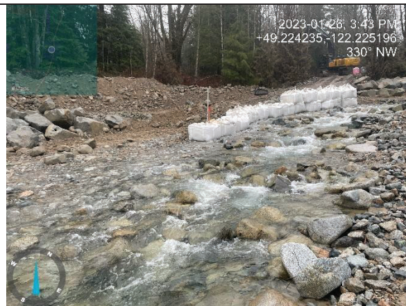
Photo 10. Northwest-facing view of ~25% flow in river right diversion channel. Deflection berm gravel bags being removed upstream. Salvage started in the afternoon. (Jan 26, 2023).
