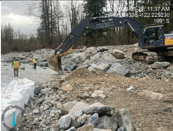
Photo 12. South-facing view prior to excavation beside last deflection gravel berm bags river right (Jan. 27, 2023).
