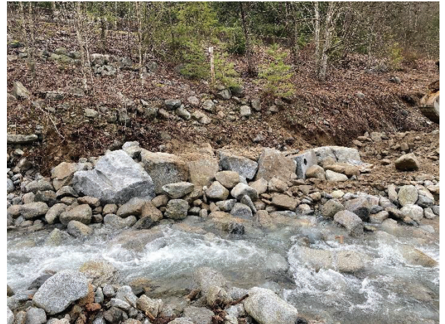
Figure - Looking westerly at first pieces of rip rap placed
