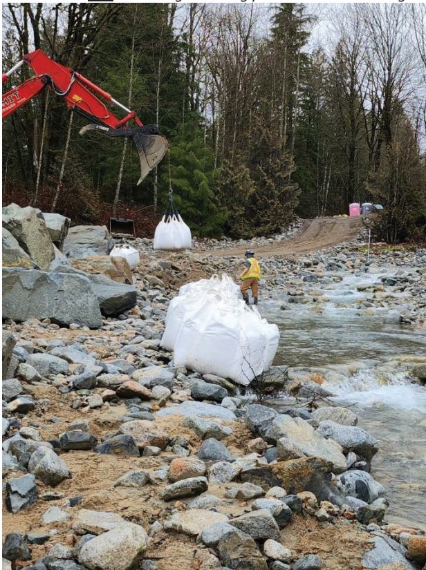
PHOTO #3 – 245 extending sand bag placement below bridge
