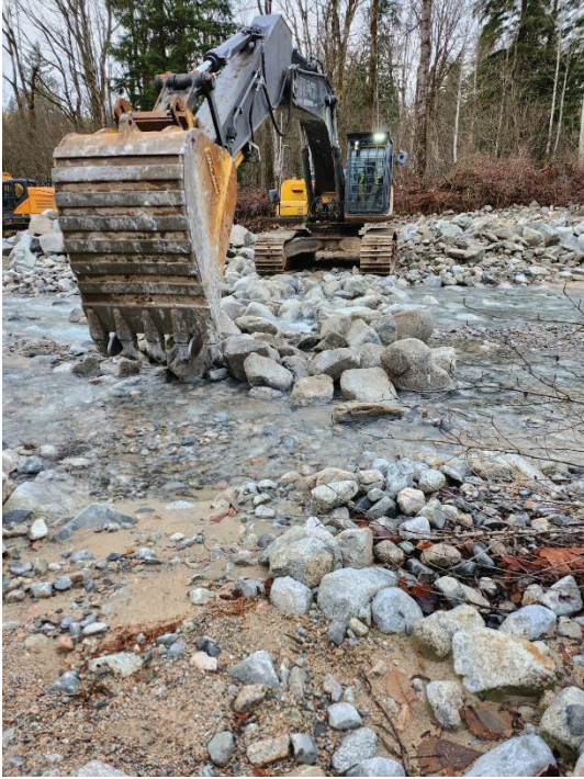
PHOTO #3 – Rip rap armouring installation along top of east bank
