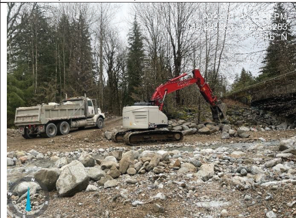
Photo 7. North-facing view downstream of the bridge of riprap placement along right bank (Jan. 25, 2023).
