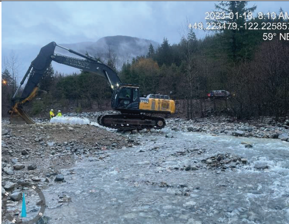
Photo 9. Excacator crossing to work on backfilling the old creek channel and bank stabilizing on the East side (Jan 18, 2023).
