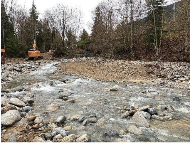
Figure -3 Looking northerly at the cleaned east bank at 0 020 to 0 040
