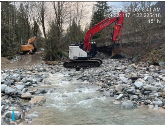
Photo 3. Creek crossing for grading and starting embankment stabilization works. (Jan. 5, 2023).
