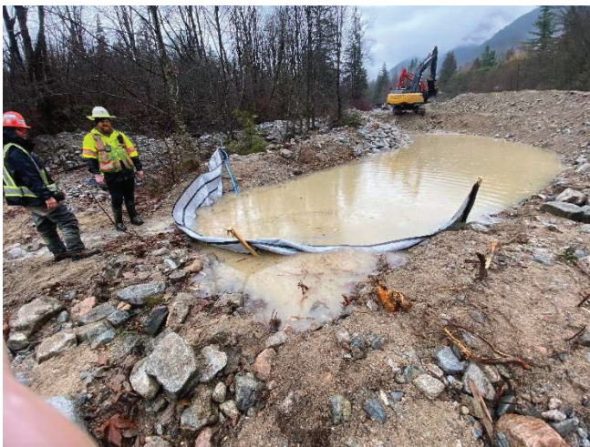
Figure -11 Looking northerly at installed settlement fencing
