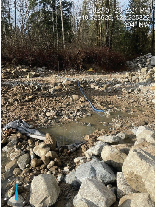
Photo 28. Set up sediment fencing to slow and settle the turbid flow (Jan 20, 2023).
