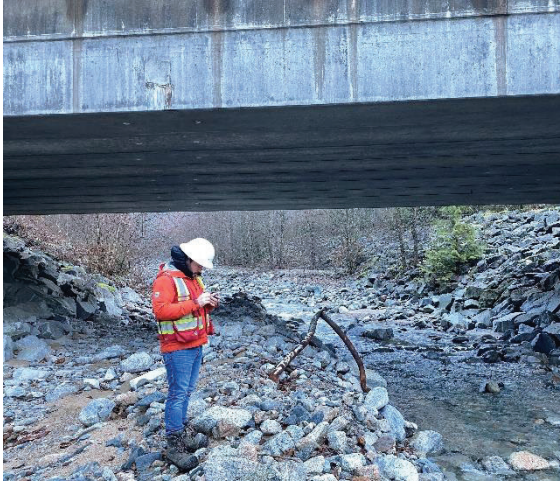
Figure 1 Looking upstream/easterly from west side of bridge-Sartori rep
