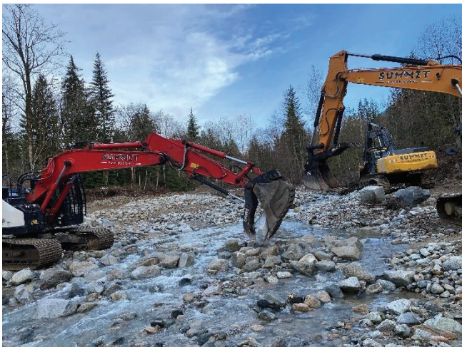
Figure -3 Looking northerly at passing of rip-rap across the creek
