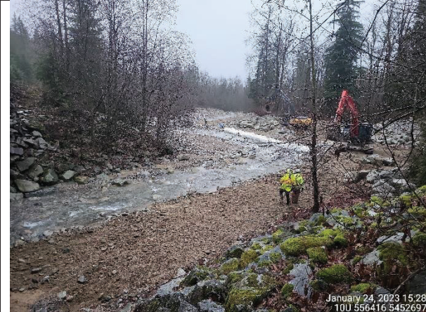
Photo 5. South-facing view of excavation downstream of the bridge to widen the creek channel (Jan 24, 2023)
