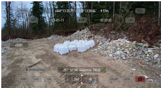
Figure -1 Looking southerly at the meg bags on site
