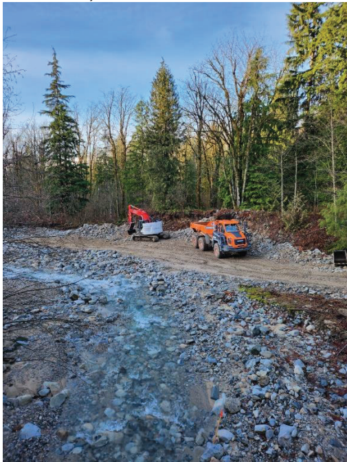
PHOTO #3 – Boney material used to armor eroded bank
