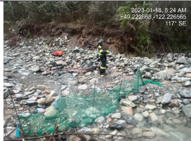
Photo 12. Backfilling for bank stabilization in the East side old creek channel (Jan 18, 2023).
