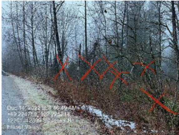
Photo 1. Trees to be felled for site access. SEI performed wildlife tree and Oregon forests nail surveys prior to tree removal (Dec. 14, 2022).
