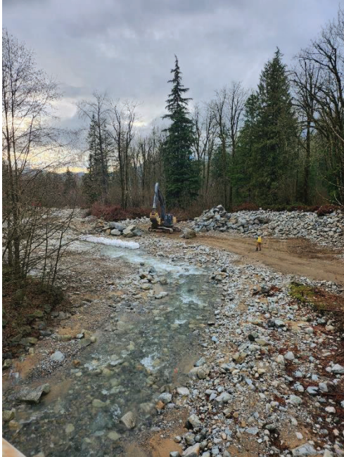
PHOTO #3 – Excavator sorting rip rap below bridge
