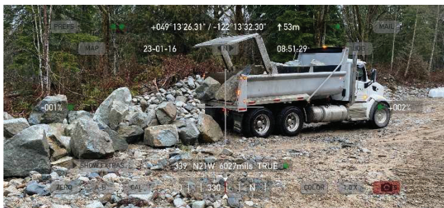
Figure -1 Looking at delivery of 1000kg rip rap to site
