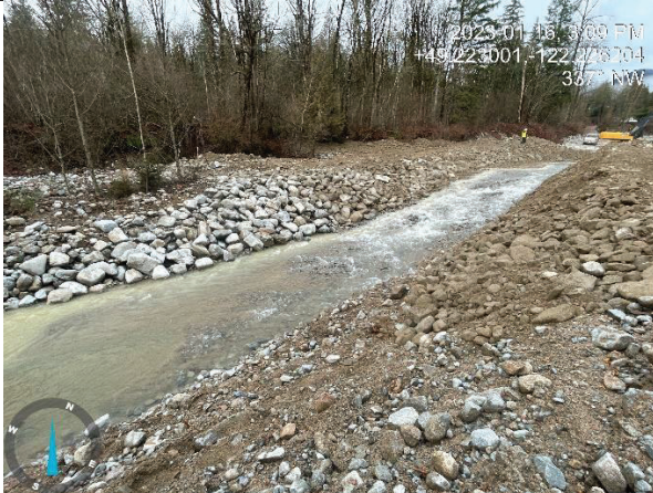
Photo 7. Flow within the diversion channel, slowly removing deflection berm gravel bags by end of the day (Jan 16, 2023).
