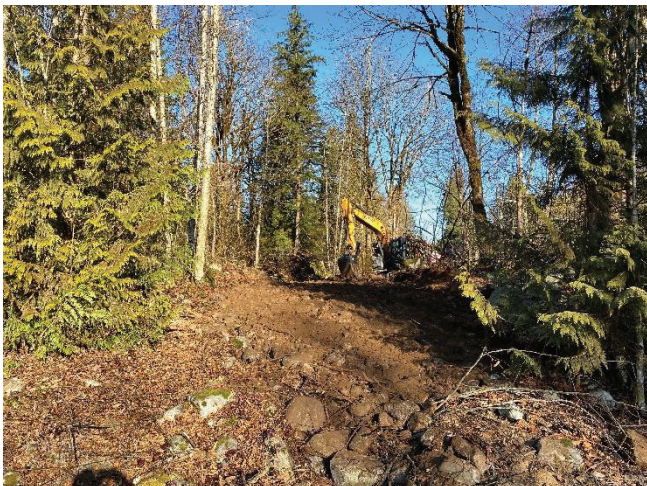
Figure -3 Looking northerly at the access clearing completed
