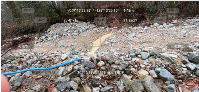
Figure -9 Looking westerly at pumped out excess water settlement
