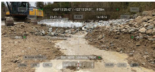
Figure -7 Looking northerly at the opening to water on the new channel
