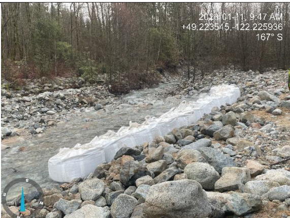
Photo 7. 13 large format gravel bags prepped for creek diversion (Jan 11, 2023).
