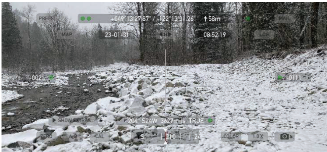
Figure -5 Looking southwesterly at creek rip rap covered in snow
