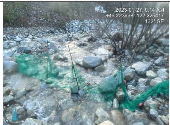
Photo 11. Southeast-facing view of fish exclusion fencing installed in the middle creek flow, removed after salvage was complete and deflection gravel berm bags removed (Jan 27, 2023).
