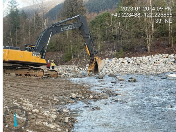
Photo 29. Excavate turbid material on inside of berm bags, and remove bags for the weekend, placing large boulders back in creek (Jan 20, 2023).
