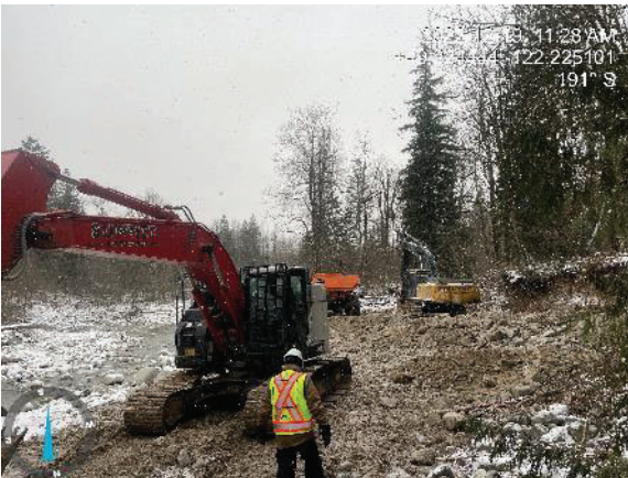
Photo 3. South-facing view of grading within the Pattison Creek floodplain above the wetted perimeter of surface water (Dec. 19, 2022).
