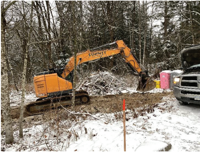
Figure - Looking westerly at rock being placed for access ramp
