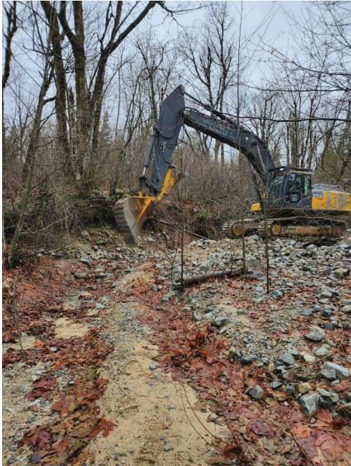
PHOTO #3 – Boney material used to armor eroded root mass
