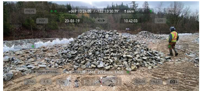
Figure -4 Looking at 8inch crush material stockpiled
