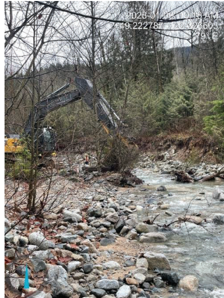
Photo 2. Tree removal for widening the creek diversion channel (Jan. 09, 2023).
