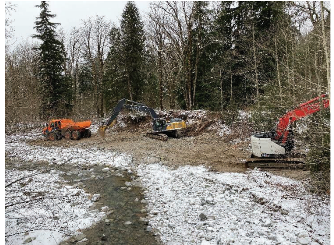
Figure -2 Looking westerly at earth works – creating a work access
