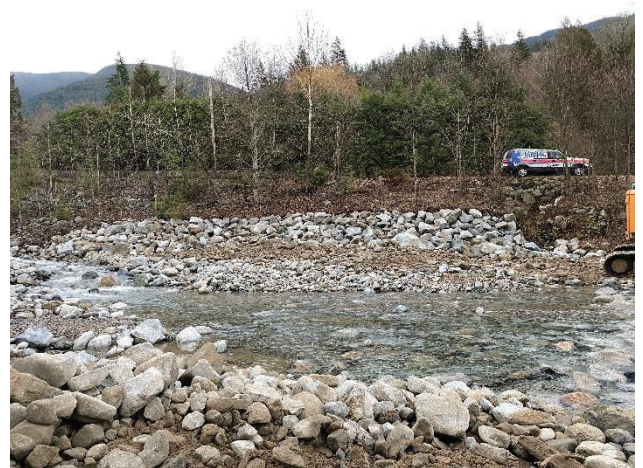
Figure - Looking easterly at the completed placement of rip rap on east bank -erosion protection
