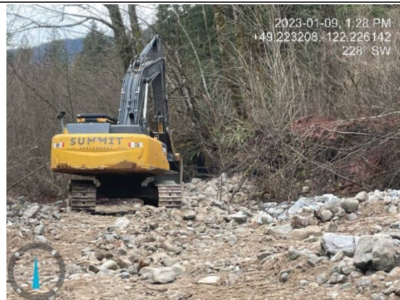
Photo 2. Tree removal for widening the creek diversion channel (Jan. 09, 2023).
