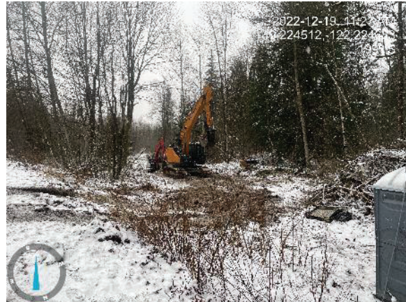
Photo 2. South-facing view of grading of the access road, above the wetted perimeter of Pattison Creek (Dec. 19, 2022).
