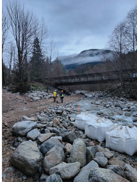
PHOTO #2 - Channel peeled back by 245 Excavator below bridge
