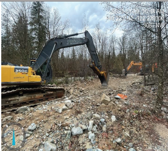
Photo 3. Tree and woody debris removal, widening diversion creek extension (Jan 9, 2023).
