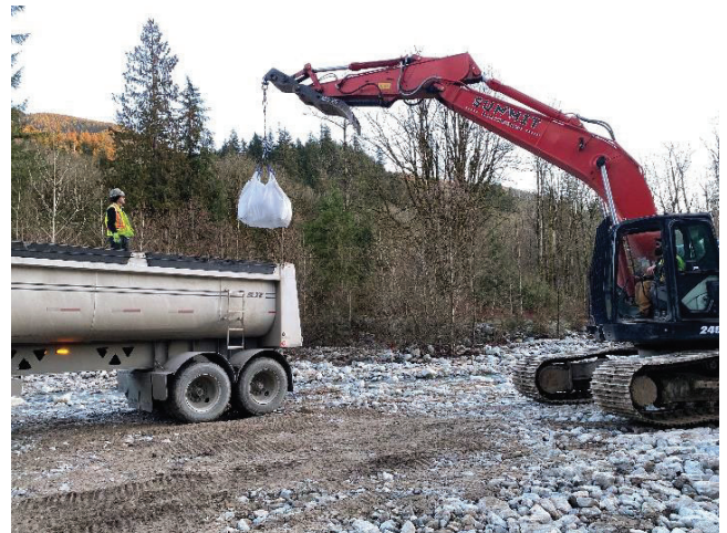
Figure -2 Looking southerly at meg bags being off loaded
