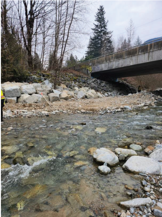
PHOTO #3 – Channel widened below bridge and rip rap armored
