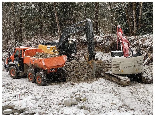
Figure -4 Looking at excavator loading up the rock truck
