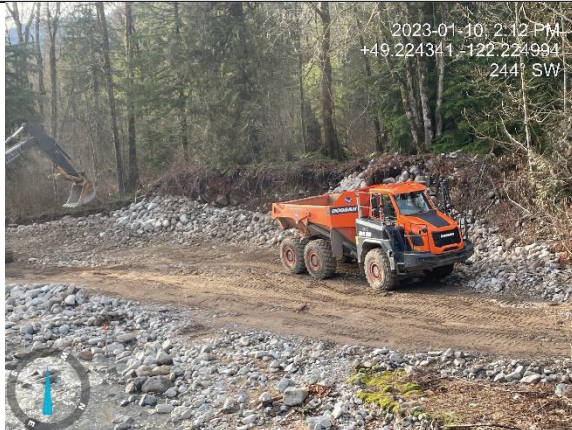
Photo 5. West bank stabilization (Jan 10, 2023).
