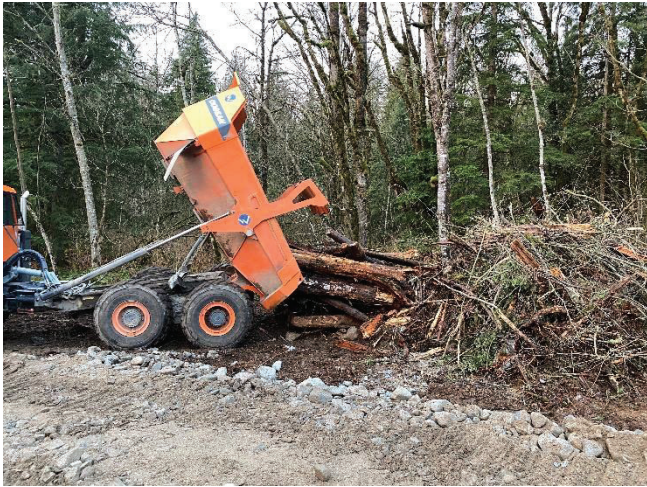
Figure -1 Looking westerly at the unloading of debris
