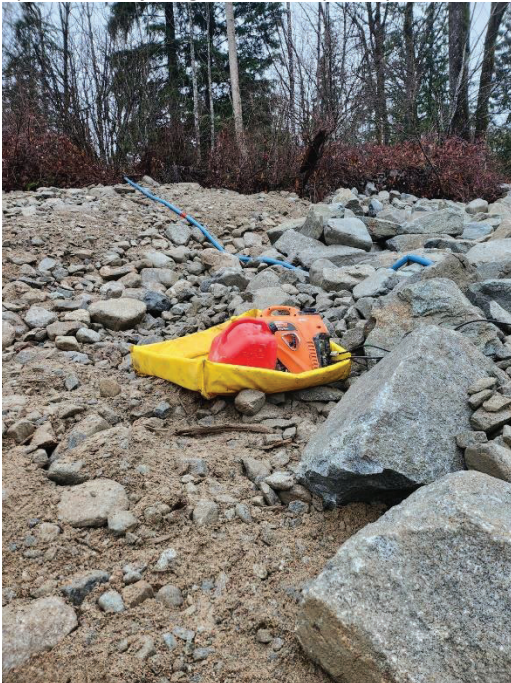
PHOTO #3 – Water pump on hand to disburse turbid water into riparian area; fuel/generator in spill tray
