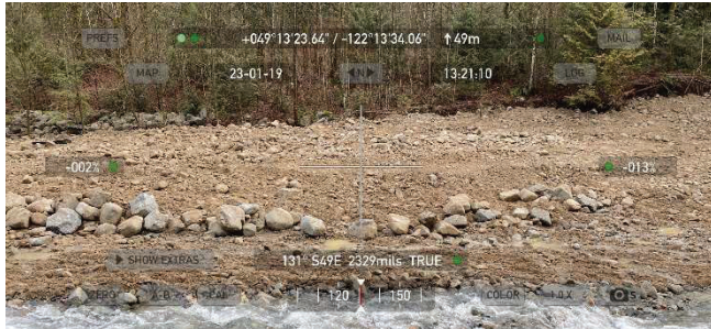
Figure -7 Looking easterly at the infill section midway
