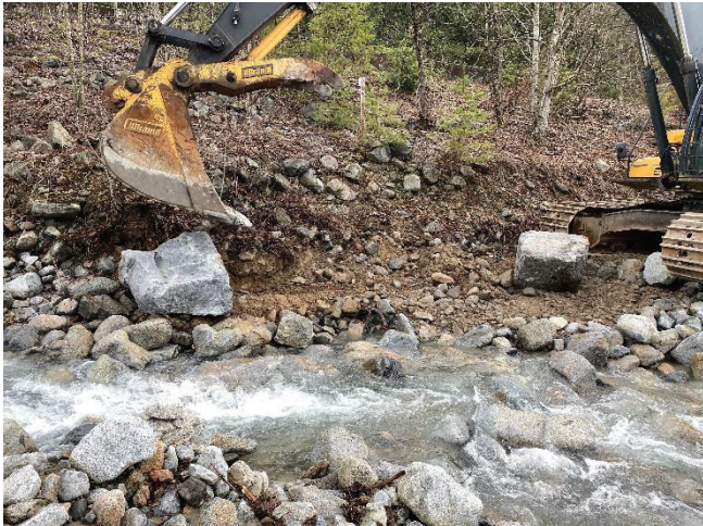
Figure - Looking easterly at start of rip rap placement- keying in
