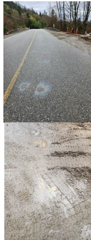
PHOTO #4 – Oil leak visible immediately after dump truck delivery
