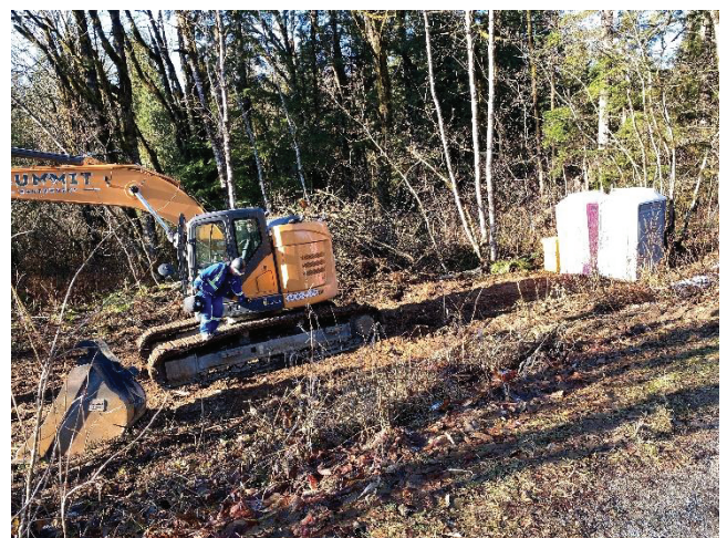
Figure -4 Looking at excavator, Washrooms & spill kit in access ramp area at day end
