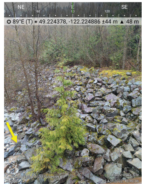
Riprap on Left Bank upstream of Sylvester Road Bridge
