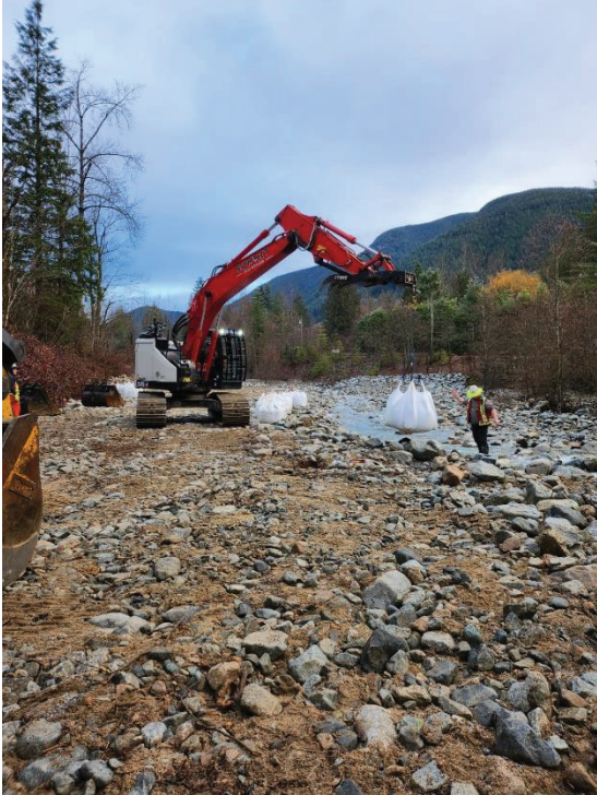
PHOTO #1 – Sang bag placement at top of diversion channel
