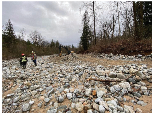
Figure - Looking southerly at created access road on the creek
