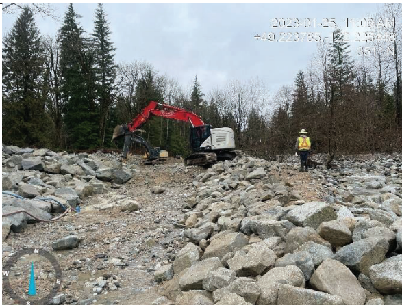
Photo 6. North-facing view of excavation of the river right diversion channel looking up. Riprap placement on right bank, as well armoring opposite bank with boulders (Jan 25, 2023).
