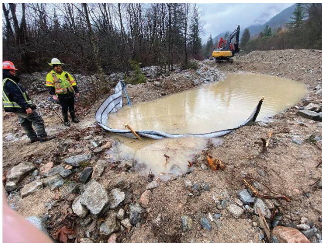
Figure -11 Looking northerly at installed settlement fencing
