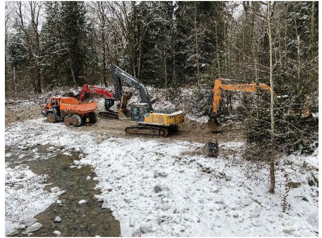
Figure - Looking westerly at excavators moving rock truck to access ramp
