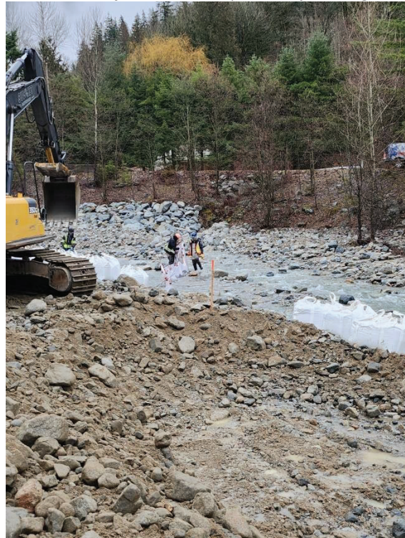
PHOTO #4 – Fish fence removed upstream of sandbags
