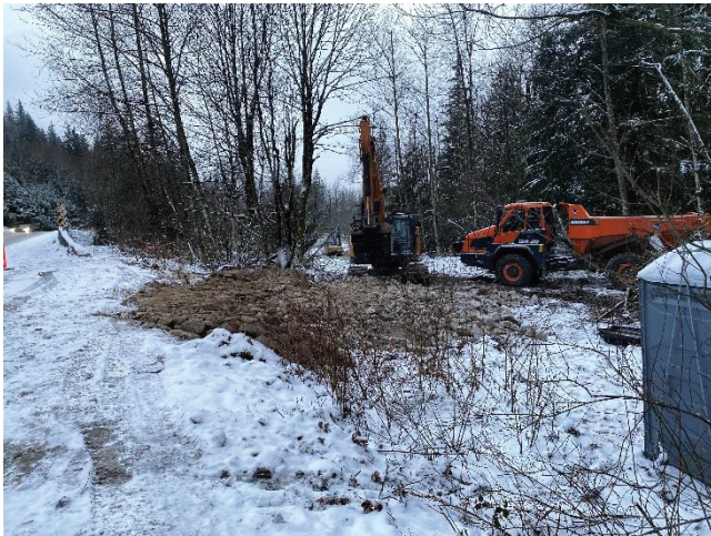
Figure - Looking southerly at the new access ramp
