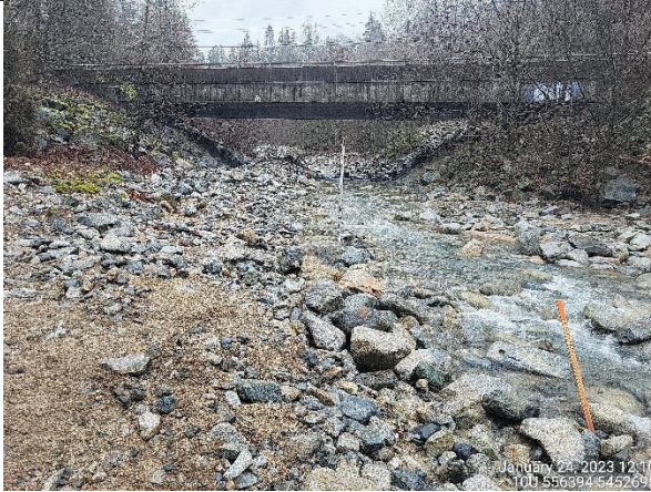
Photo 4. Northeast facing view prior to day's works below the bridge (Jan 24, 2023).
