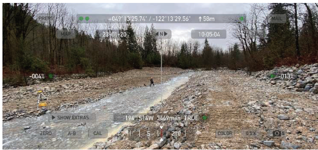
Figure -1 Looking southerly at new diverted creek
