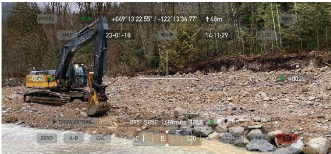
Figure -5 Looking at mid section of the infill works
