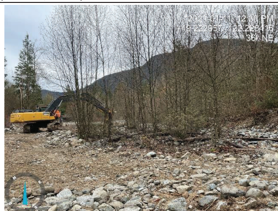
Photo 8. Tree removal to widen creek diversion channel and use material for East bank stabilization (Jan 11, 2023).
