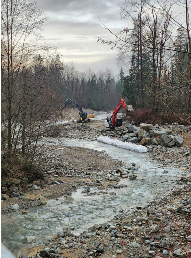
PHOTO #3 – Pulse of turbid water during channel widening and sand bag removal
