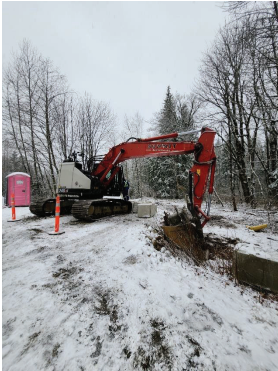
PHOTO #3 – Lockblocks placed on and adjacent to road access
