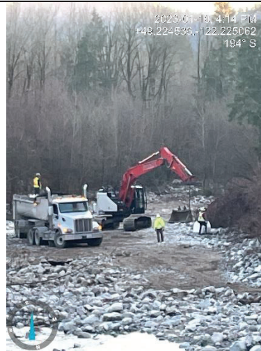
Photo 6. 26 gravel bags were delivered onsite (Jan. 10, 2023).
