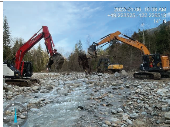
Photo 6. rock placement to minimize sediment upheaval for stream crossing (Jan 06, 2023).
