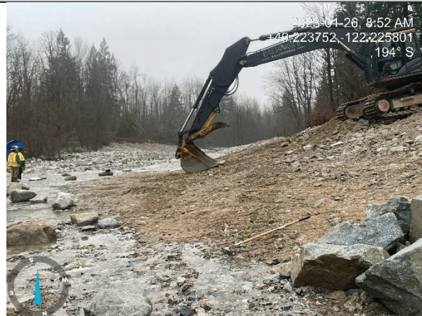
Photo 8. South-facing view of bank contouring along the right bank (Jan 26, 2023).
