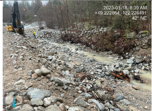
Photo 10. Old creek channel back filling after all electrofishing has been finished and salvage complete (Jan. 18, 2023).
