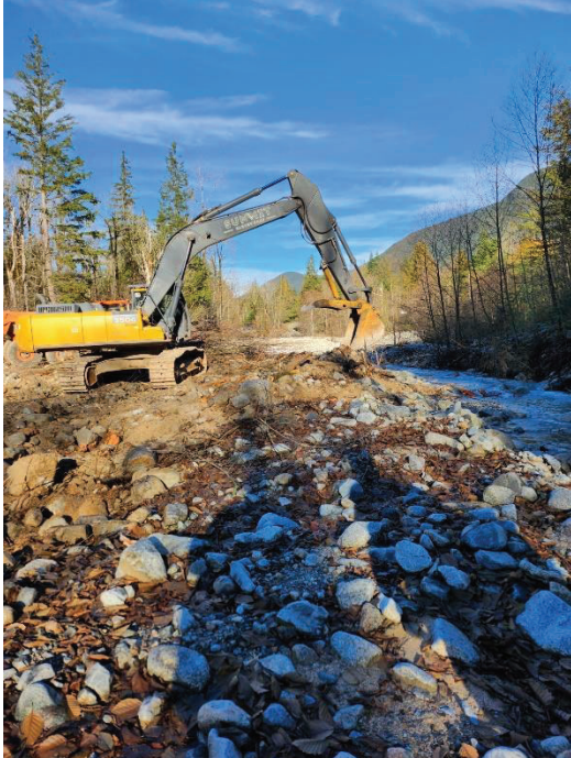
PHOTO #3 – East side of diversion channel after tree removal
