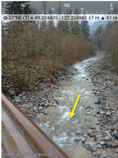
Pattison Creek: Viewing Upstream from Sylvester Road Bridge
