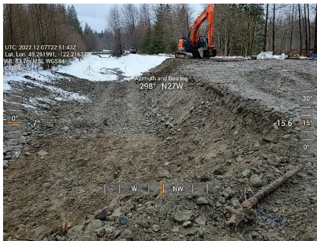
Figure 2-3 Richco - Sediment Removal Progress
