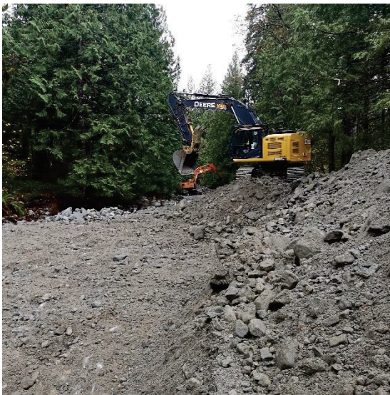
Figure 2-7 Jakes - Upstream Truck Turn-Around Construction
