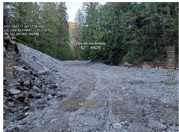
Figure 2-8 Jakes - End of Day Progress
