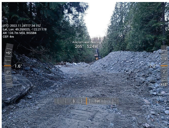
Figure 2-7 Jakes - On-going Sediment Stockpiling
