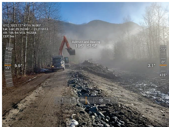
Figure 2-3 Richco – Sediment Removal Progress
