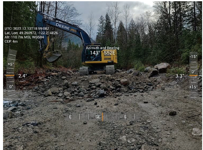
Figure 2-6 Jakes – Sediment Removal Progress
