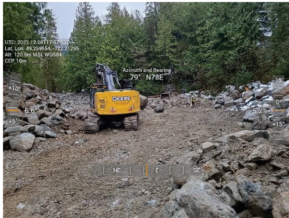
Figure 2-5 Jakes – On-going Sediment Removal
