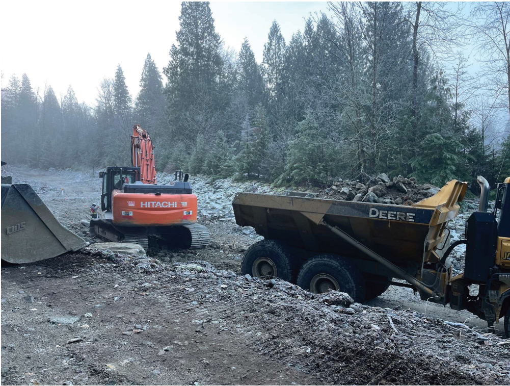
Photo 2. Jakes loading rock truck to be hauled to Richco's temporary stockpile.
