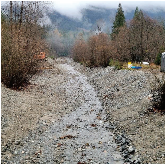
Figure 2-3 Richco – Sediment Removal Progress
