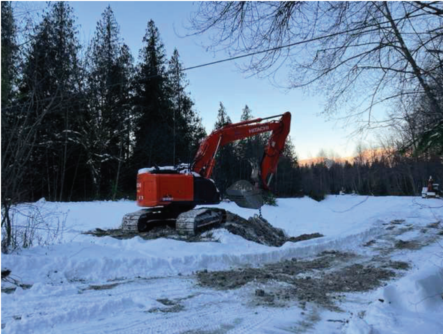
Photo 1. Richco removing material from downstream of Carratt Road bridge.
