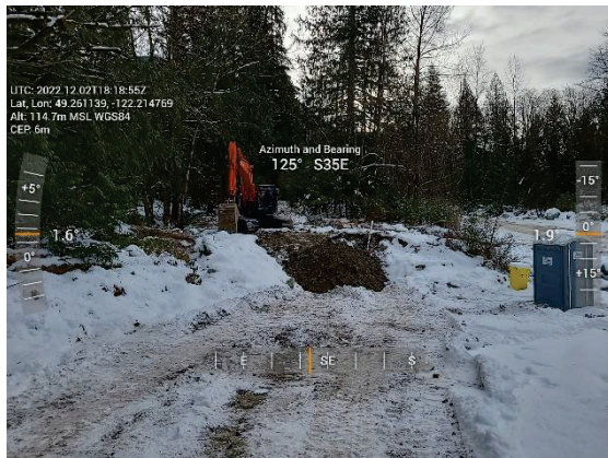
Figure 2-1 Richco - Access ramp creation (HESCO Baskets)
