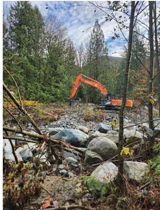
PHOTO #4 – Richco's excavator prepping access for temporary crossings to upper reach
