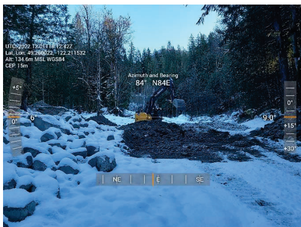
Figure 2-5 Jakes – Channel Shaping/Sediment Removal
