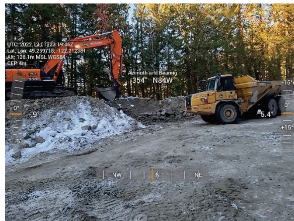
Figure 2-6 Jakes – Removal of Stockpiled Channel Sediment
