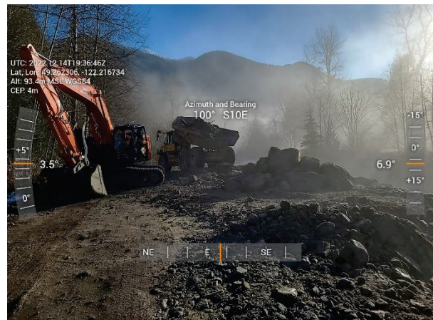
Figure 2-1 Richco – Sediment Removal Progress
