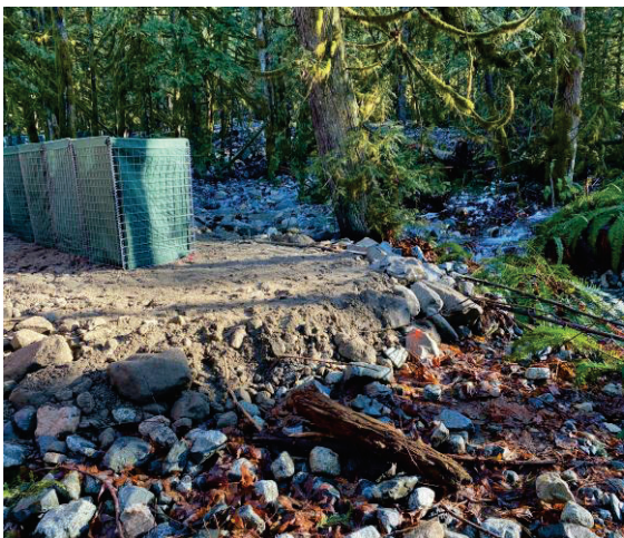
Figure 2-3 Richco - HESCO Basket Progress
