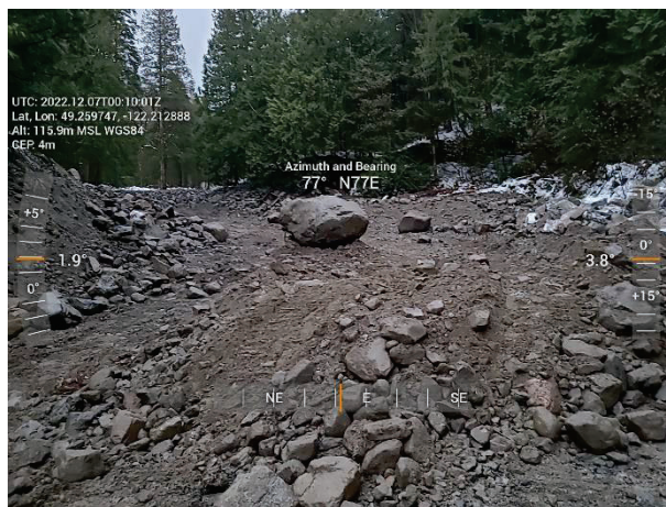
Figure 2-7 Jakes – End of Day Progress
