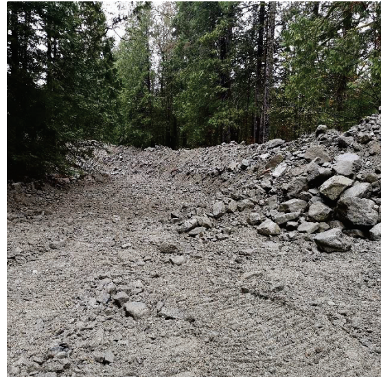
Figure 2-6 Jakes – Stockpiling of Channel Sediment
