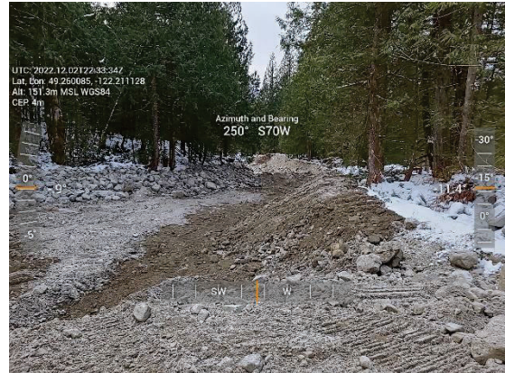
Figure 2-6 Jakes - Channel Grading
