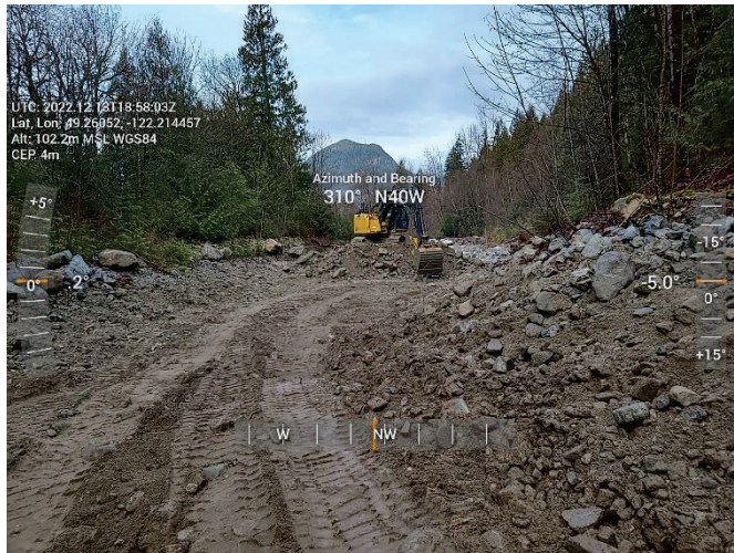
Figure 2-5 Jakes – Sediment Removal Progress
