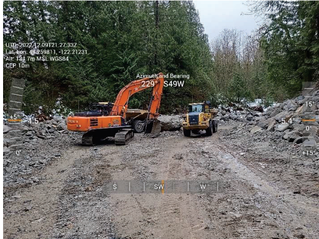
Figure 2-5 Jakes – On-going Sediment Removal
