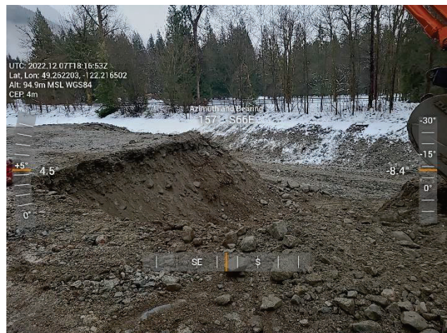
Figure 2-4 Richco - Sediment Removal Progress
