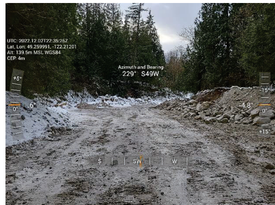
Figure 2-8 Jakes - End of Day Progress
