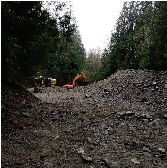
Figure 2-7 Jakes – On-going Sediment Stockpiling
