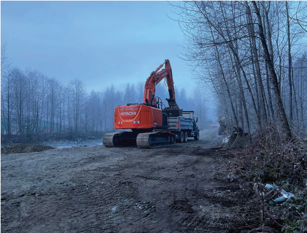
Photo 1. Richco loading haul trucks with temporary stockpile.
