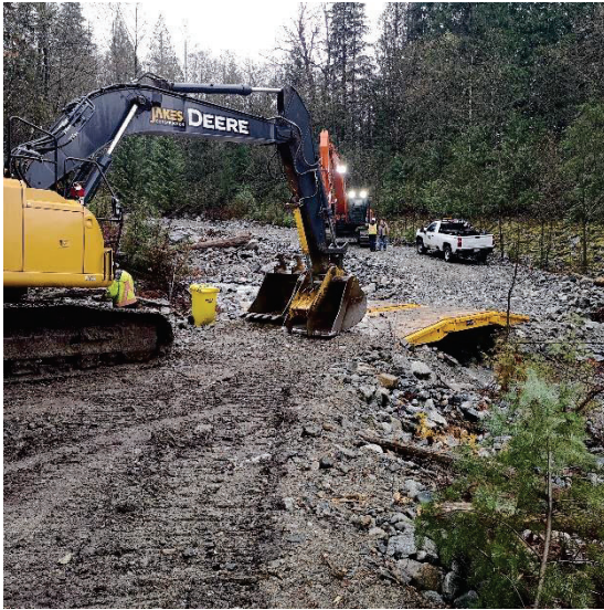
Figure 2-5 Jakes - Temporary Bridge Installation
