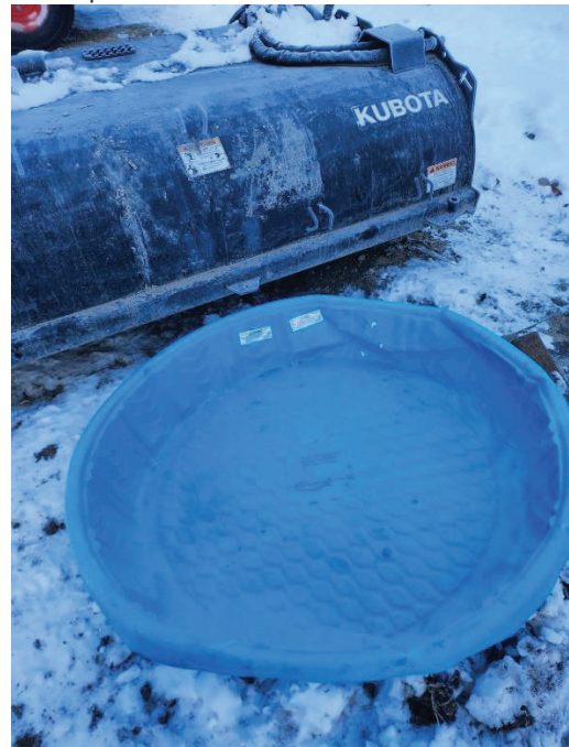
PHOTO #4 – Spill tray at beginning of worksite, adjacent to street sweeper
