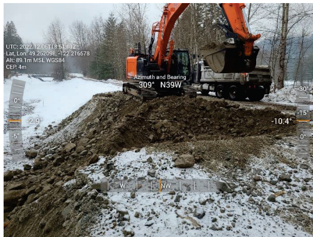
Figure 2-3 Richco - Sediment Removal Progress
