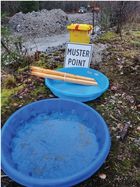
PHOTO #3 – Spill trays and Spill kit onsite
