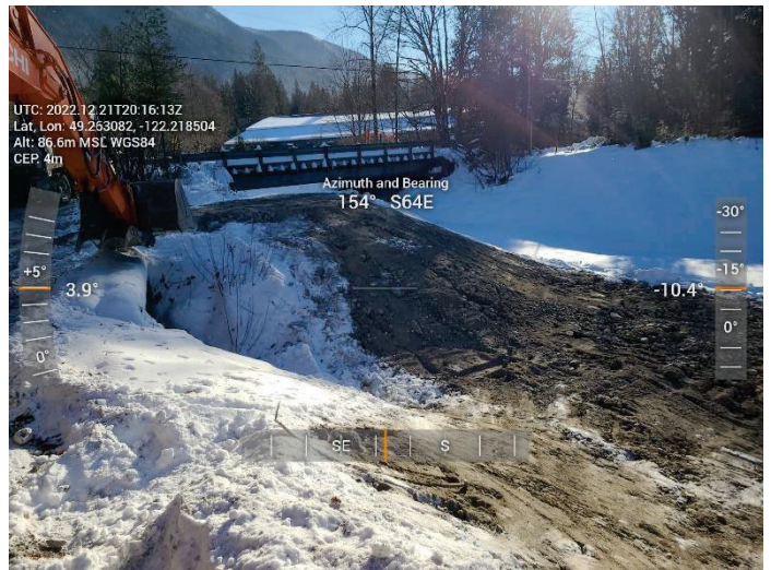
Figure 2-4 Richco- Completed Sediment Removal
