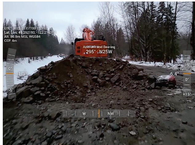
Figure 2-4 Richco - Sediment Removal Progress
