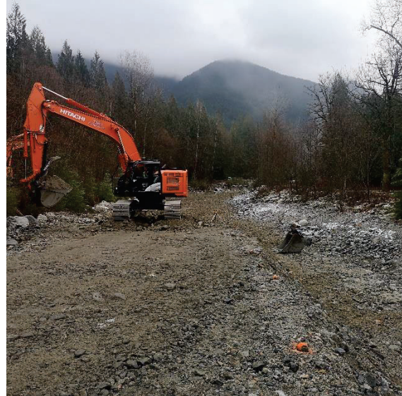
Figure 2-1 Richco - Sediment Removal Progress
