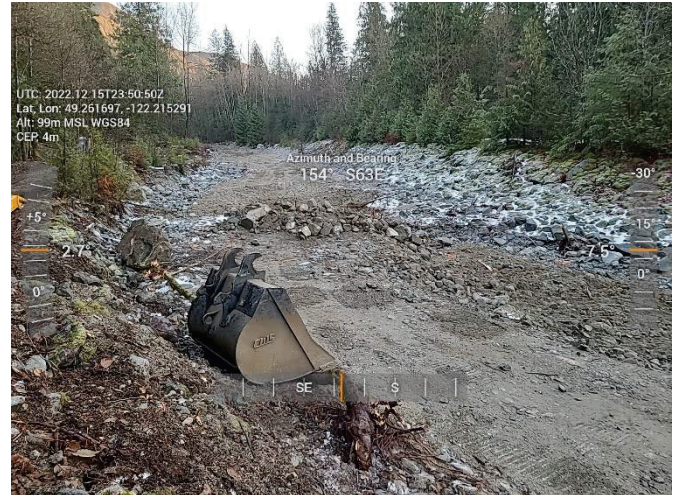
Figure 2-6 Jakes – Sediment Removal Progress
