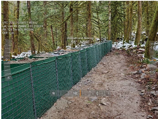
Figure 2-1 Richco - HESCO Basket Progress
