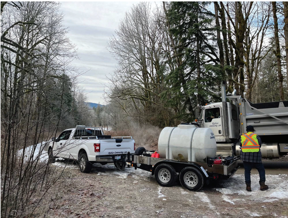
Photo 3. Wash station on Eng Road to clean off haul trucks when exiting Eng Pit.
