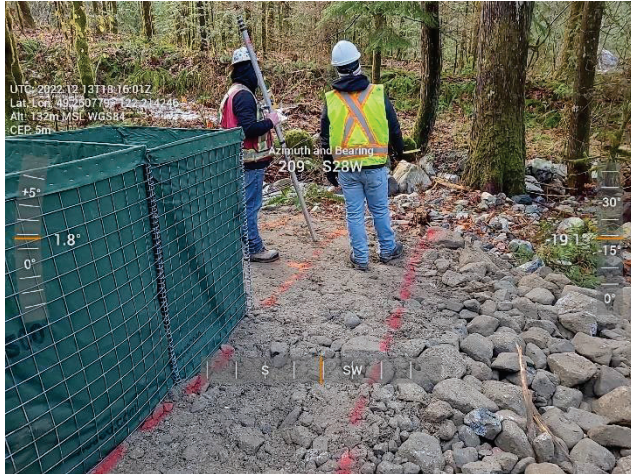
Figure 2-1 Richco - HESCO Basket Progress
