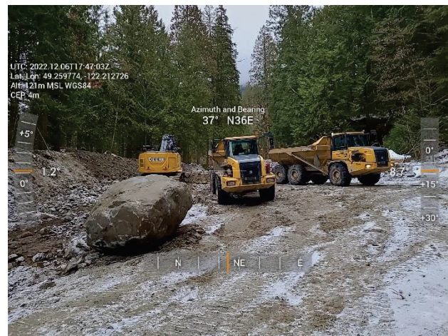
Figure 2-6 Jakes – Removal of Channel Sediment
