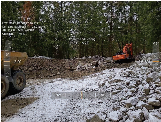
Figure 2-5 Jakes – Removal of Channel Sediment
