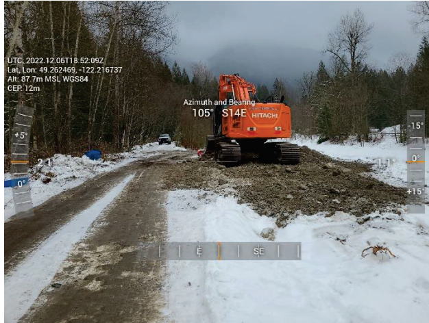
Figure 2-1 Richco - Sediment Removal Progress
