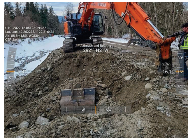
Figure 2-4 Richco - Sediment Removal Progress
