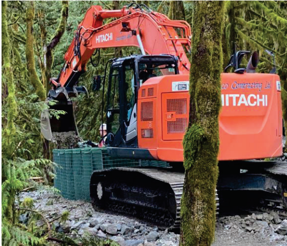
Figure 2-1 Richco - HESCO Basket Progress
