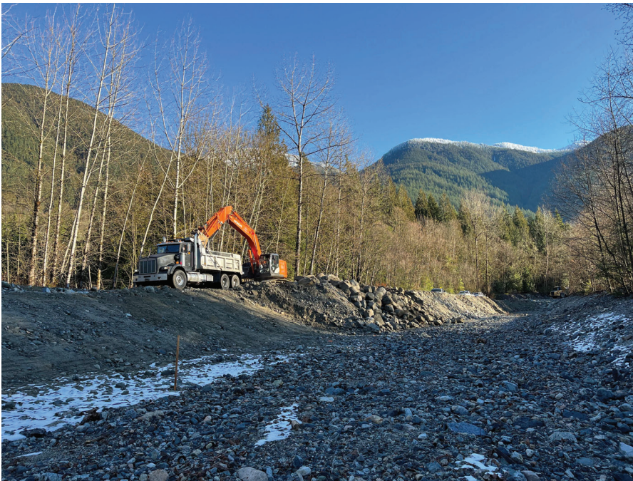
Photo 1. Richco loading haul trucks with temporary stockpile.
