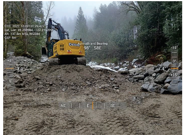
Figure 2-6 Jakes – On-going Sediment Removal
