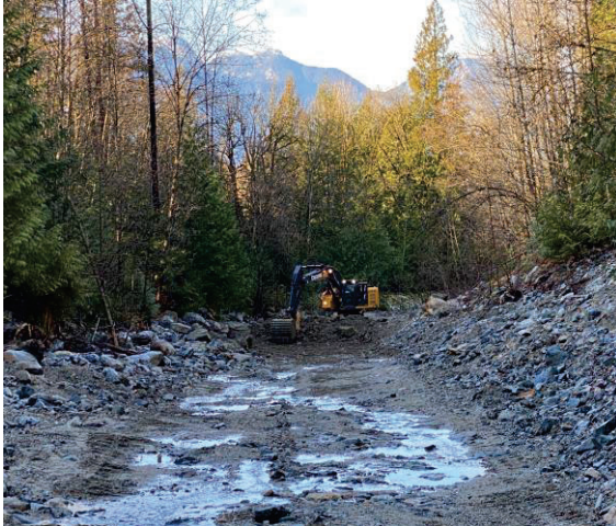
Figure 2-5 Jakes – Shaping creek to grade
