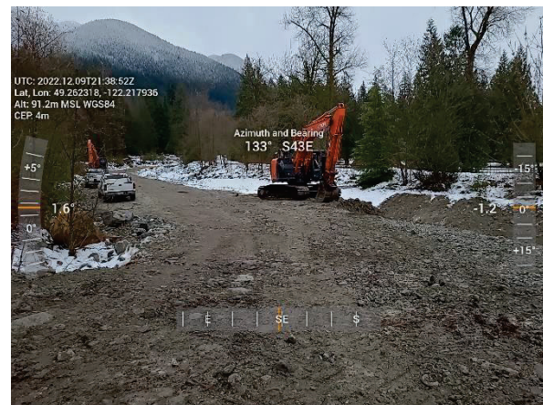
Figure 2-4 Richco - Sediment Removal Progress
