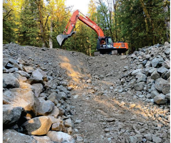
Figure 2-6 Jakes – Diversion Removal Progress
