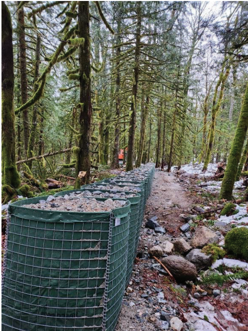
PHOTO #3 – Hesco Baskets assembled, filled, placed along wetted area in lower reach
