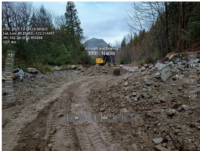
Figure 2-5 Jakes – Sediment Removal Progress
