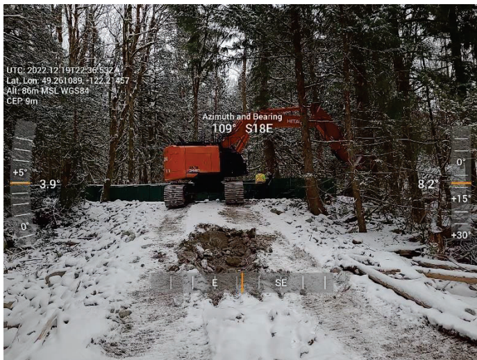
Figure 2-3 Richco – HESCO Baskets Progress
