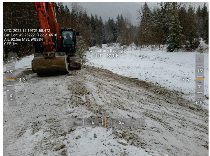
Figure 2-1 Richco – Completion of Sediment Removal
