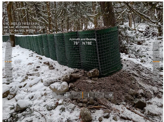
Figure 2-4 Richco- Completion of HESCO Baskets
