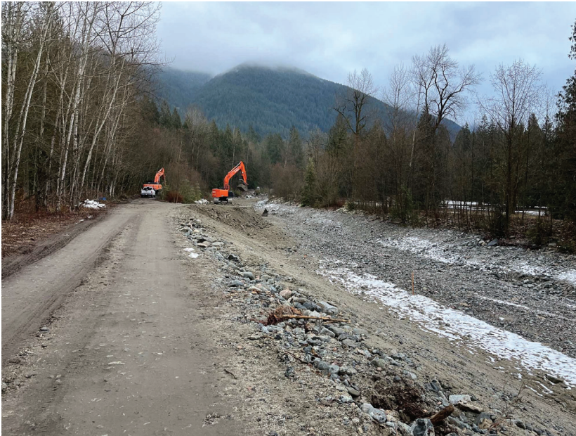
Photo 2. Richco's work location along the dike road.
