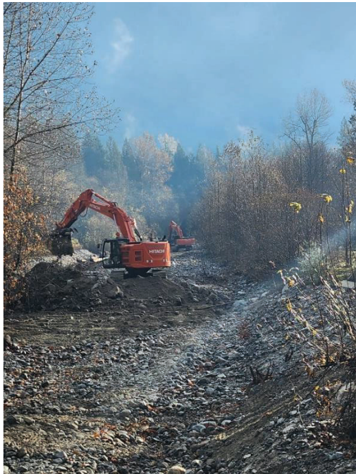
PHOTO #3 – Jake's excavation of lower reach upstream of Carrat Rd Bridge
