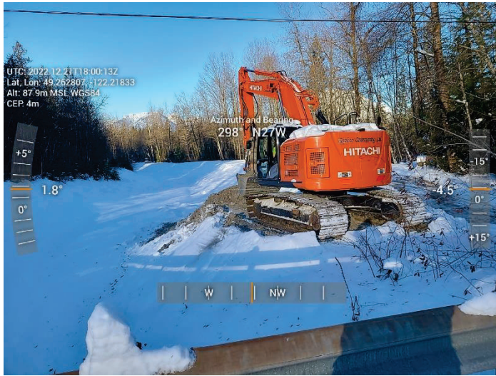
Figure 2-1 Richco – Sediment Removal Progress
