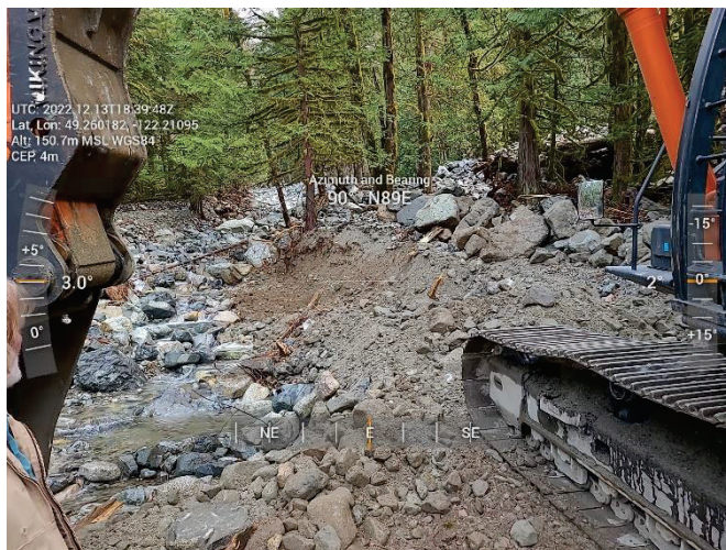
Figure 2-7 Jakes – Channel Restoration Works
