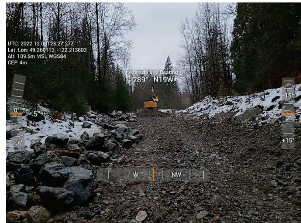
Figure 2-8 Jakes – End of Day Progress
