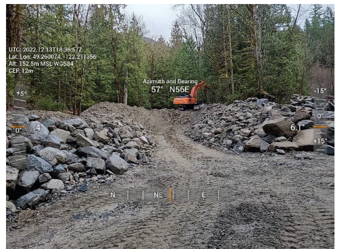
Figure 2-8 Jakes –Channel Restoration Works
