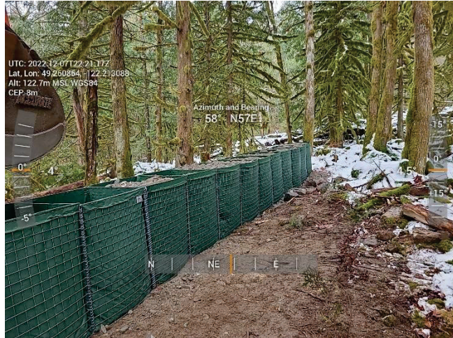
Figure 2-1 Richco - HESCO Basket Installation
