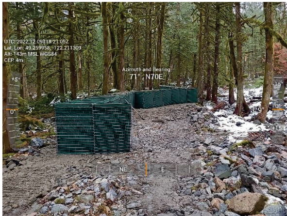
Figure 2-1 Richco - HESCO Basket Progress
