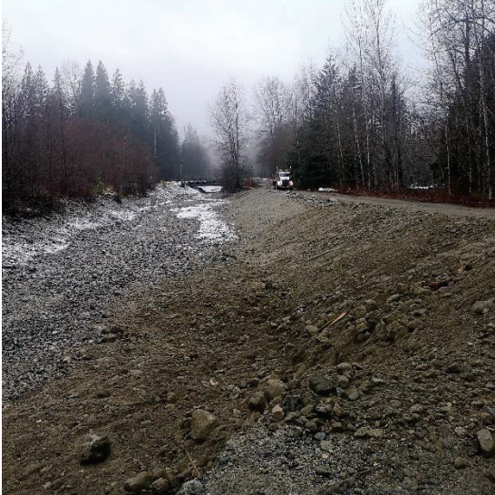
Figure 2-1 Richco - Sediment Removal Progress
