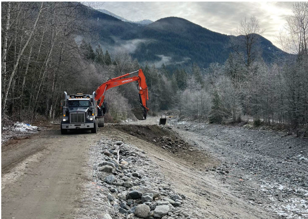
Photo 1. Richco loading haul trucks with temporary stockpile.
