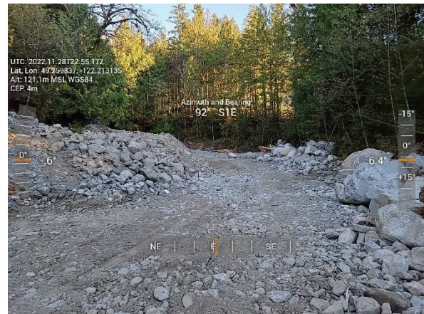
Figure 2-6 Jakes - Stockpiling of Channel Sediment
