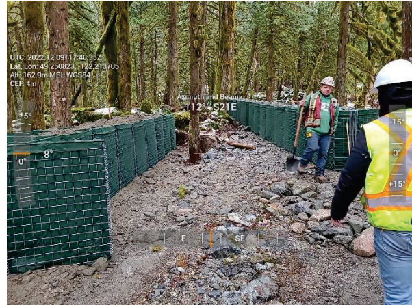
Figure 2-2 Richco - HESCO Basket Progress & Alignment Extension (Right)
