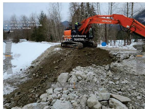
Figure 2-4 Richco - Sediment Removal Progress
