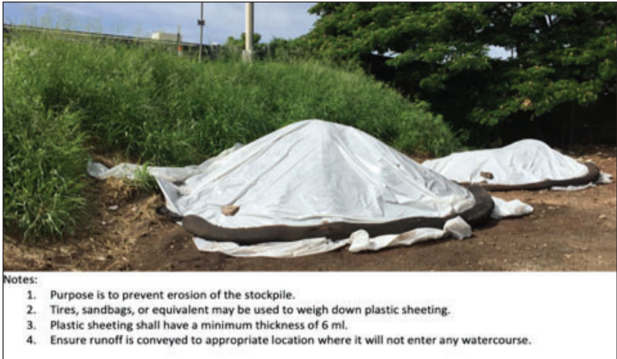
Figure 8. Stockpile protection.
