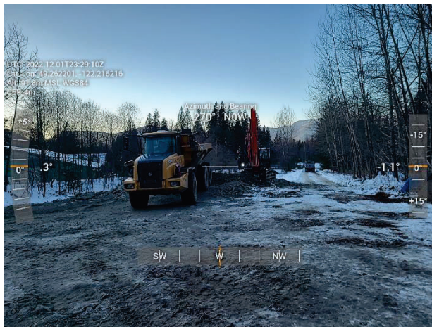
Figure 2-3 Richco - Sediment Removal Progress
