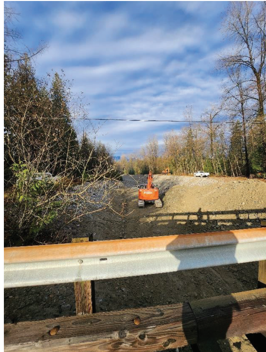
PHOTO #4 – Richco's excavator prepping access for temporary crossings to upper reach
