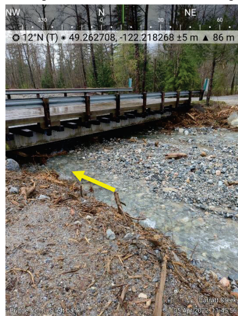
Carratt Rd Bridge: Viewing Downstream from Upstream Left Bank
