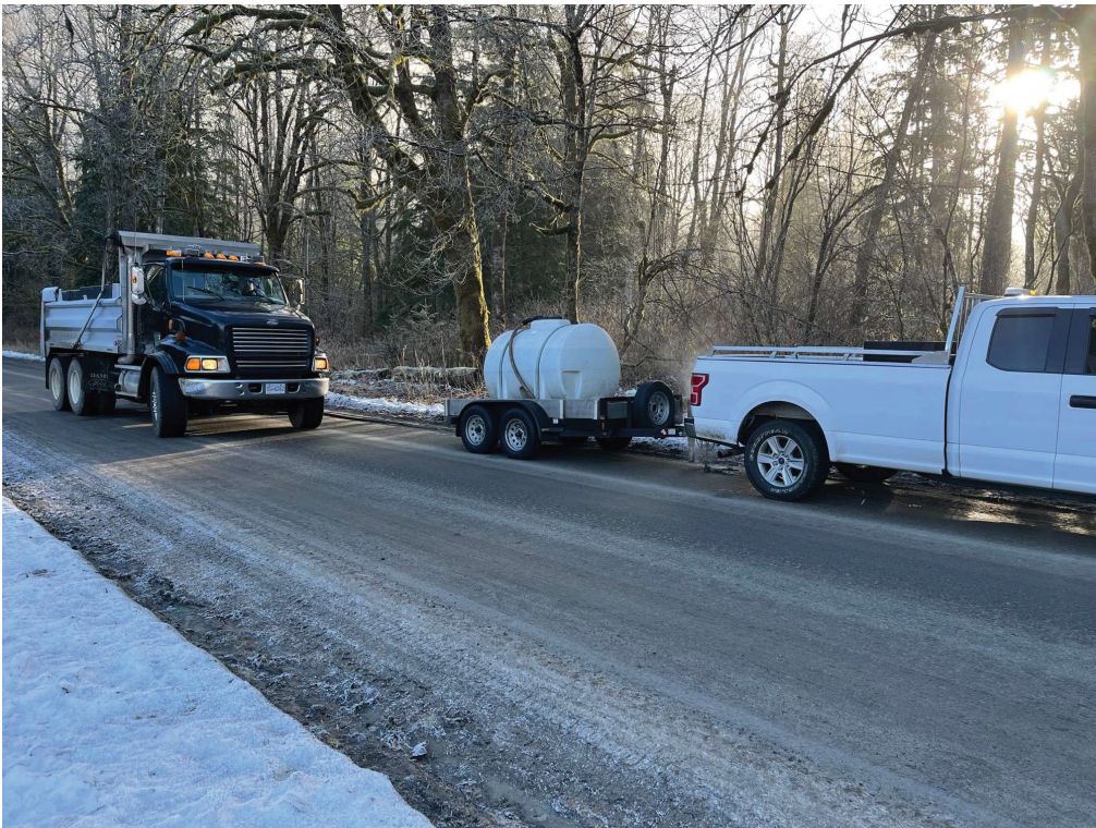
Photo 3. New wash station location on Eng Road to clean off haul trucks after exiting Eng Pit.
