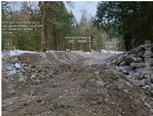
Figure 2-5 Jakes - Channel Grading
