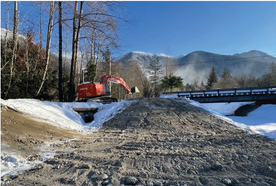
Photo 2. Completed works downstream of bridge.
