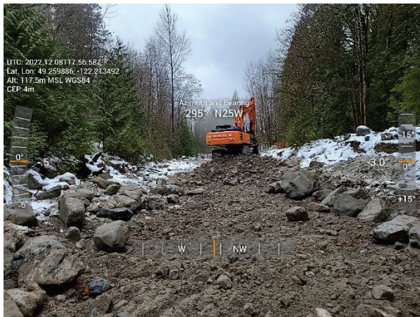
Figure 2-7 Jakes – On-going Sediment Removal
