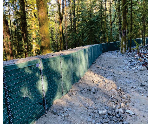
Figure 2-2 Richco - HESCO Basket Progress
