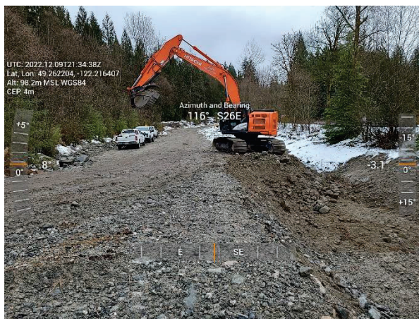
Figure 2-3 Richco - Sediment Removal Progress
