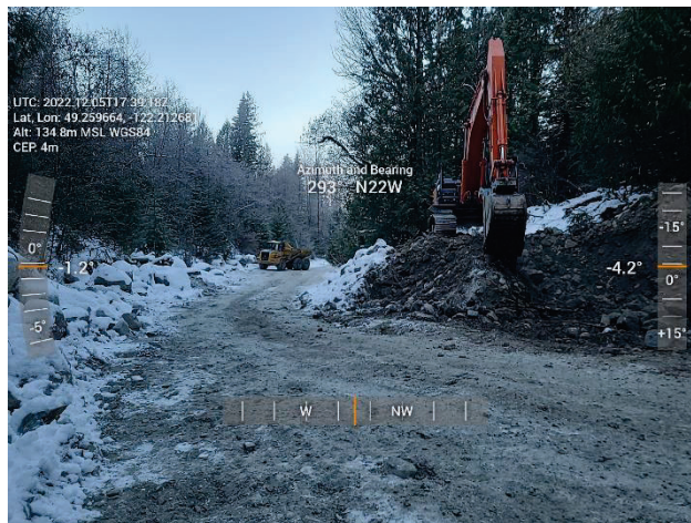
Figure 2-7 Jakes - On-going Sediment Removal
