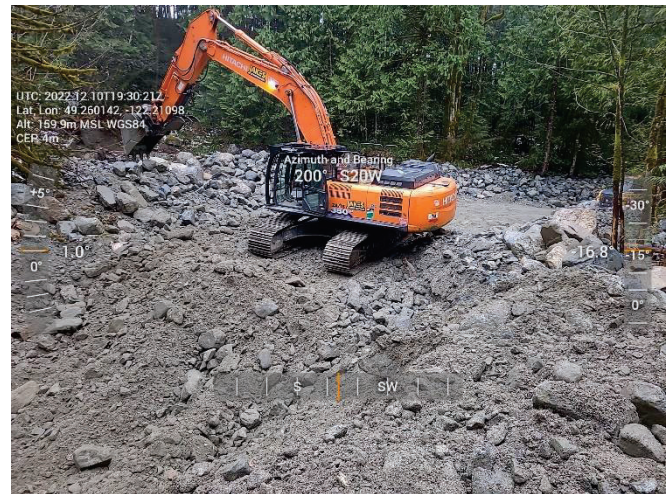
Figure 2-8 Jakes - Channel Restoration Works
