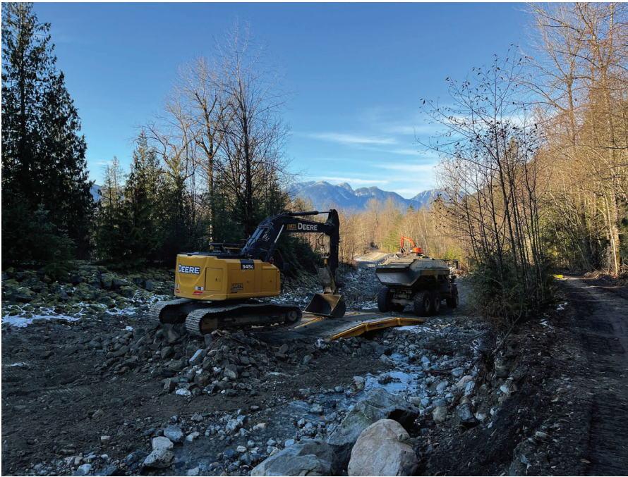
Photo 2. Jakes loading rock truck to be hauled to Richco's temporary stockpile.
