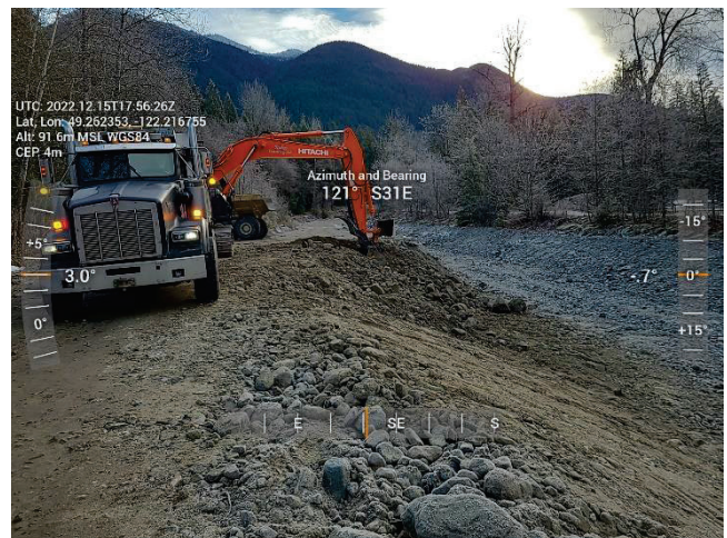
Figure 2-4 Richco – Sediment Removal Progress
