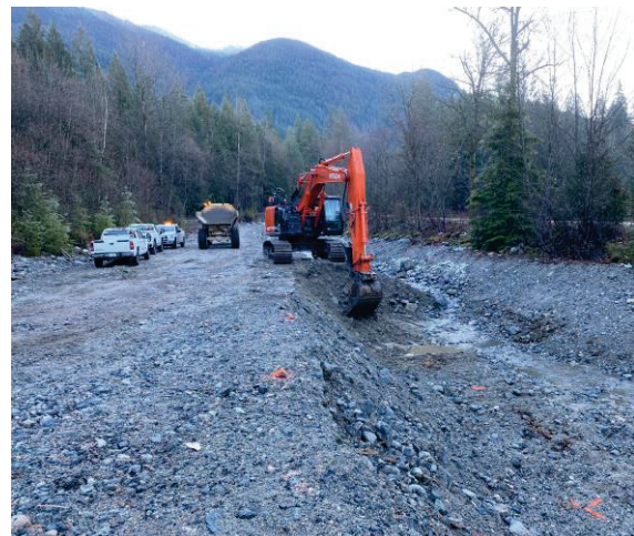
Figure 2-4 Richco - Sediment Removal Progress
