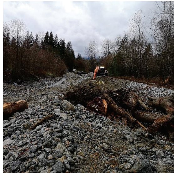
Figure 2-4 Richco – Woody Debris Removal
