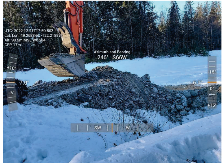
Figure 2-1 Richco – Sediment Removal Progress
