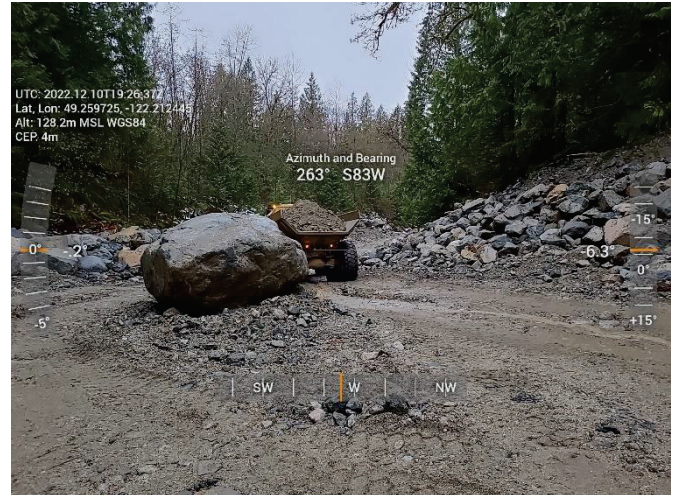
Figure 2-6 Jakes - Sediment Removal Progress
