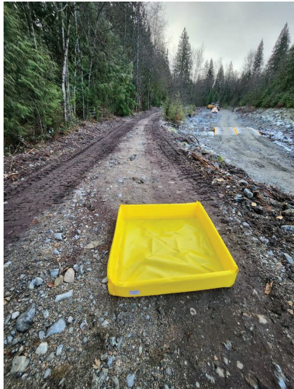
PHOTO #4 – Clean spill tray along access road into Hesco Basket area
