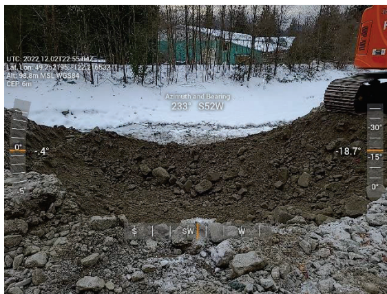
Figure 2-3 Richco - Sediment Removal Progress
