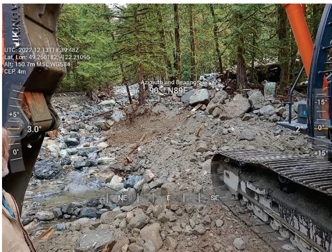
Figure 2-7 Jakes – Channel Restoration Works
