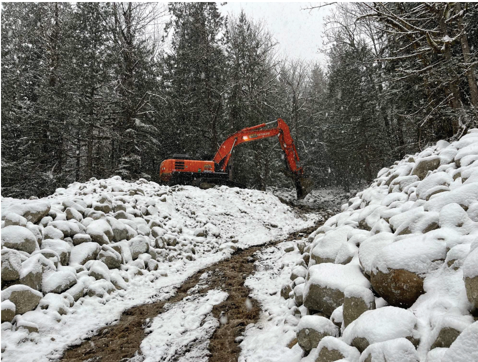
Photo 2. Jakes creating a berm across avulsion channel.
