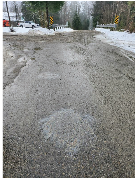
PHOTO #4 – Fuel sheen visible on Carratt Rd & dyke access road
