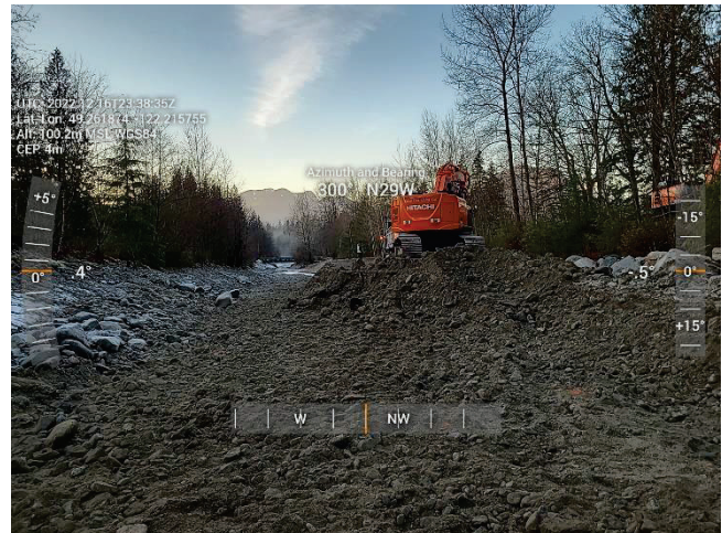
Figure 2-4 Richco/Jakes - Sediment Removal Progress
