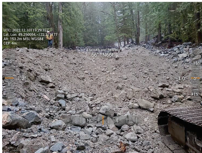
Figure 2-7 Jakes - Channel Restoration Works
