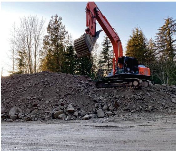
Figure 2-7 Richco – Shaping pf Stockpile at the Pit
