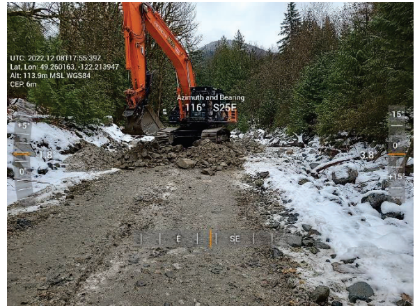
Figure 2-6 Jakes – On-going Sediment Removal
