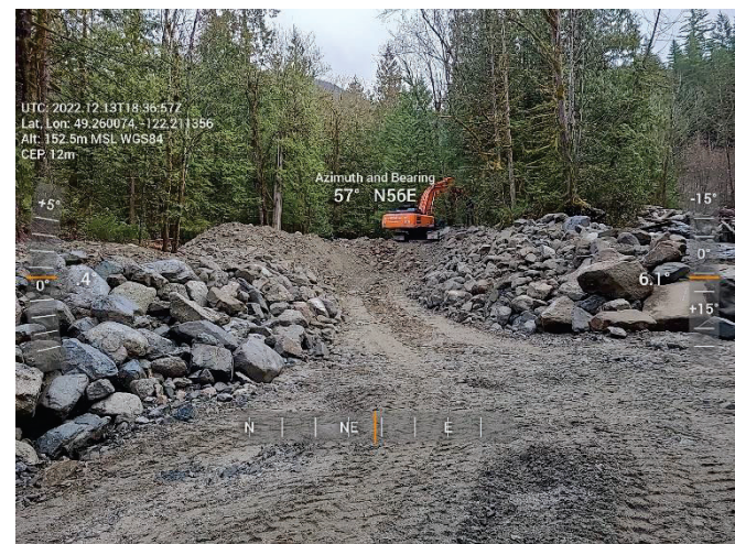
Figure 2-8 Jakes – Channel Restoration Works
