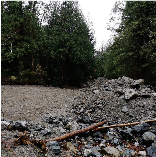
Figure 2-5 Jakes – Turn-Around Area Completion
