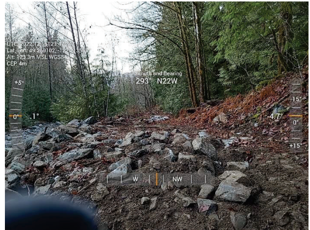
Figure 2-10 Jakes – Access Trail onto Existing Dike
