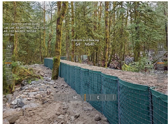
Figure 2-1 Richco - HESCO Basket Progress
