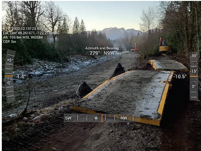
Figure 2-5 Jakes – Temporary Bridge Removal
