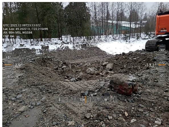
Figure 2-4 Richco - Sediment Removal Progress
