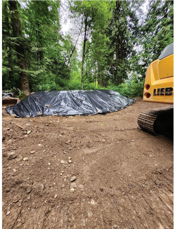
Stockpile covered with poly-sheeting
