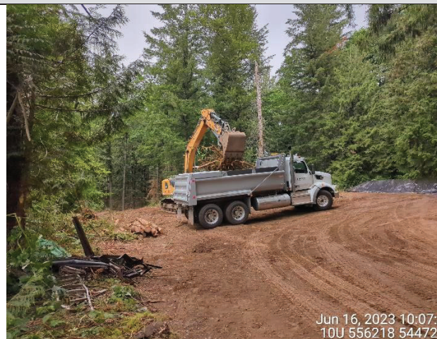
Photo 1. View of woody debris from road clearing being removed and sent to Summit's dump site. (Jun. 16, 2023).
