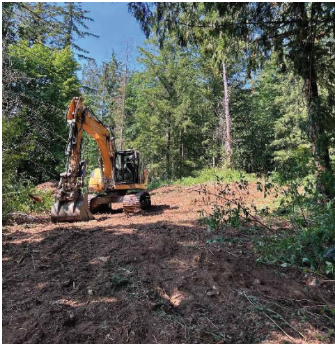
Figure 3 Excavator Clearing at the Open Area
