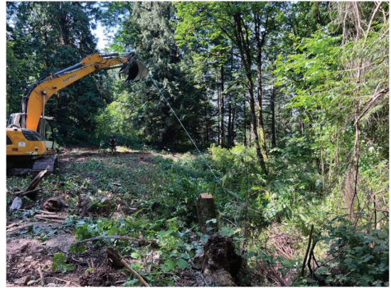
Figure 2 Excavator Pulling Organics Out of the Creek
