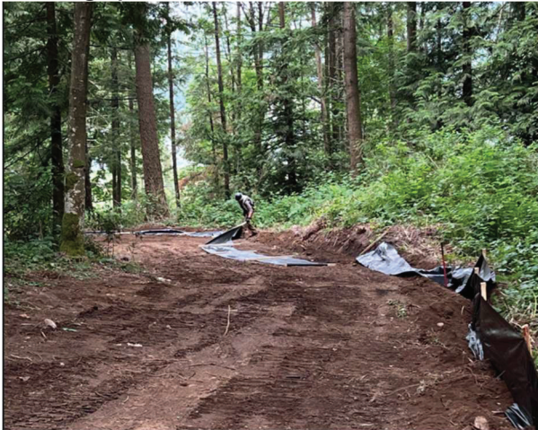
Figure 1 Installing Silt Fences Along Upper Access Road
