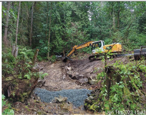
Photo 2. View of armoring of the southern bank of Davies Creek. (Jun. 16, 2023).
