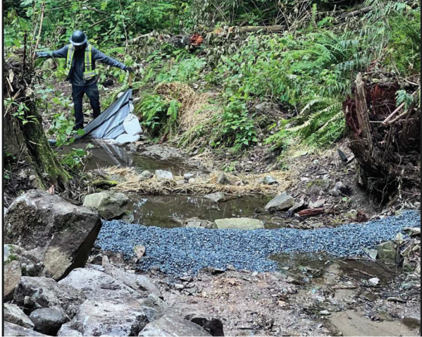
Figure 1 Removing Check Dam and Sediment Control Structure
