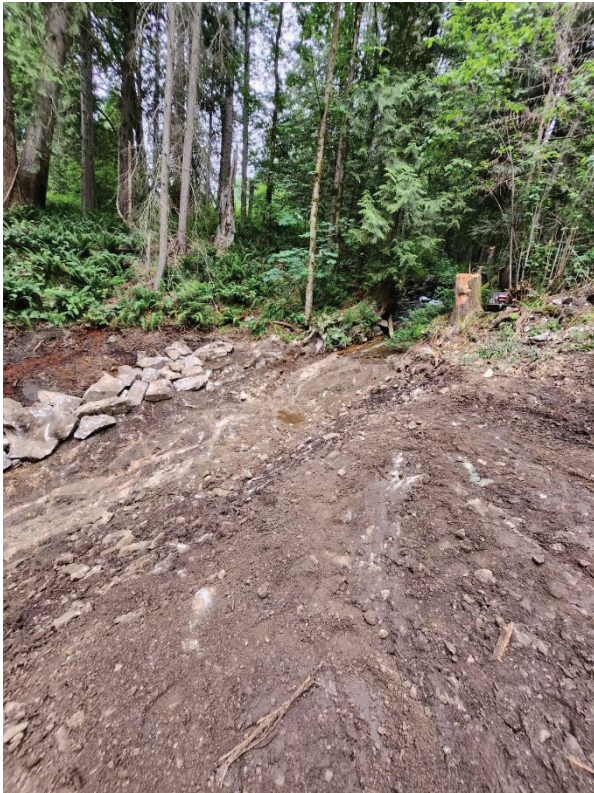
Boulder placement along north bank, looking up-stream
