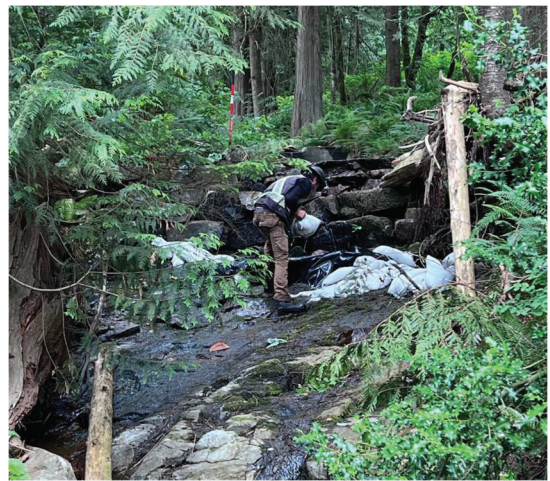
Figure 2 Sandbags Placed on Creek
