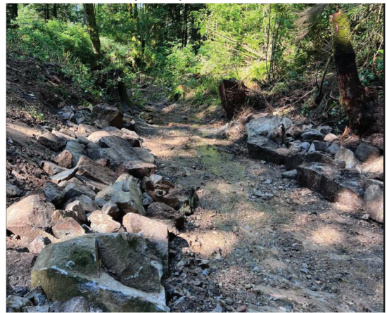
Figure 4 Looking Downstream After Removal of Check Dam
