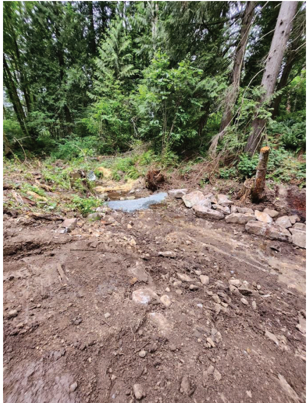
Boulder placement along north bank, downstream
