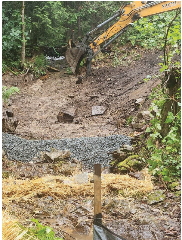
Boulder placement along north bank, downstream
