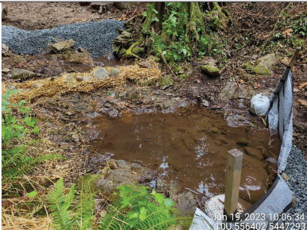
Photo 1. View of gravel, straw , and silt fence check dams set up at the top of Davies Creek. (Jun. 19, 2023).
