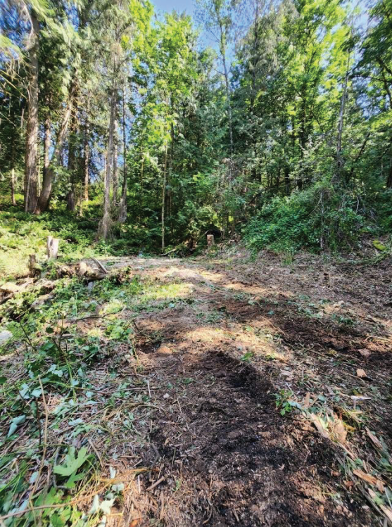
Access cleared to sediment deposit at creek
