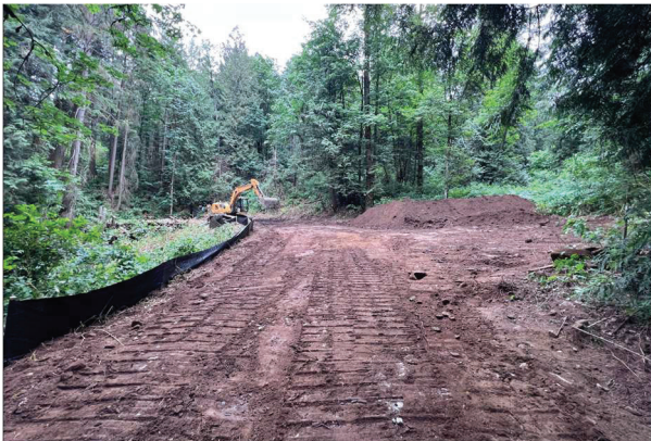
Figure 3 Upper Access Road with Silt Fences
