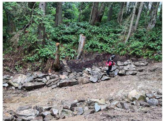
Figure 4 Sump Pump and Hoses Removed from Site
