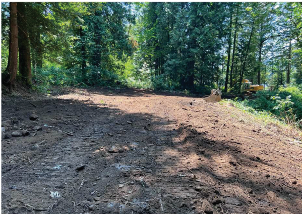
Figure 3 Spreading Soil Stockpile to Ground and Removal of Silt Fences
