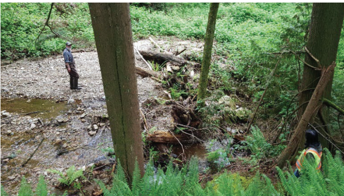
Davies Creek – Upstream Log Jam (Side Profile)
