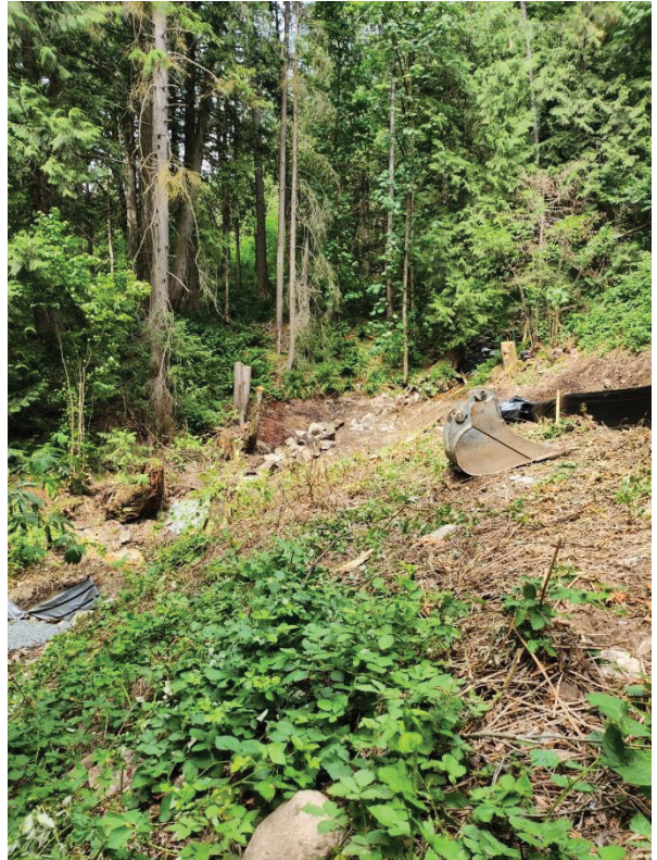
Boulder placement along North edge of bank
