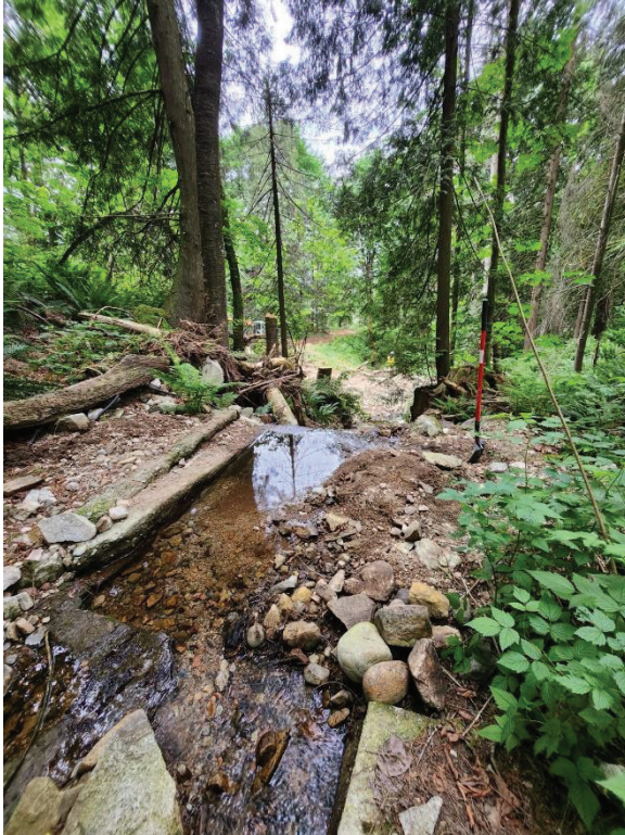
Pool dug for sump-pump preparation
