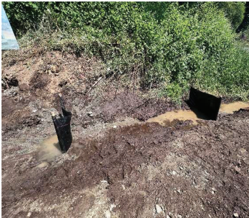
Figure 3 Silt Fences on the Ditch
