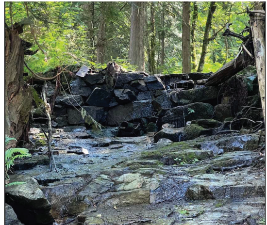
Figure 2 Temporarily Pool Removed
