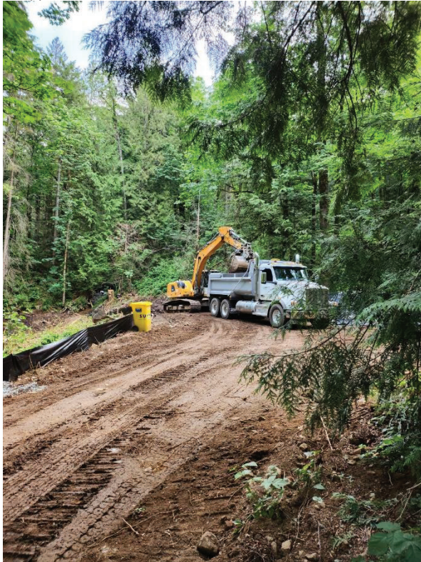
Upper reach stream sediment excavated and loaded out
