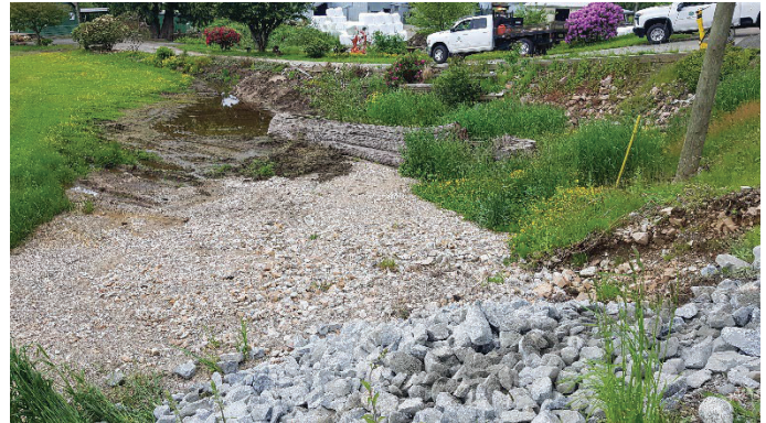
Sylvester Road – West Side Slope (Not Davies Creek)
