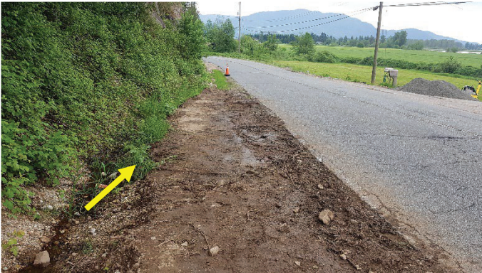
Sylvester Road – East Roadside Ditch (Not Davies Creek)
