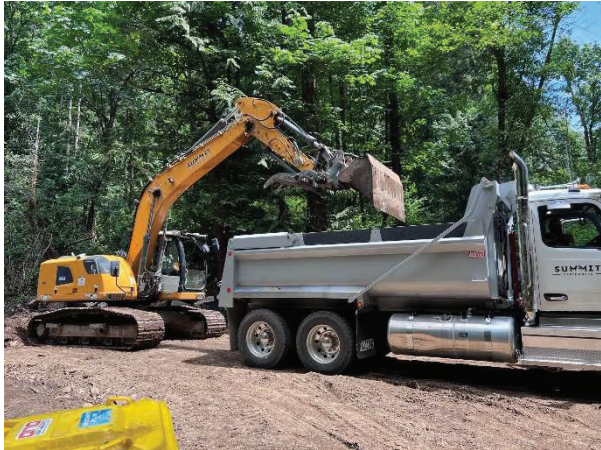
Figure 1 Loading Mix Materials to Tandem Truck
