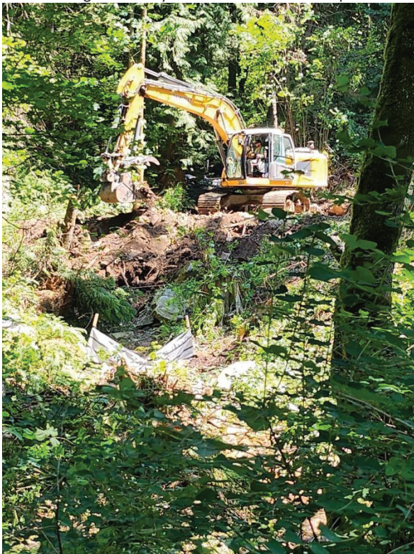
Pulling out woody debris from sediment deposit
