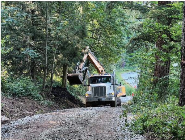
Figure 1 Loading Non-invasive Organics (Soil) to Tandem Truck and Transported to Upper Access Road
