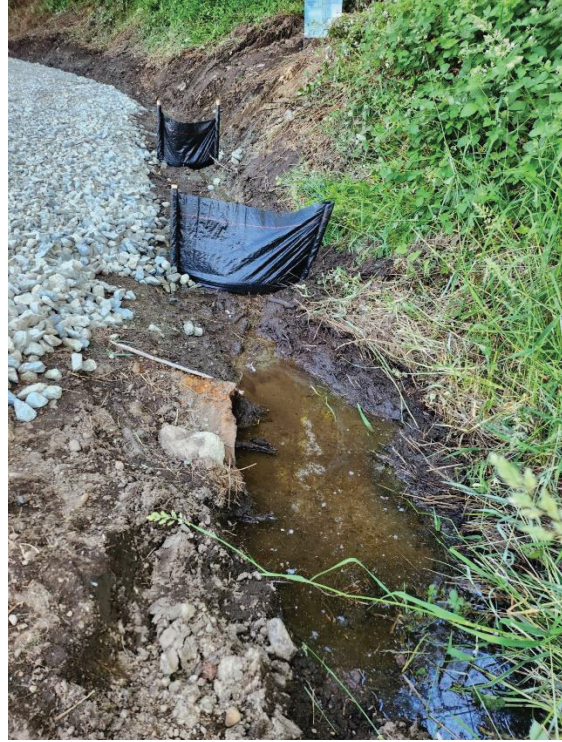
Silt fences functioning well, turbidity settling out
