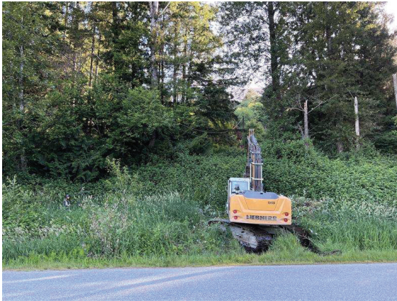
Figure 1 Excavator at the Entrance of Access Road
