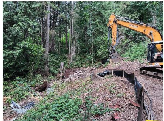
Figure 4 Excavator Placing Boulders to Creek's Bank
