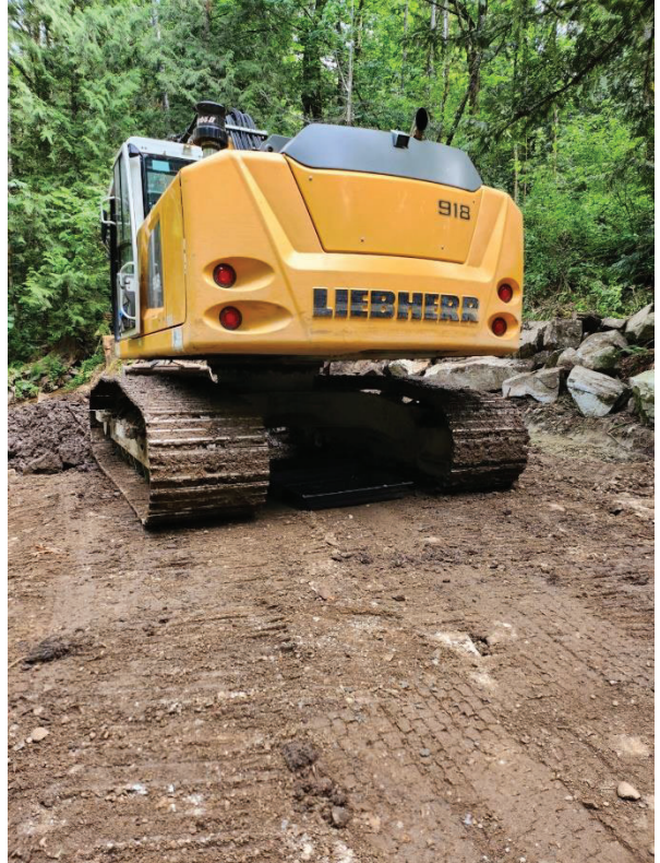
Boulder placement along North edge of bank
