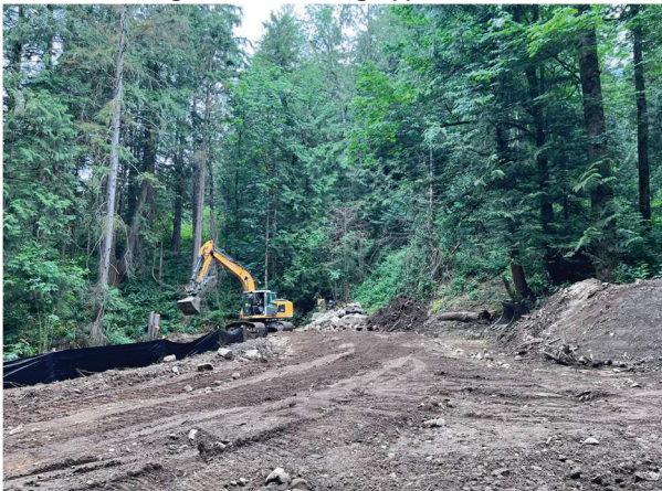
Figure 3 Removing Sediment from the Creek
