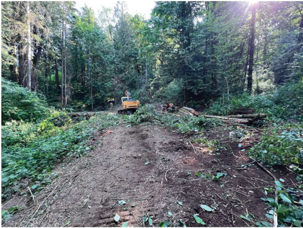
Figure 1 Stockpiling Logs and Stripping Topsoils
