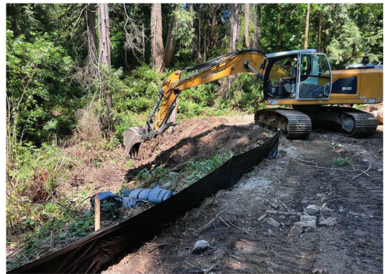
Figure 4 Clearing on the Creek
