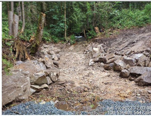
Photo 2. View of Davies Creek after armouring works have completed. (Jun. 19, 2023).
