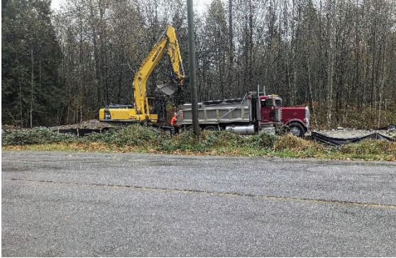
Figure - 3 Facing E – Loading contaminated soil offsite.
