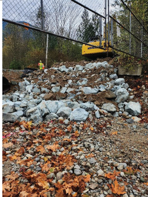
Figure 2 - Downstream Geo-Fabric/Armor around culvert complete
