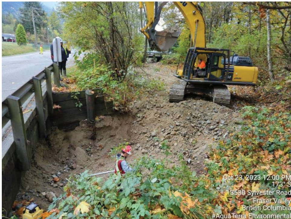
Photo 7: Excavating under Sylvester Road.
