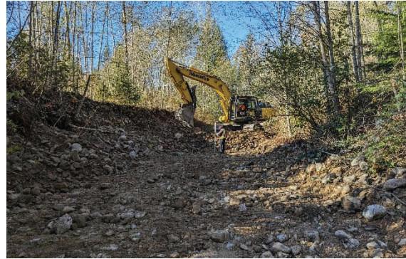
Figure - 4 Facing NW – Sediment removal near station 210.
