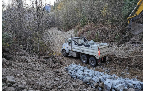
Figure - 2 Facing NE – Hauling rip-rap upstream to station 350.
