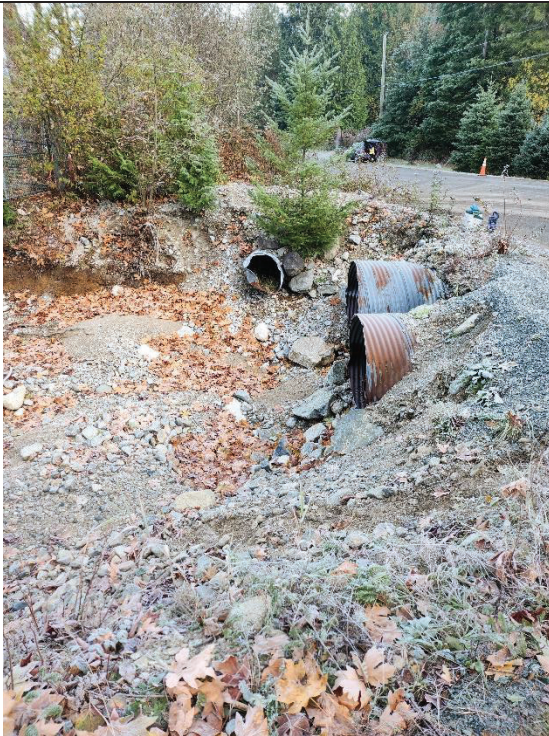
Figure 3 - Downstream culvert side before armor placement
