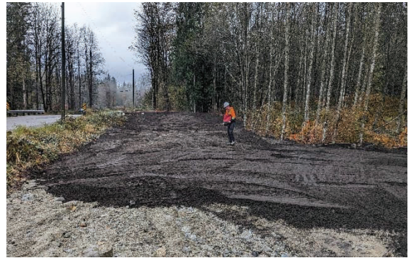
Figure - 2 Facing N – Seeding the Eng creek disturbed extents of the laydown area.
