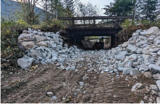
Figure - 1 Facing S – Finished rip-rap at the Hartley Rd bridge.
