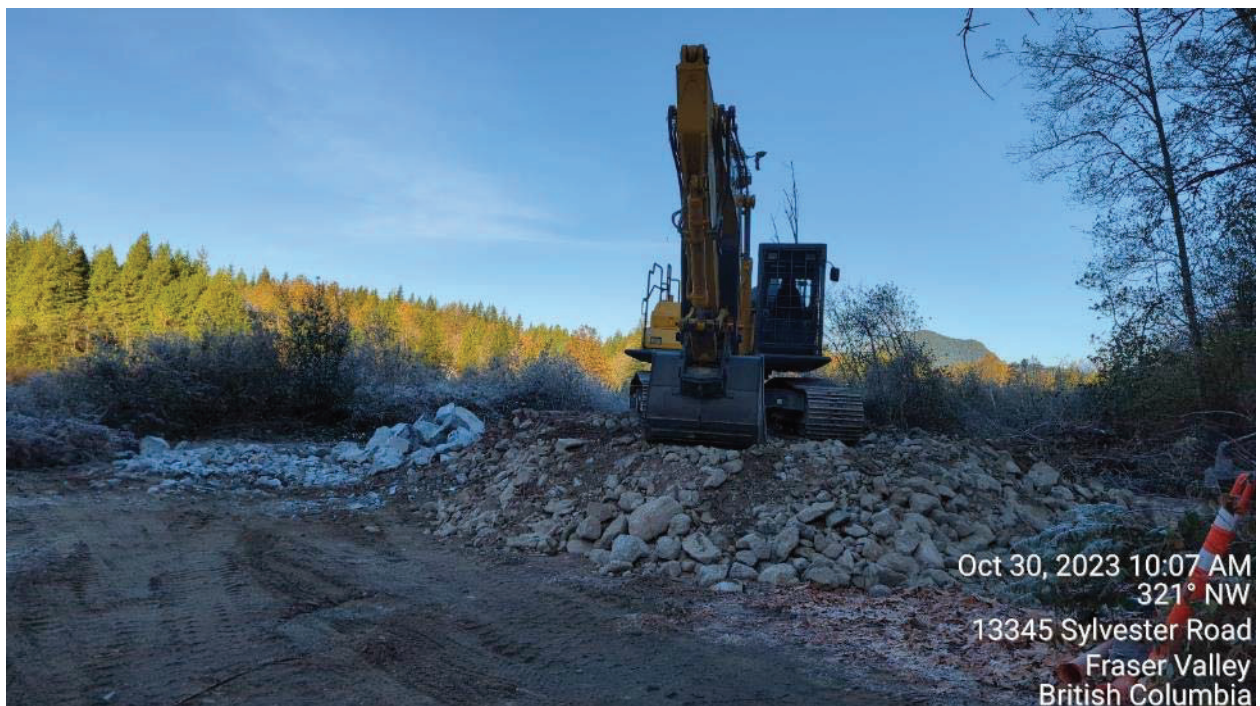
Photo 2: Laydown area with stockpile of riprap and creek gravel.
