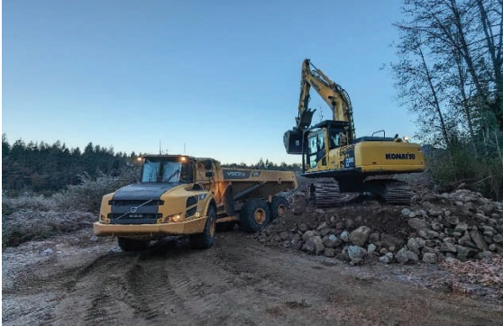
Figure - 1 Facing W – Hauling sediment to the laydown area next to Allan lake.
