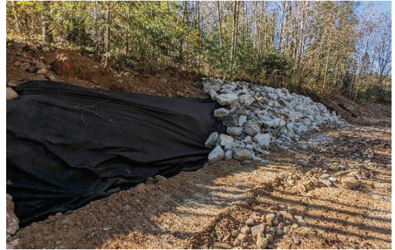
Figure - 4 Facing SW – Installing rip-rap at station 150.
