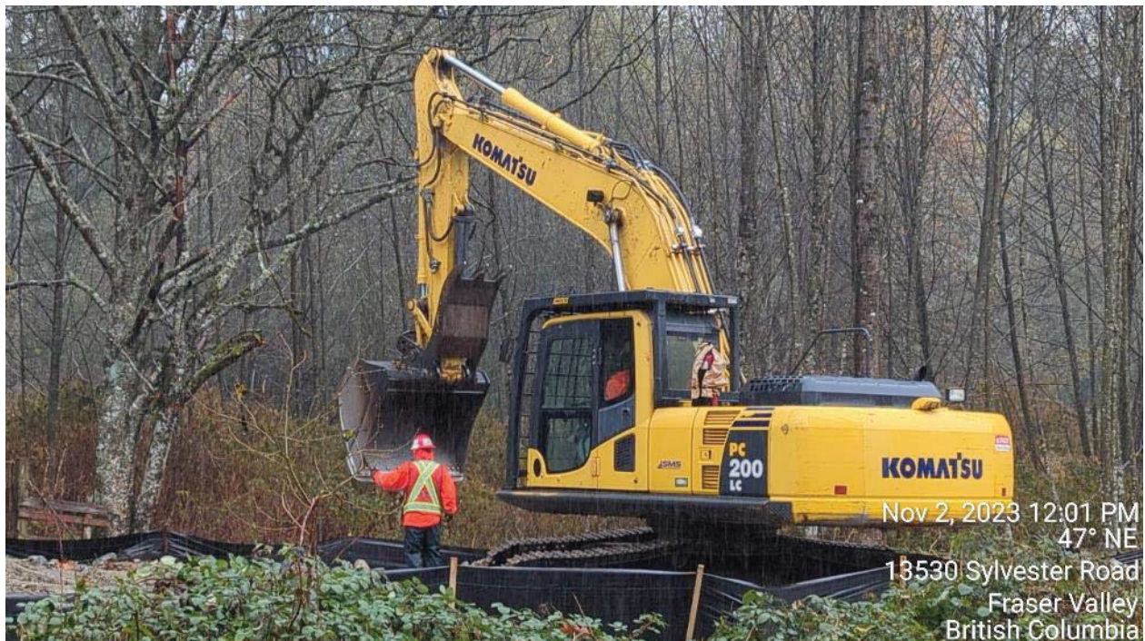
Photo 20: Crews cleaning the excavator bucket.
