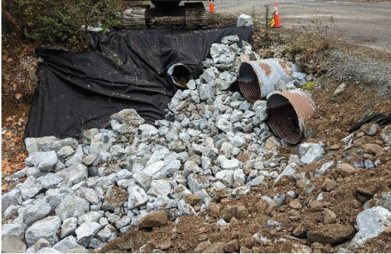
Figure - 3 Facing N – Installing rip-rap and filter fabric at the culvert outlet.
