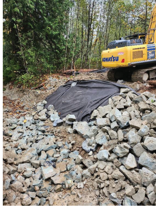
Figure 6 - Last of armoring before site ran out of rip-rap
