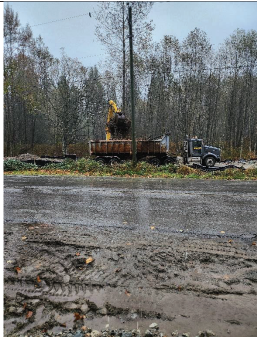
Figure 4 – Brush/woody debris loaded out from Eng Creek laydown yard
