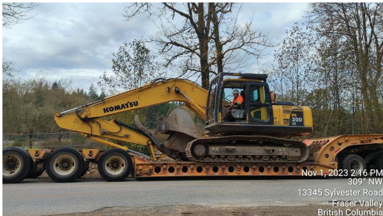
Photo 13: Transporting the excavator by flatbed to Eng Creek after cleaning.
