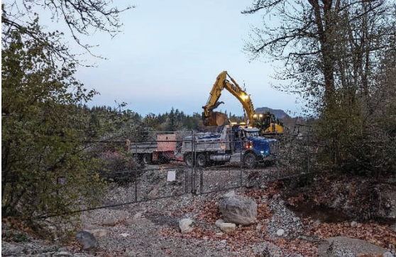
Figure - 1 Facing NW – Loading sediment from the laydown area.
