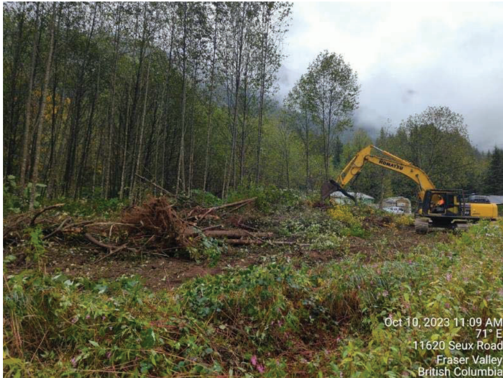
Photo 2: Removal of alders for the access road / laydown area (10 October).
