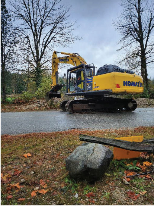
Figure 5 – 360 Ex. Removing excess material from berm
