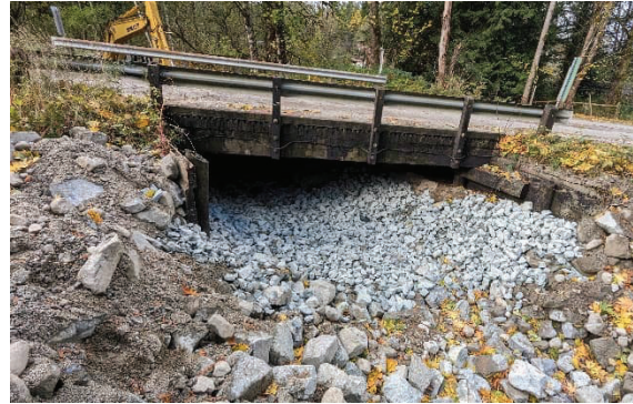
Figure - 4 Facing W – Finished rip-rap on the east side of the Sylvester road bridge.
