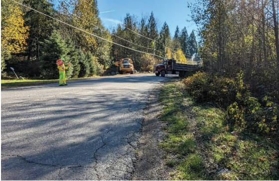
Figure - 3 Facing S – Hauling sediment from site. Flaggers controlling traffic.
