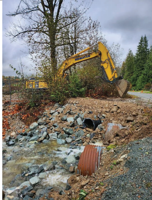
Figure 6 – 360 Ex. Removing excess material from berm
