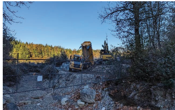
Figure - 2 Facing NW – Hauling sediment to the laydown area next to Allan lake.
