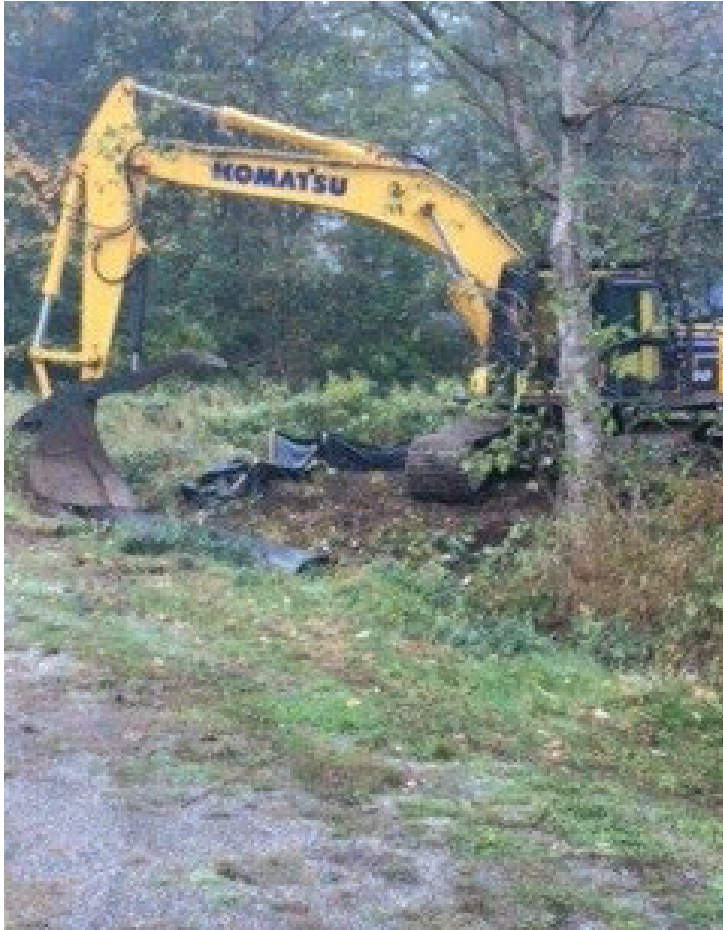
Figure 2 Installing temporary culvert at Hartley Rd. entrance to lay down.
