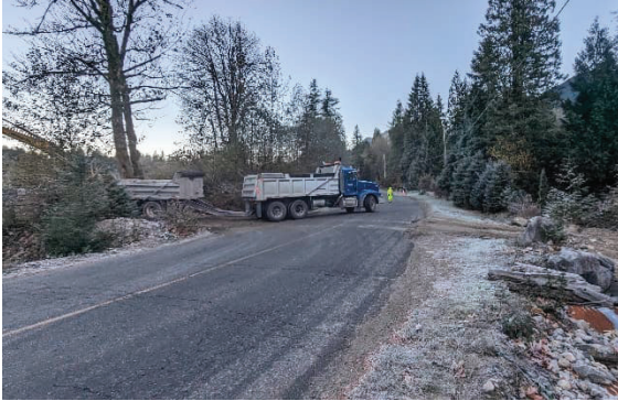
Figure - 3 Facing NW – Hauling sediment from site. Flaggers controlling traffic.
