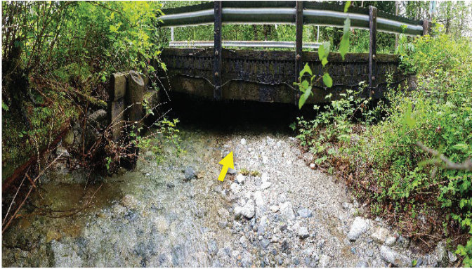
Eng Creek Upstream of Sylvester Road Bridge – Looking Downstream
