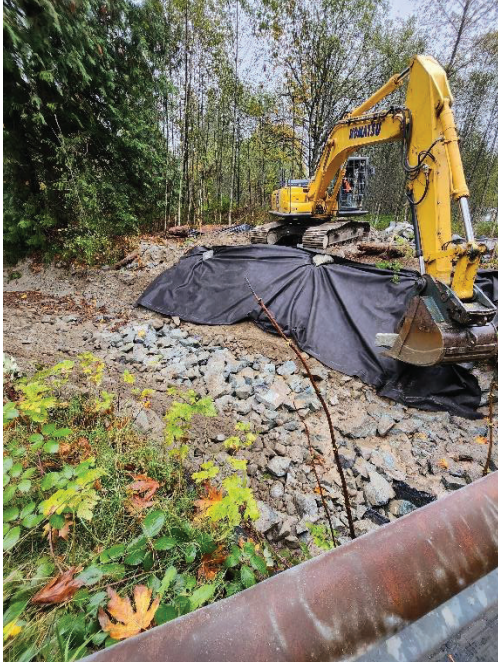
Figure 5 - Initial Geo Fabric/Rip-rap placement on NE bank
