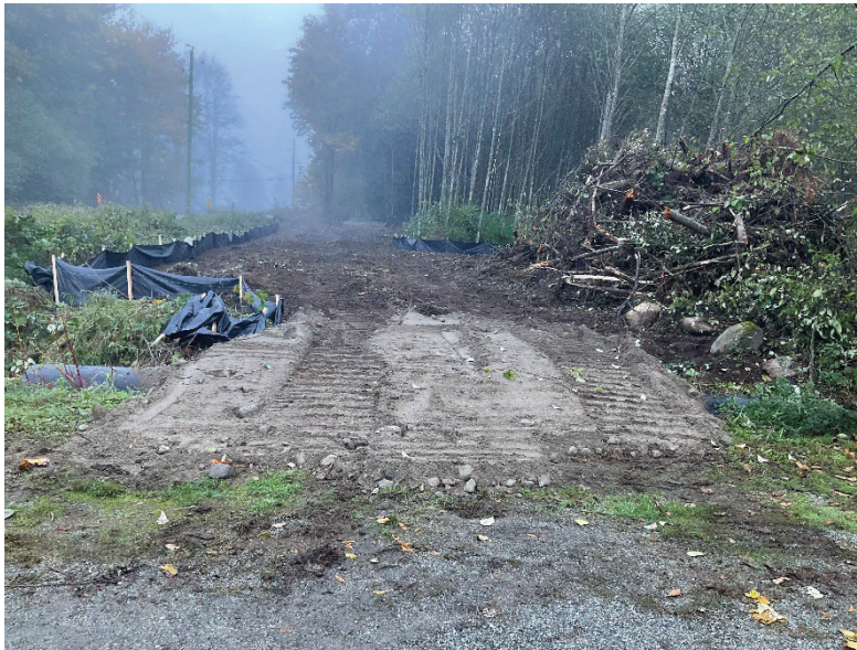
Figure 2 Beginning of Bedload as buffer pad in laydown are.
