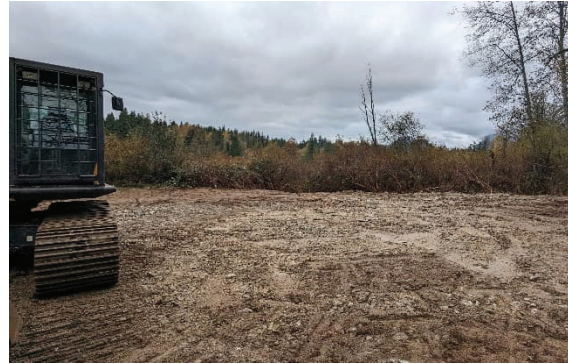
Figure - 4 Facing NW – McNab laydown stockpiles removed.
