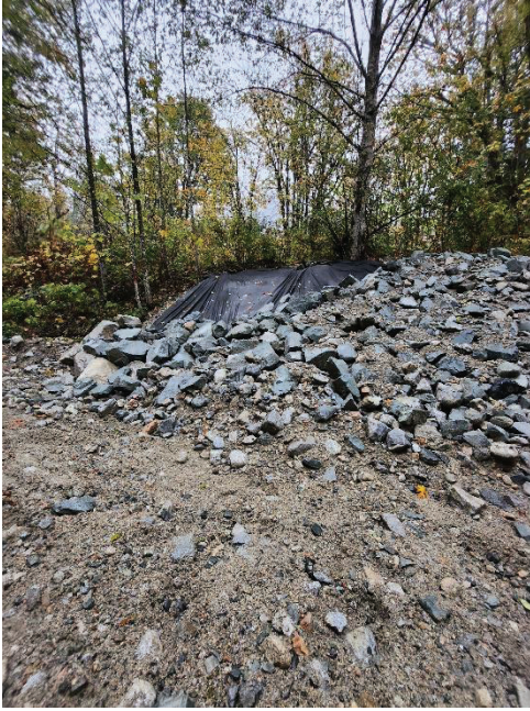
Figure 1 - Upstream bank-right fabric/rip-rap installation
