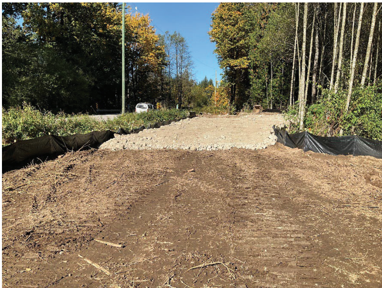
Figure 2 Beginning of Bedload as buffer pad in laydown are.
