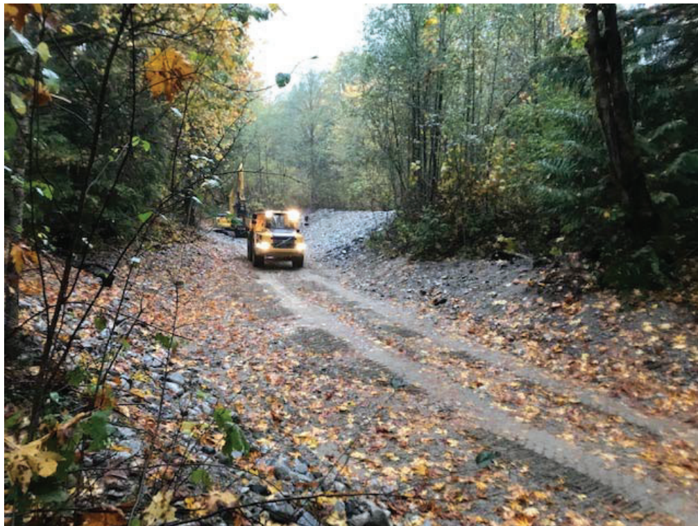
Photo 2: Overview of the work area / Eng Creek.
