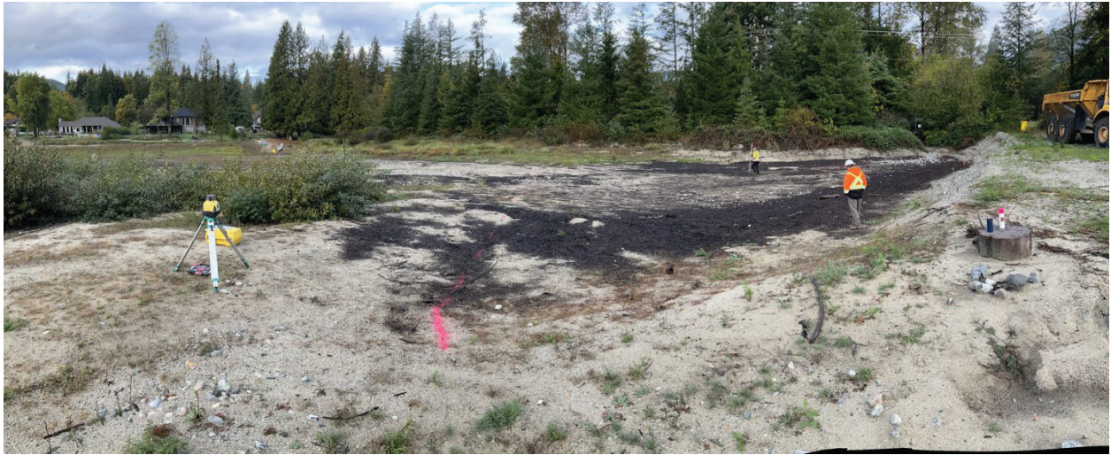
Figure 1 Prepping sediment removal at confluence of Eng creek and Allan Lake.
