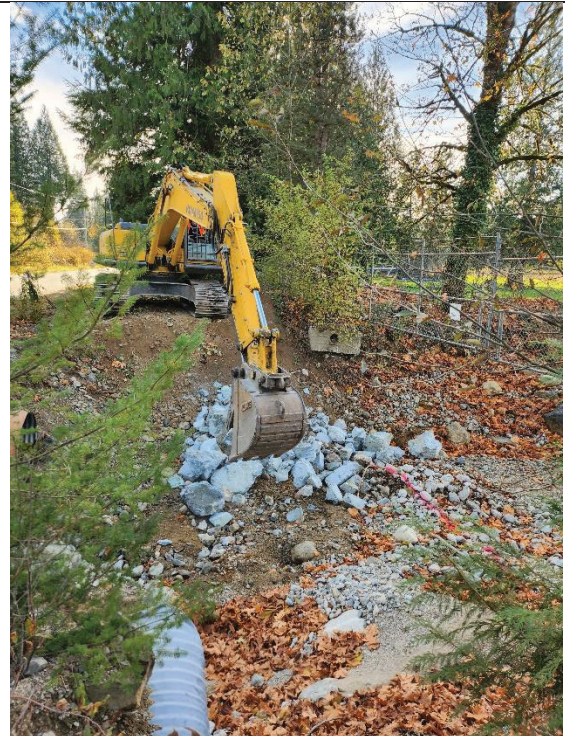
Figure 4 - Downstream culvert side after initial armor placement
