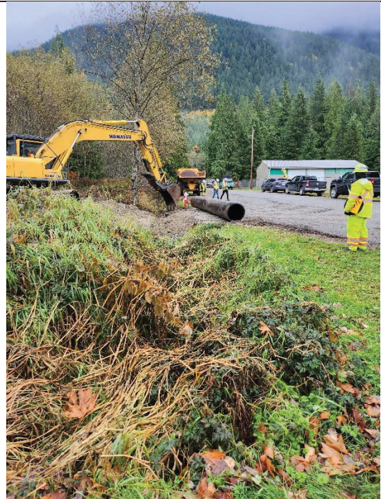
Figure 4 – Removal of temporary culvert
