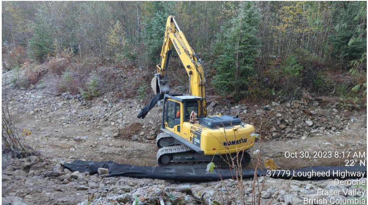
Photo 3: Laydown of geotextile fabric on the exposed bank.
