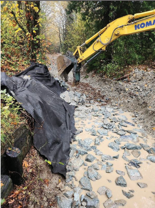
Figure 3 - Geo Fabric & rip-rap placement on NW bank above Sylvester Rd
