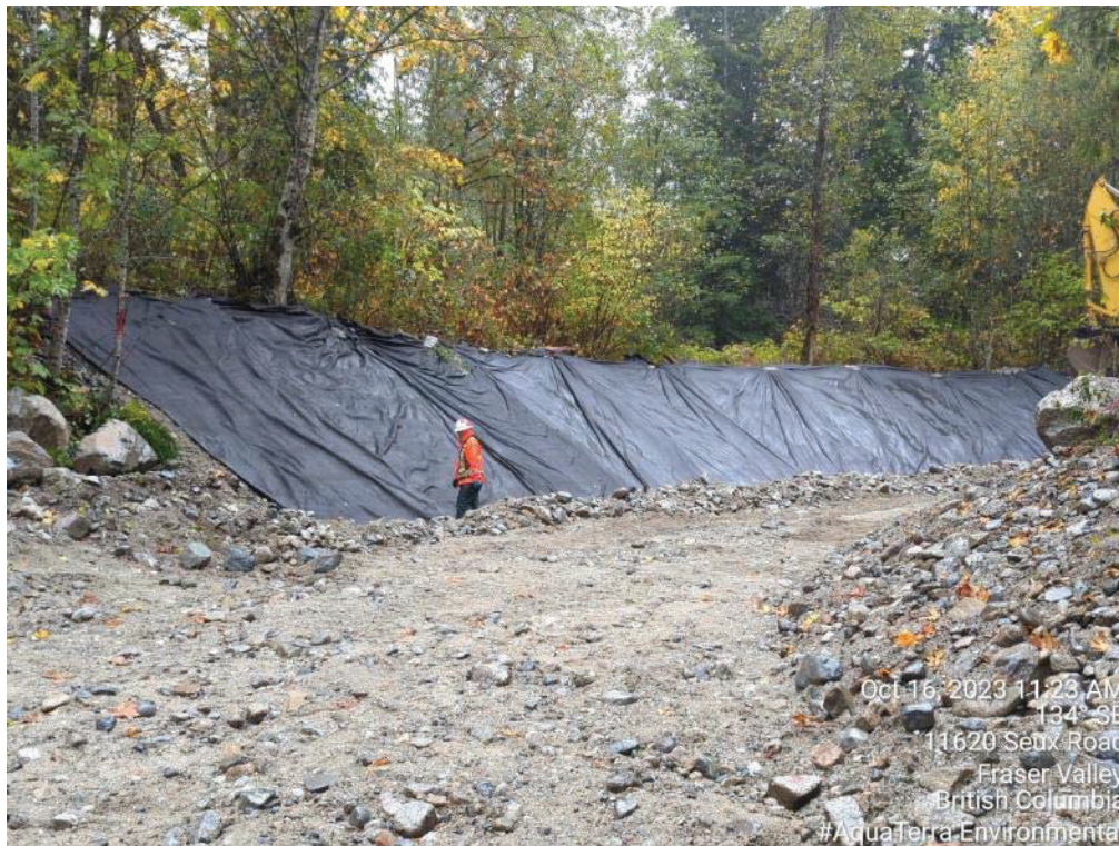
Photo 3: Textile fabric covering exposed bank slope.
