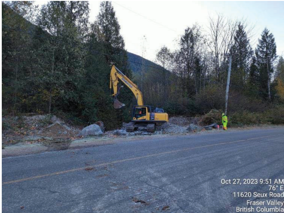
Photo 15: The excavator entering MacNab Creek.
