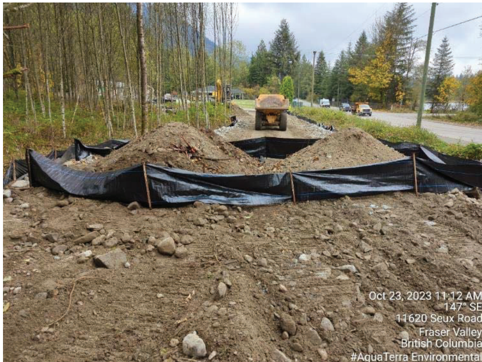
Photo 5: Excavated Japanese knotweed creek material stockpiled in laydown area.
