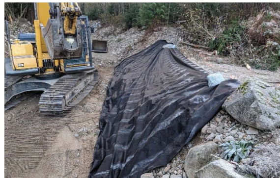
Figure - 2 Facing SE – Installing filter fabric along the banks near the culvert inlet.
