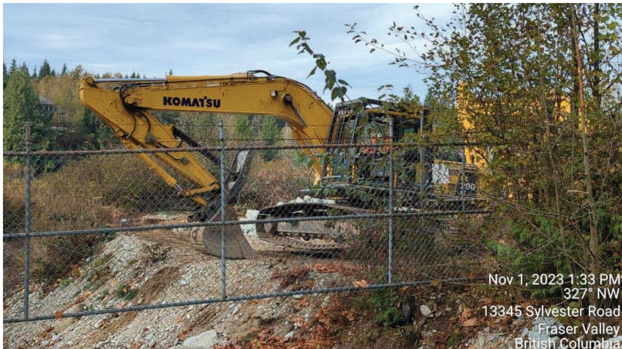
Photo 12: The excavator spinning its tracks to remove soil prior to transportation to the Eng Creek laydown area.
