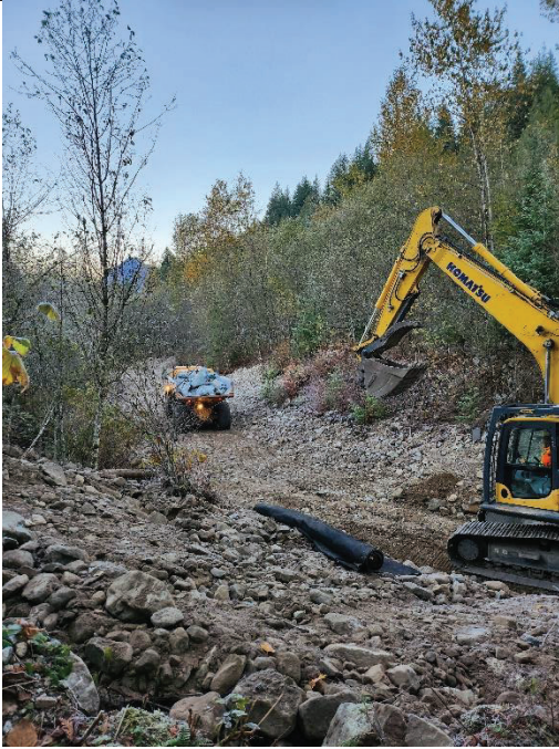
Figure 1 – Eastern bank of upper reach with Geo-Fabric/Armor
