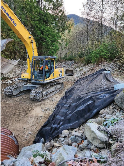
Figure 1 – Upstream Geo-Fabric/Armor around culvert
