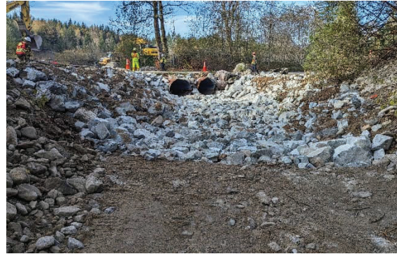
Figure - 4 Facing W – Finished rip-rap at culvert inlet.
