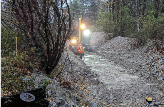
Figure - 1 Facing S – Removing excess sediment from Eng creek.
