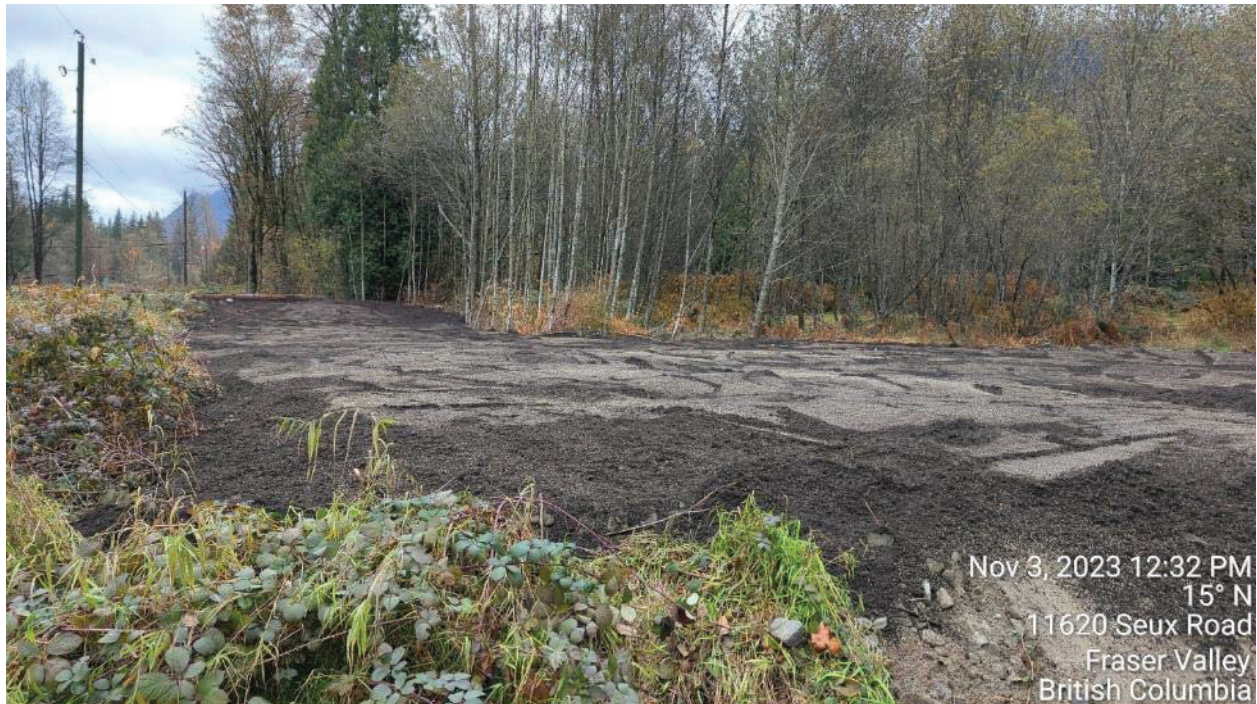
Photo 22: Eng Creek laydown area was capped with topsoil and seeded with a grass mix.
