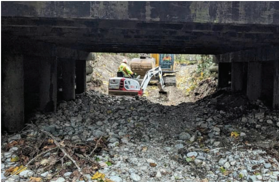
Figure - 1 Facing E – Placing rip-rap underneath the Sylvester road bridge.
