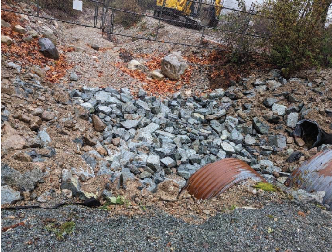
Photo 11: Completed work at the culvert outflow.
