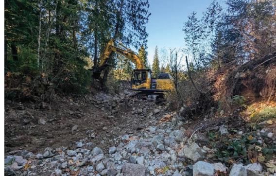
Figure - 2 Facing W – Sediment removal at station 0 350
