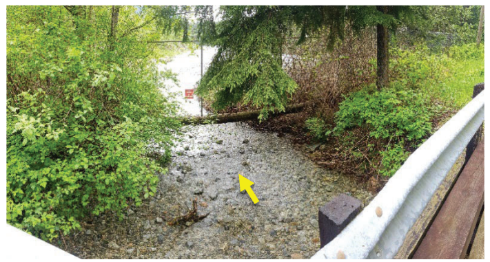
Eng Creek On Hartley Road Bridge – Looking Downstream
