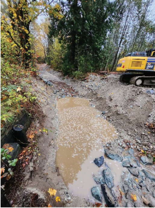
Figure 1 - Standing water with armor placement at creek bottom
