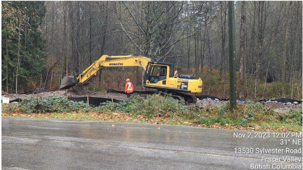
Photo 21: The excavator capping the stockpile area with clean creek gravel.
