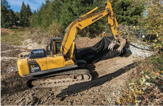
Figure - 3 Facing NW – Installing filter fabric at the Allen Lake inlet.
