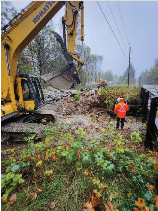
Figure 3 - Excavating bedload to creek level above Sylvester Rd Bridge
