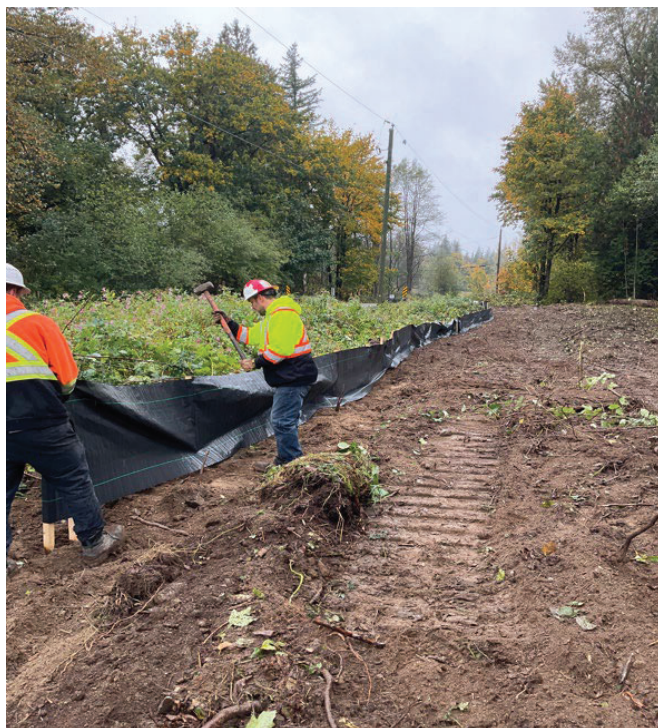
Figure 3 Installing isolation/sediment fence around laydown pad Hartley Rd./Eng Creek entrance.
