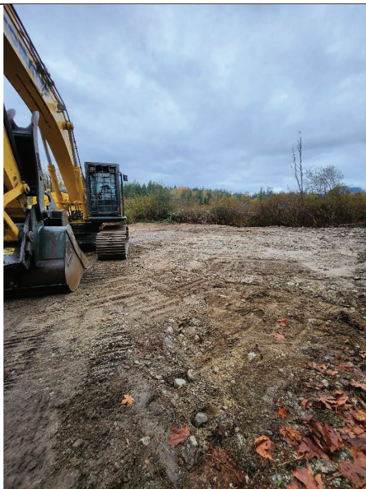
Figure 5 – 360 Ex. Removing leveling excess soil/gravel at McNab laydown area
