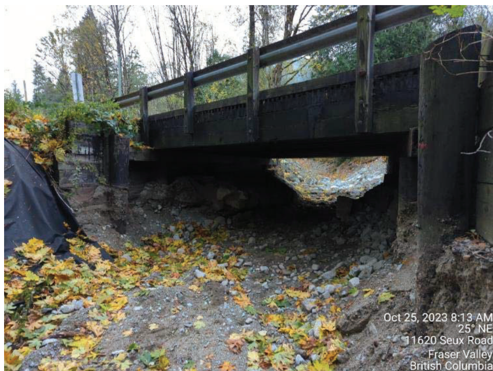
Photo 10: Excavation of Sylvester Road bridge.
