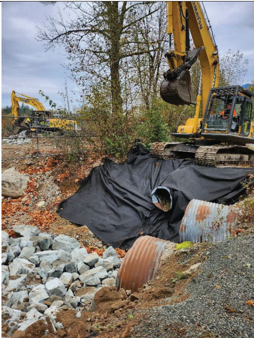
Figure 3 - Downstream culvert side before armor placement on west bank
