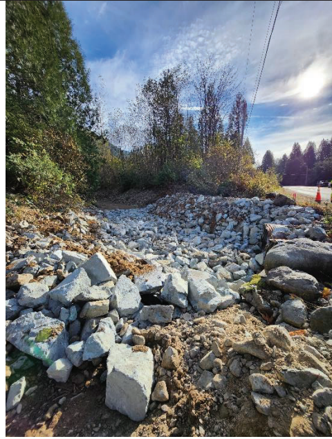
Figure 2 - Upstream Geo-Fabric/Armor around culvert complete
