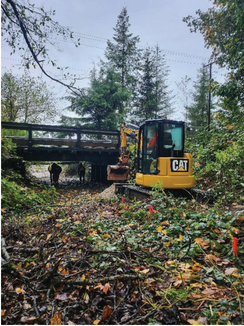
Figure 5 -Prep for middle section work between Sylvester & Hartley; Above Hartley Rd
