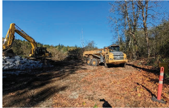
Figure - 4 Facing NW – Offloading creek sediment at the laydown.
