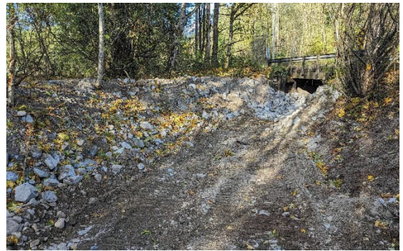
Figure - 2 Facing N – Finished rip-rap on the west side of the Sylvester road bridge.
