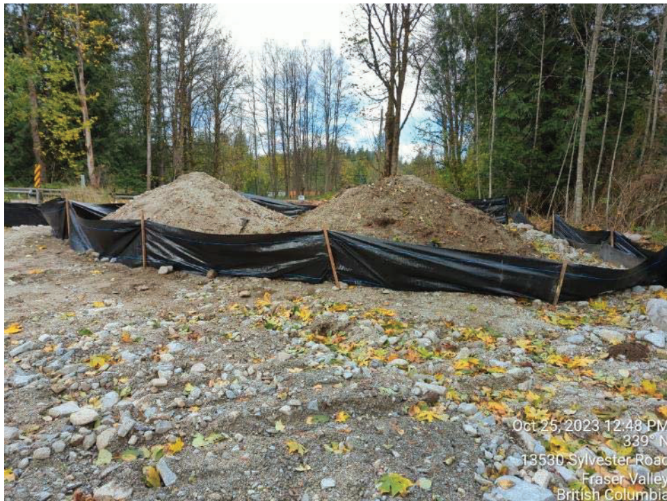
Photo 13: Stockpiles of Japanese knotweed infested material excavated from the creek.
