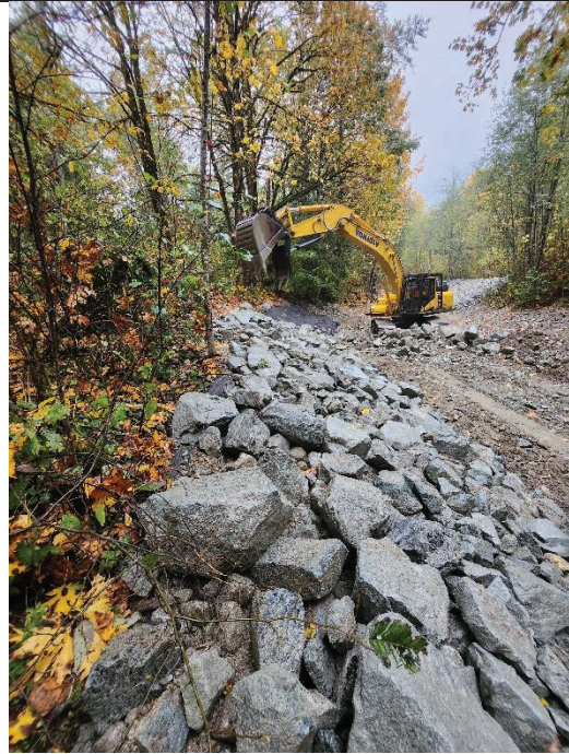
Figure 2 - Upstream bank-left fabric/rip-rap installation
