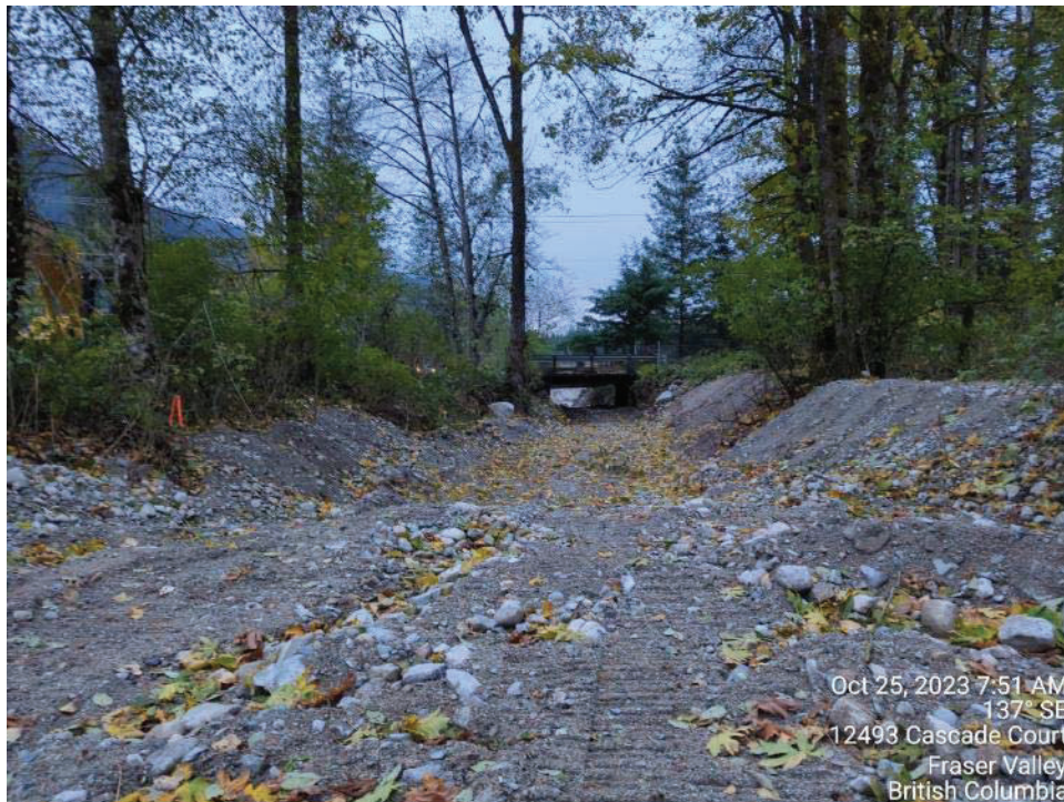
Photo 9: Excavated creek bed with Hartley Road bridge in the background.
