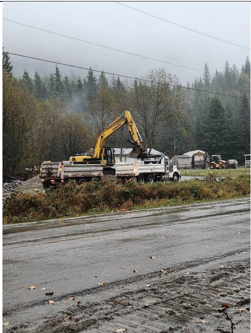
Figure 3 – Last of bedload loaded out from Eng Creek laydown yard
