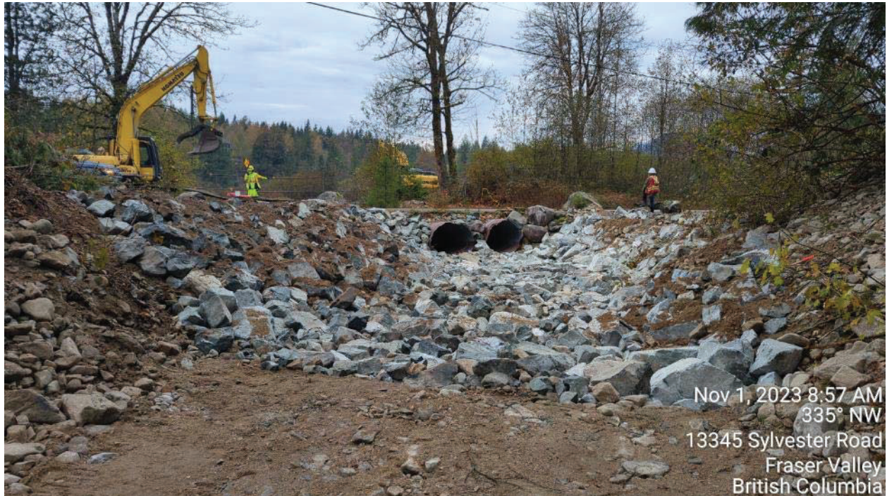
Photo 8: Completed work at the culvert intake.
