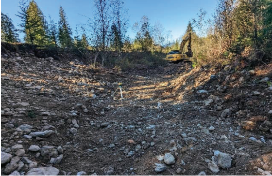
Figure - 3 Facing NW – Sediment removal near station 0+340
