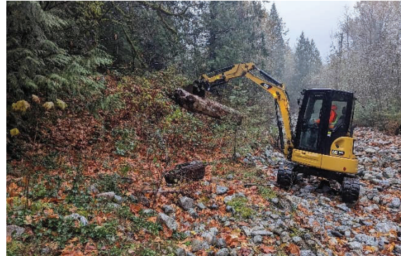
Figure - 2 Facing E – Removing a large from the Eng creek.
