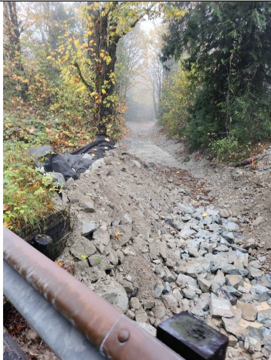
Figure 4 - Final armoring of NW bank
