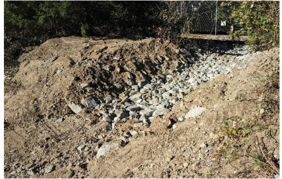
Figure - 4 Facing NW – Finished rip-rap at the Allen Lake inlet.
