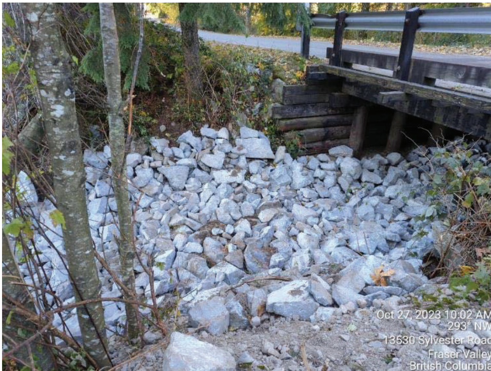
Photo 18: Riprap installed at the outflow of Eng Creek on the southside of Hartley.
