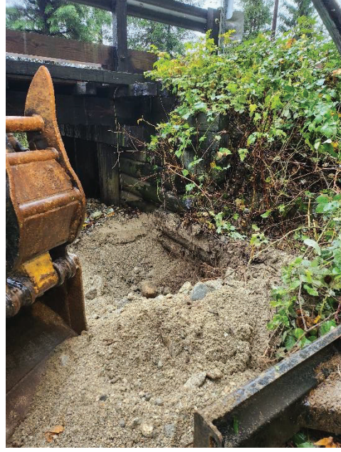
Figure 6 - Test dig of bedload to find depth of bridge mooring
