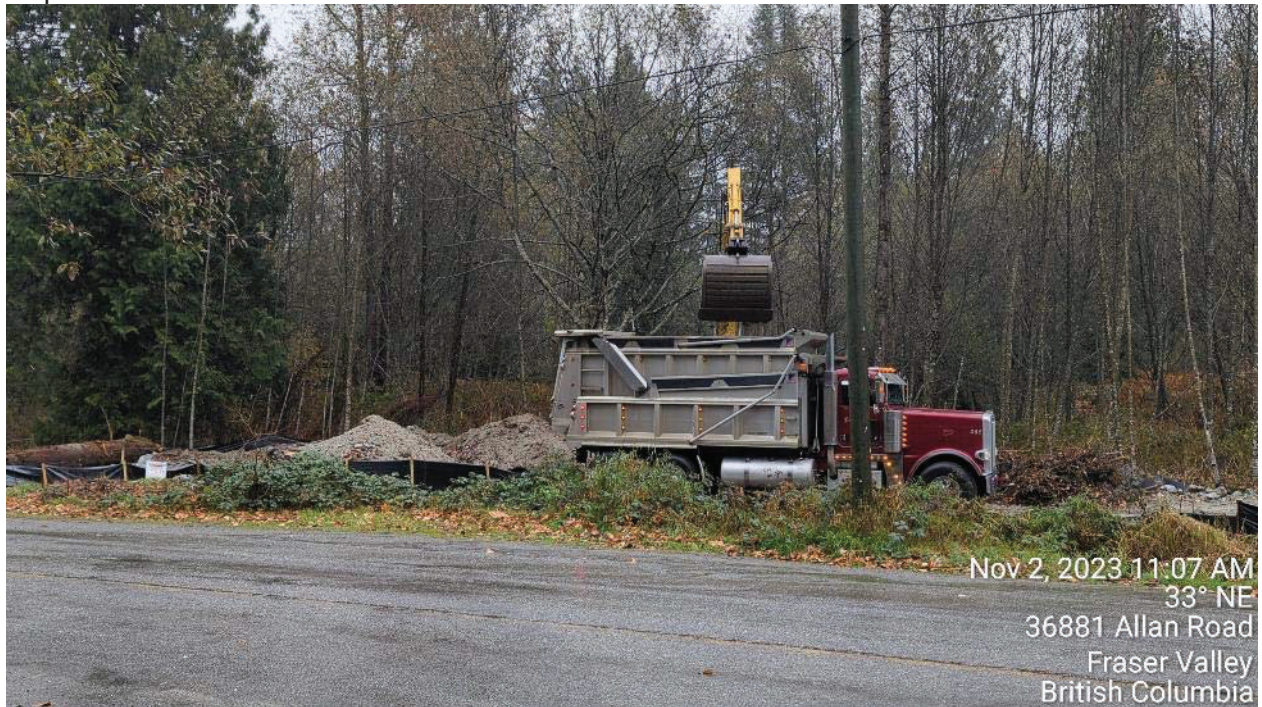
Photo 17: Japanese knotweed infested material loaded into BC Earth Exchange truck for offsite disposal.
