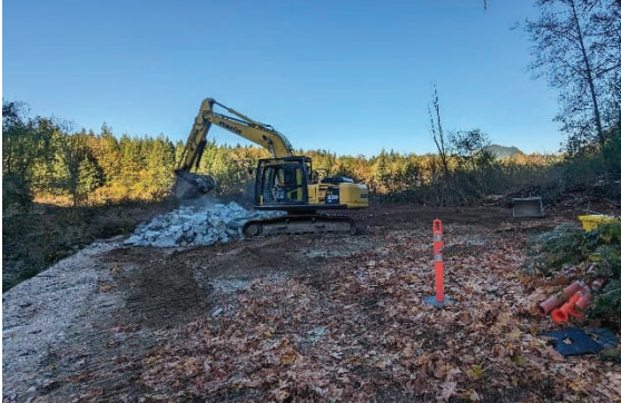
Figure - 1 Facing W – Establishing the laydown area.
