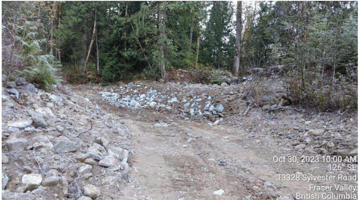
Photo 5: Completed riprap installation work.
