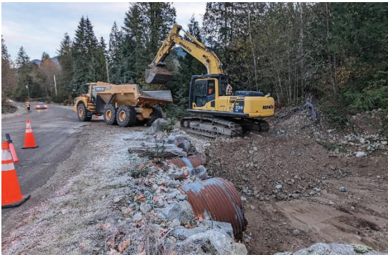
Figure - 1 Facing N – Removing the last of the sediment from McNab creek.
