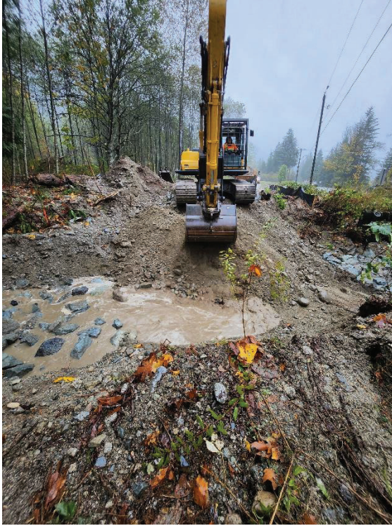
Figure 5 - Instream work area becoming wetted
