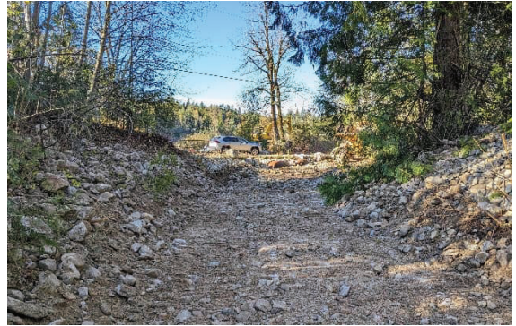
Figure - 4 Facing W – Sediment removed up to the Sylveser Rd culverts.
