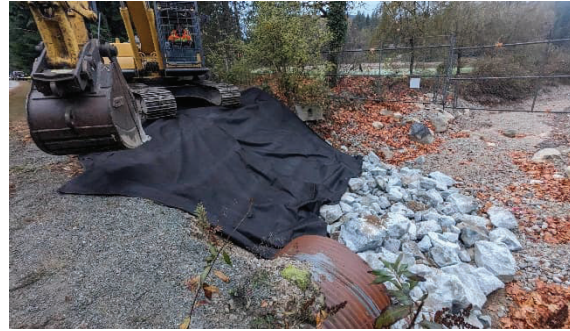
Figure - 2 Facing SW – Installing filter fabric along the banks near the culvert outlet.
