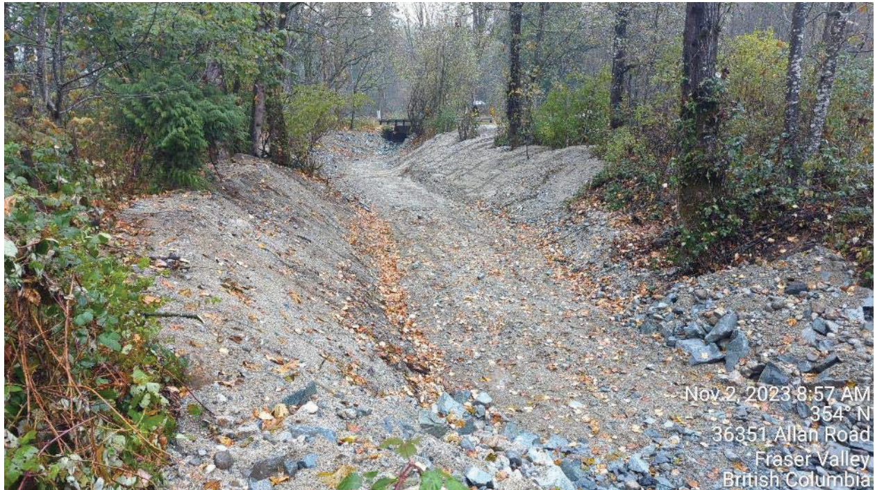
Photo 15: Regrading of the creek complete.
