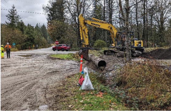
Figure - 3 Facing W – Removing access ramp and temporary culvert from the Eng Creek laydown area.
