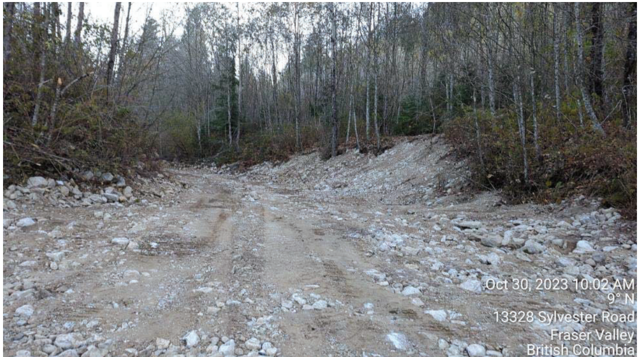
Photo 1: Excavation of MacNab Creek.
