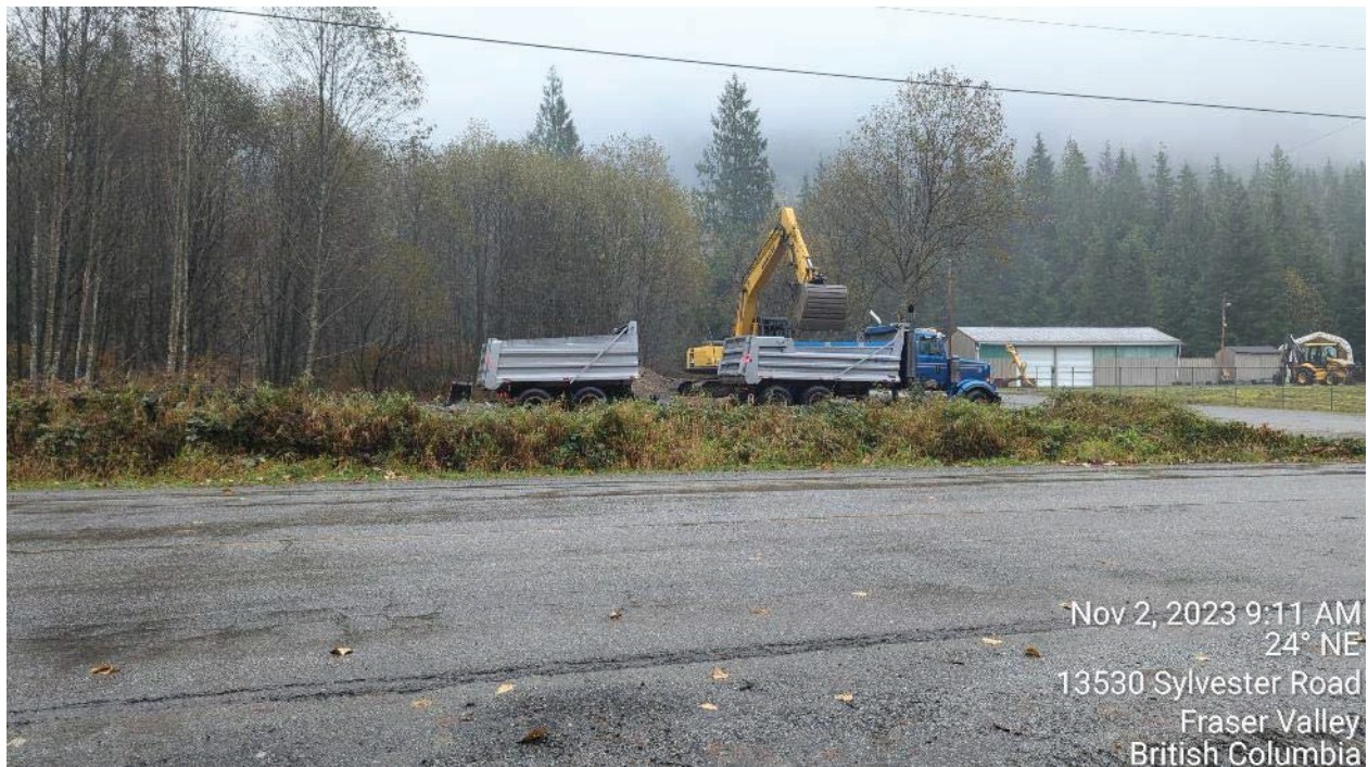
Photo 16: Gravel trucks removing creek gravel from site.
