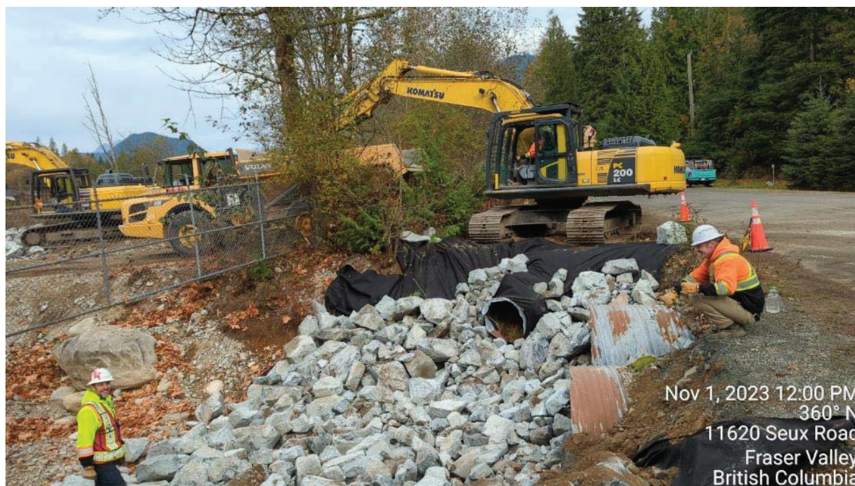
Photo 10: Installation of riprap over the geotextile material in progress.
