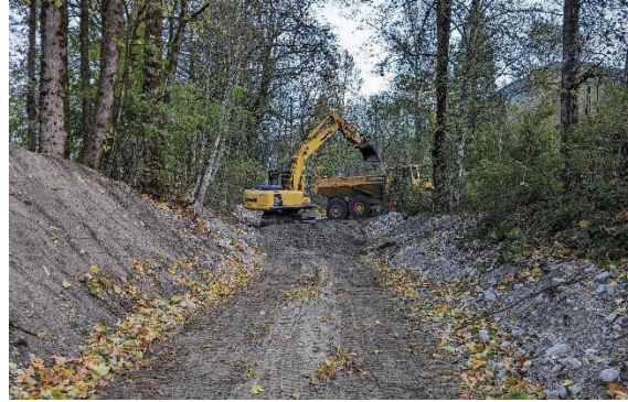
Figure - 2 Facing N – Removing remaining sediment from between the 2 bridges.
