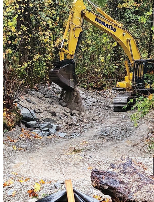
Figure 2 - Finishing of first rip-rap placement
