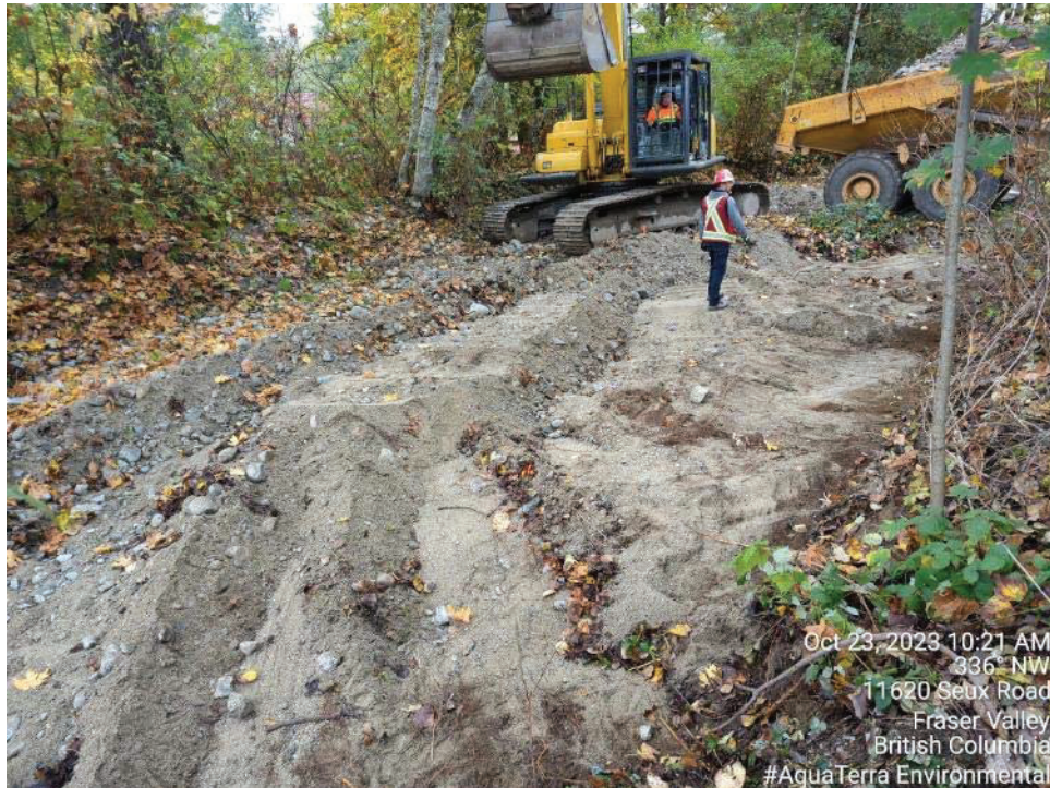
Photo 4: Japanese knotweed being excavated from the creek bed.
