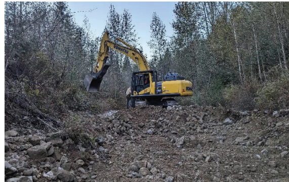
Figure - 2 Facing N – Sediment removal near station 310
