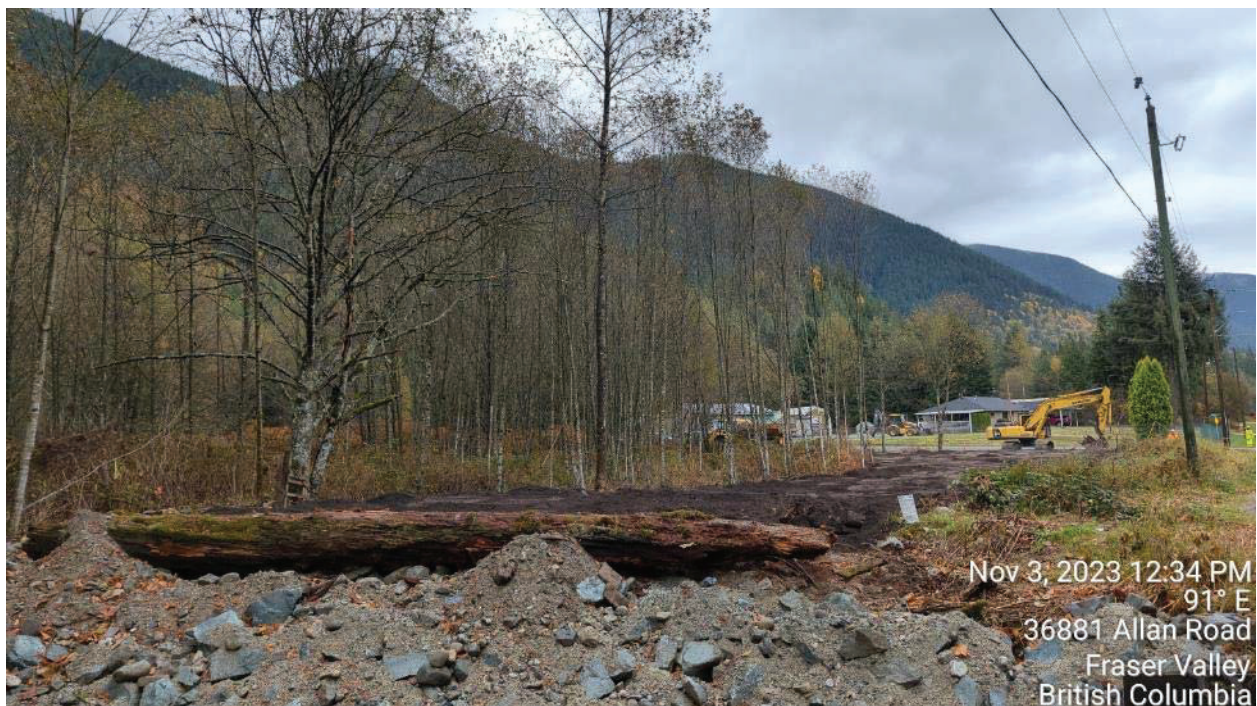
Photo 23: Laydown area facing south.
