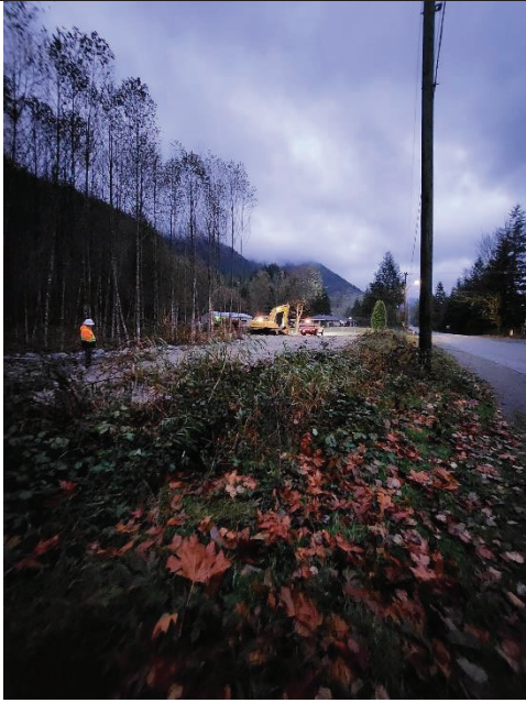
Figure 1 – Topsoil delivery at Eng laydown area
