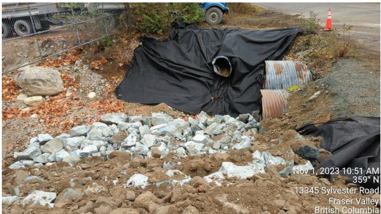
Photo 9: Geotextile fabric laid down on the exposed northwest bank of the culvert outflow.
