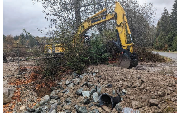
Figure - 4 Facing N – Removing excess material at McNab culvert outlets.
