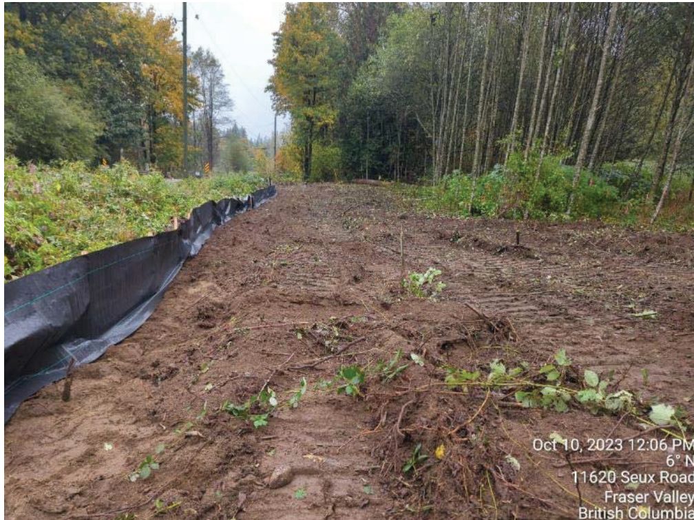
Photo 4: Vegetation removed from the access road / laydown area.
