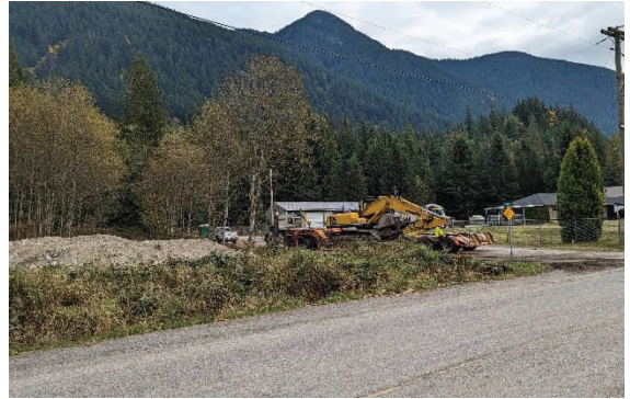
Figure - 4 Facing E – Mobilized equipment back to Eng Creek laydown.
