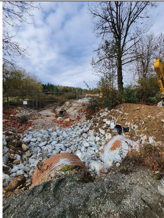
Figure 4 - Downstream culvert side after initial armor placement west bank complete
