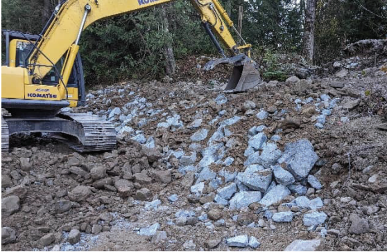
Figure - 3 Facing SE – Installing rip-rap at station 350.
