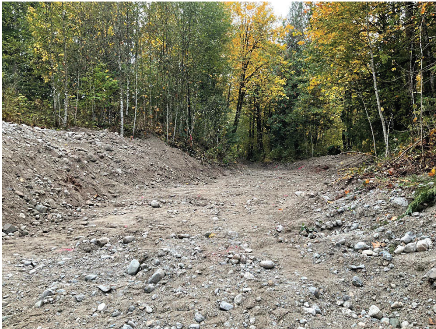
Figure 4 Looking down stream at banks prepped for riprap on Monday.
