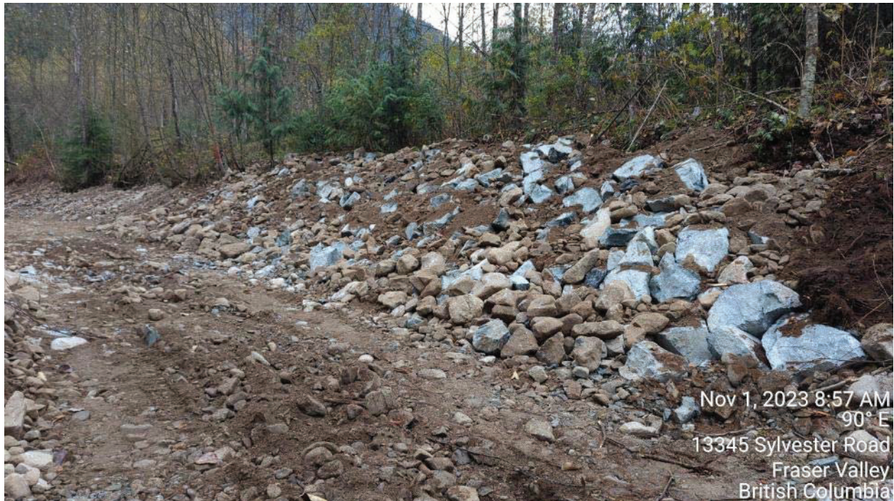
Photo 7: Completed riprap installation at MacNab Creek.
