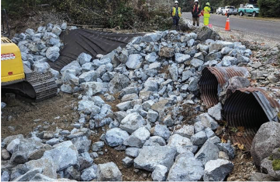
Figure - 3 Facing S – Installing rip-rap at the culvert inlet.
