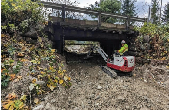
Figure - 3 Facing S – Removing sediment from under the Hartley road bridge.
