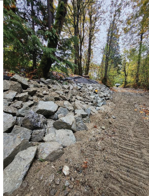
Figure 4 - Lower section bank-right fabric/rip-rap installation
