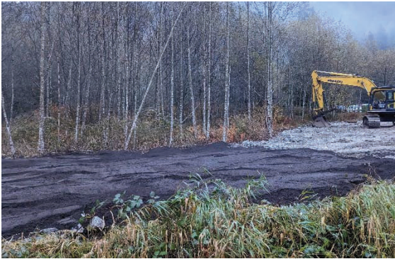
Figure - 1 Facing SE – Topsoiling Eng Creek laydown area.
