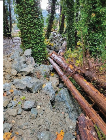
Photo 2 Completed riprap bank armouring along relic side channel
