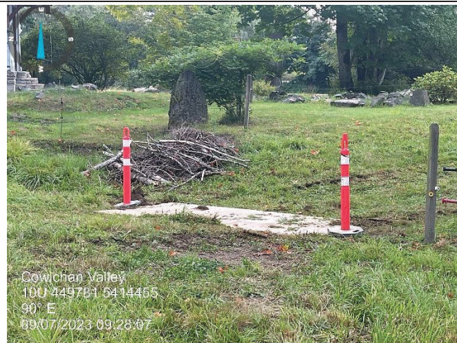
Photo 3: Steel plates placed over irrigation line at request of property owner
