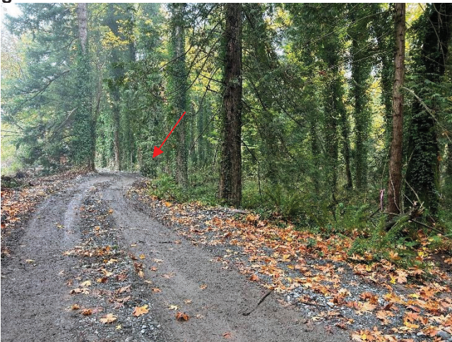
Photo 3: Potential location for riprap (aprox Chainage 0+340)
