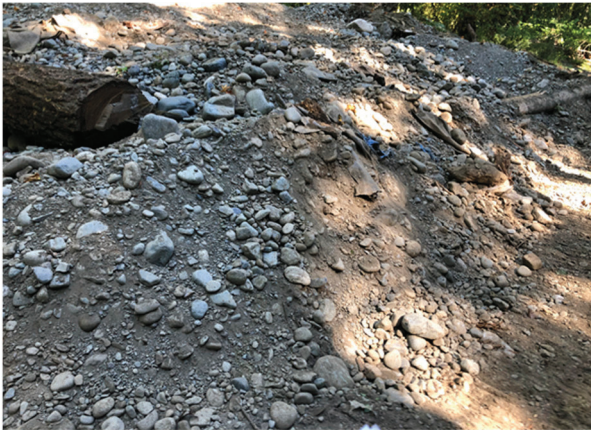
Photo 9: Berm constructed within Halat FN across the relic floodplain side channels on right bank of Chemainus River
