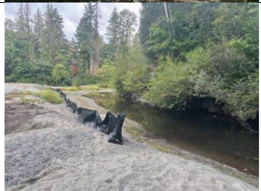
Photo 8 Installation of silt fencing as directed by KWL Environmen tal monitor. 2023-09-08
