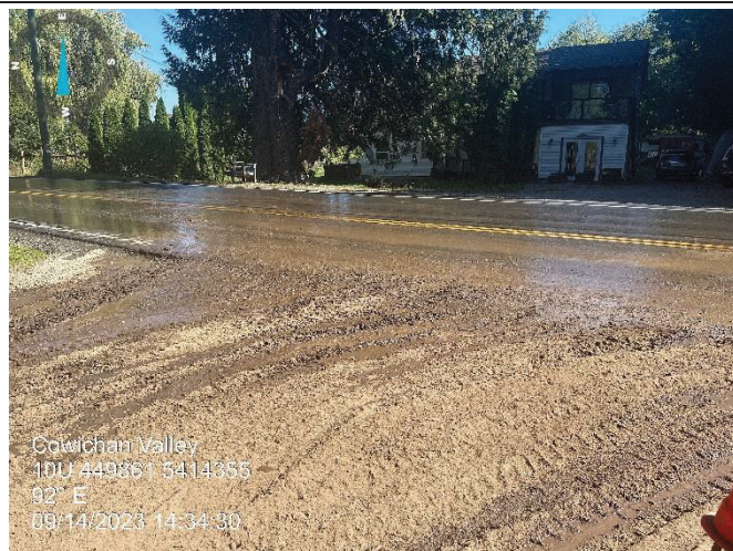
Photo 5: Chemainus Road after water truck had come
