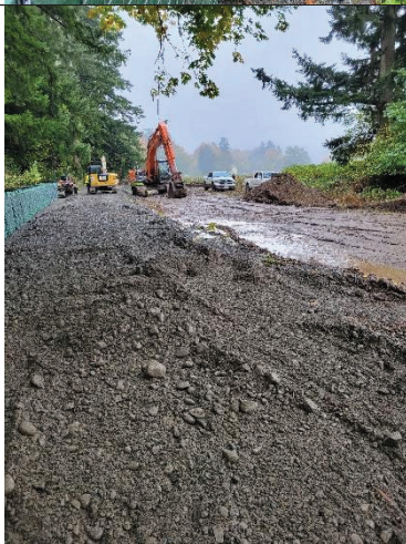
Photo 5 Material being removed to narrow access road and restore farm property
