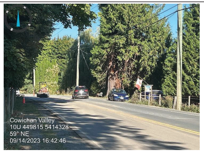
Photo 8: Road being cleaned at end of shift
