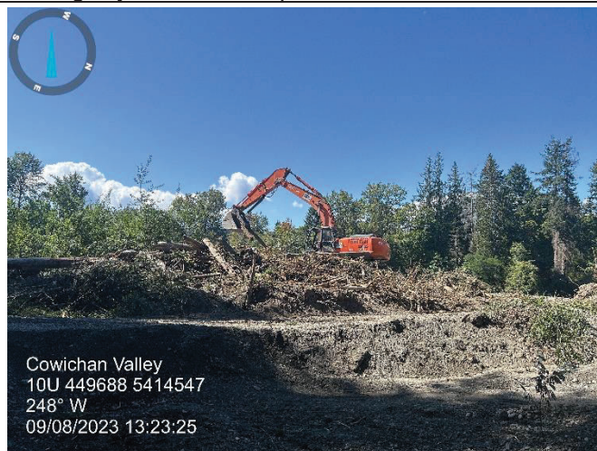
Photo 5: Excavator sorting large woody debris from clearing brush
