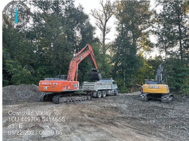
Photo 1: Final sediment being removed
