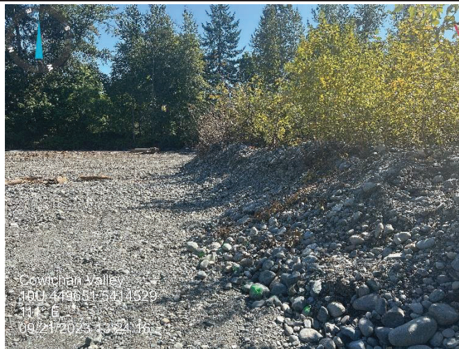
Photo 3: Transition between gravel bar and excavated area before sloping
