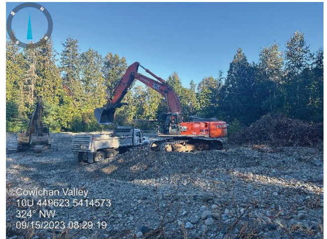
Photo 2: Gravel being removed off-site
