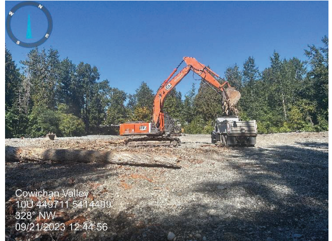
Photo 2: Large logs being removed off-site
