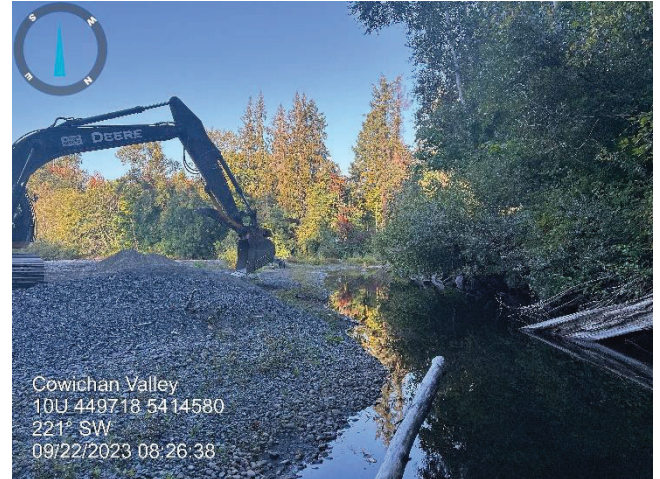
Photo 2: Amphibian fencing removed and smoothing of slopes
