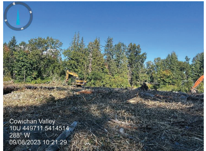
Photo 2: Grubbed gravel bar
