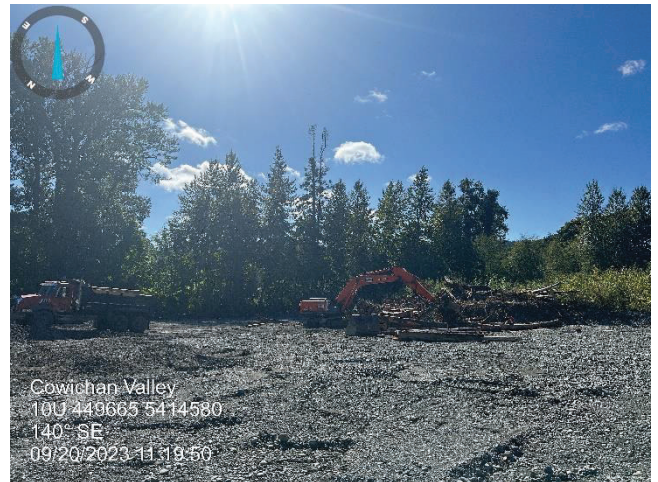
Photo 2: Large logs being removed off-site
