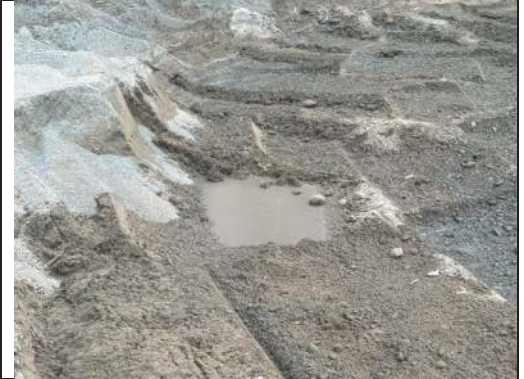
Photo 4 Groundwater infiltration from overexcavation of silt. 2023-09-11
