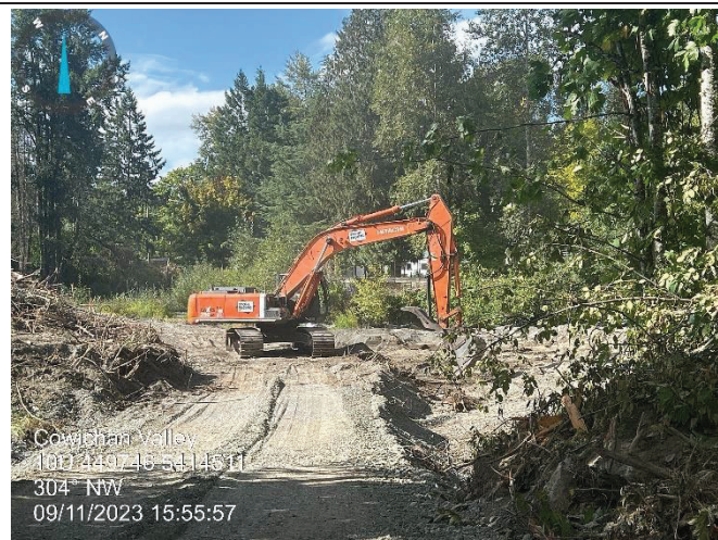
Photo 5: Fine material pile removed
