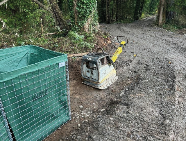
Photo 1: End of constructed HECO baskets at chainage 0+220. Note excavation into original ground.
