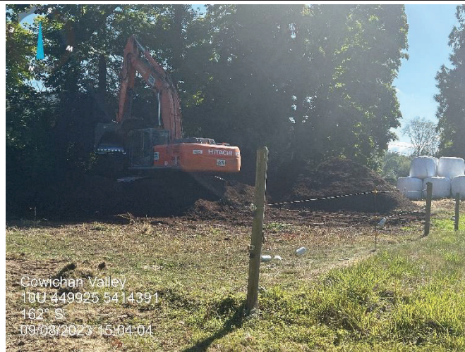
Photo 7: Excavator prepping property owner's determined area for fine material placement
