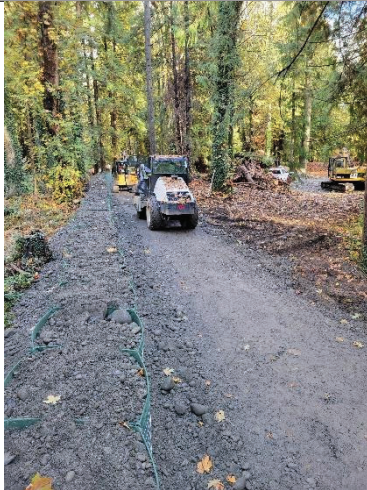
Photo 3 Barrier extent as of November 2, 2023
