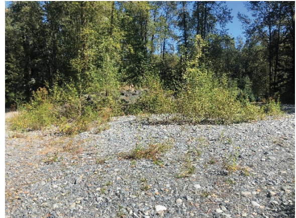
Photo 4: DNC Water Supply Well Head Protected by Riprap Adjacent to Side Channel
