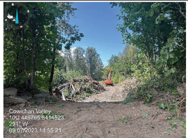
Photo 4: Construction access progressing
