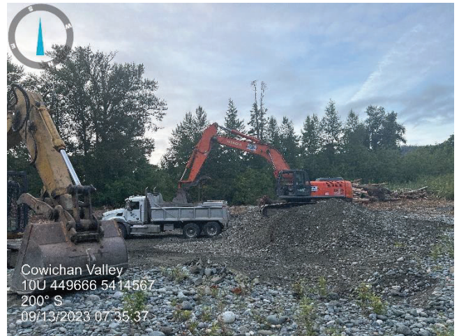
Photo 2: Gravel being removed off-site
