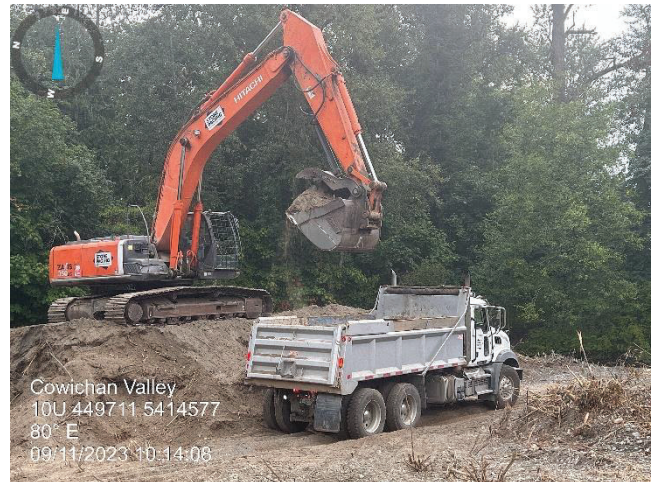
Photo 2: Fine material stockpile being removed
