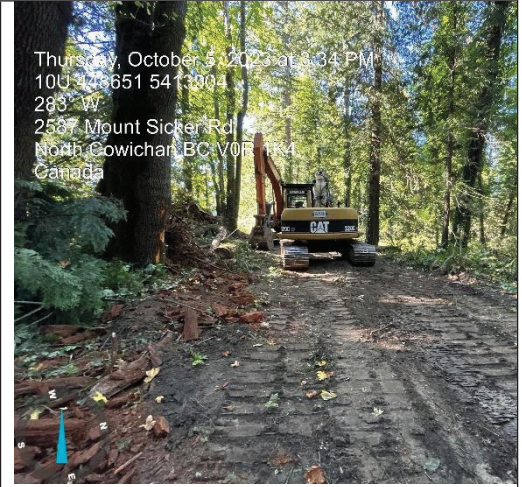
Photo 2 Excavator clearing along barrier alignment
