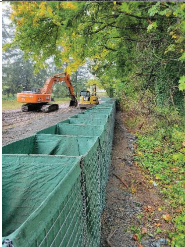
Photo 3 Hesco baskets placed and ready for filling
