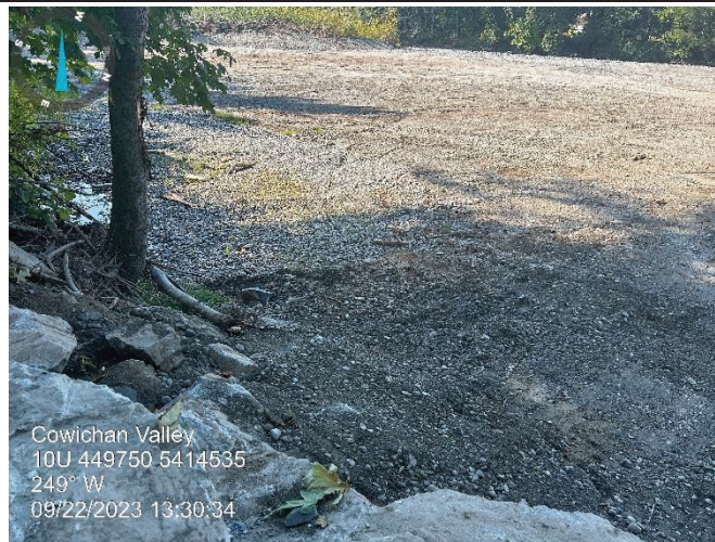
Photo 3: Access ramp removed
