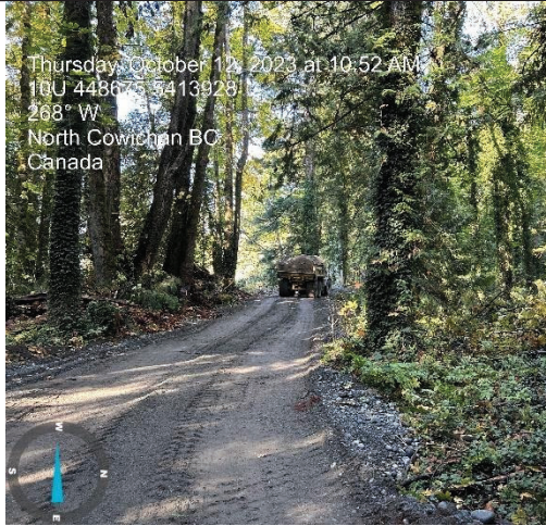
Photo 2 Alignment cleared and grubbed before base material placement near upstream terminus at Highway 1.
