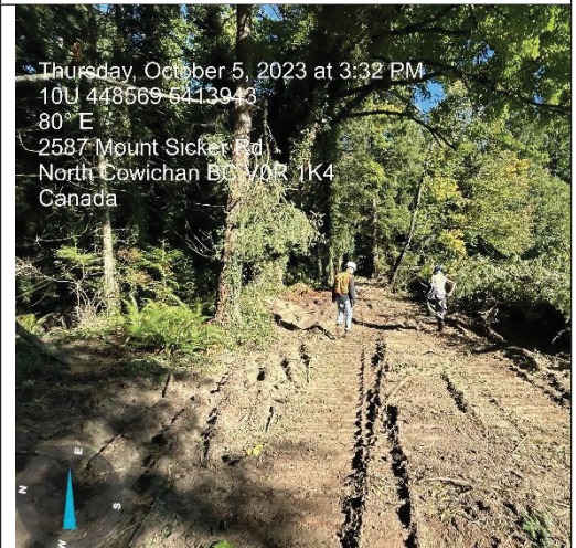
Photo 4 Completed alignment stripping and grubbing on Russell Farms property
