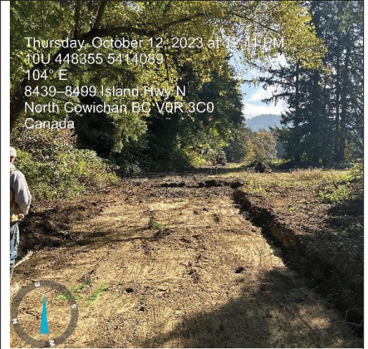
Photo 2 Alignment cleared and grubbed before base material placement near upstream terminus at Highway 1.
