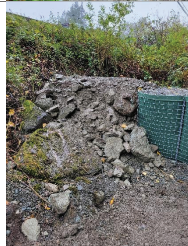
Photo 4 Upstream terminus where barrier ties into Highway 1 embankment
