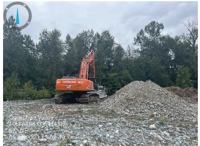
Photo 2: Gravel being removed off-site
