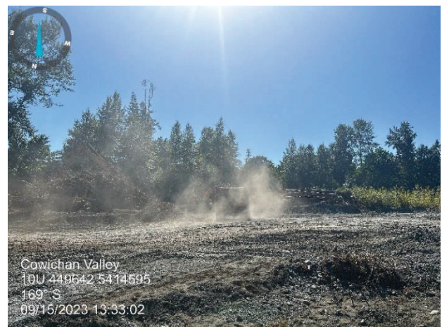
Photo 2: Dust on gravel bar
