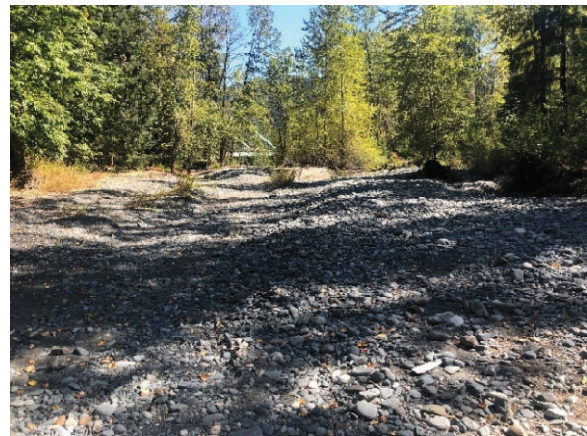
Photo 2: Sediment Accumulated Inside Channel on Right Bank of Chemainus River Note Highway 1 Bridge in background
