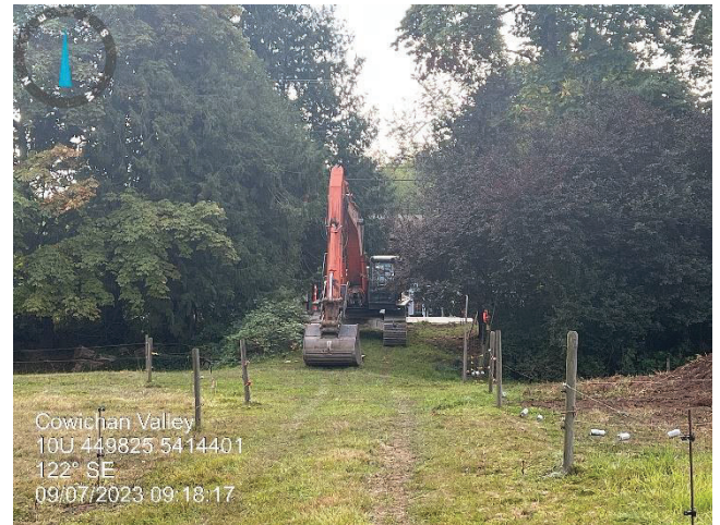
Photo 2: Constructing access to gravel bar
