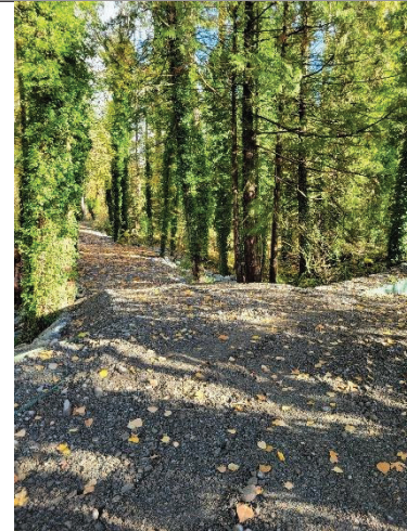
Photo 4 Completed access ramp
