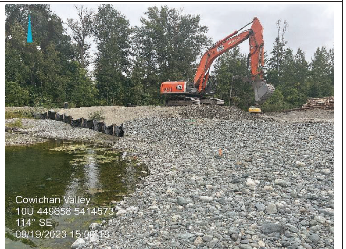
Photo 4: Removal of sediment berm
