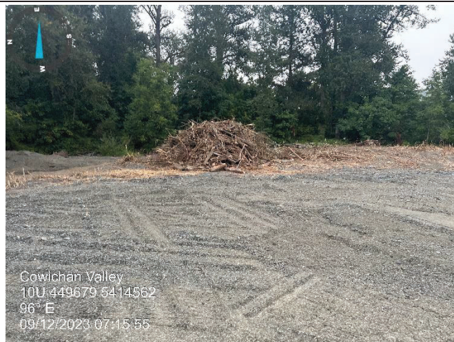
Photo 3: Brush pile to be removed off-site
