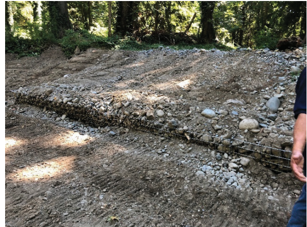
Photo 10: Opening Through the Berm for Smaller Right Bank Side Channel
