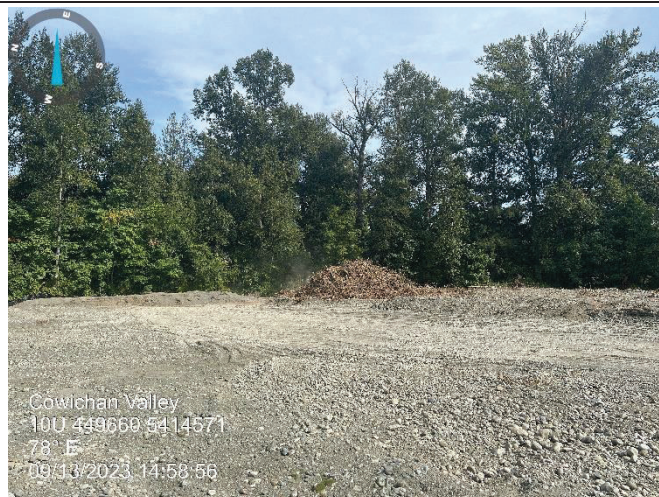
Photo 3: Brush pile to be removed off-site
