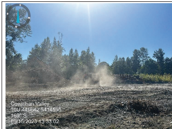
Photo 7: Dust on gravel bar
