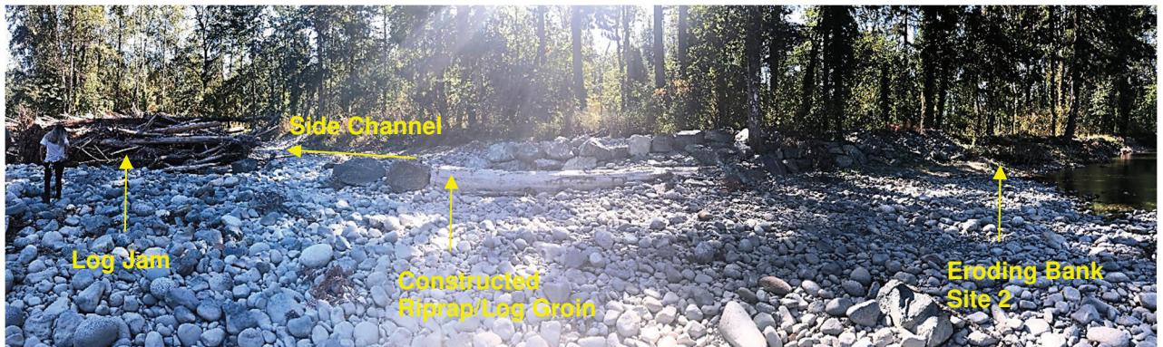
Photo 8: Entrance to Right Bank Side Channel Showing Eroding Bank, Riprap/Log Groin, and Log Jam
