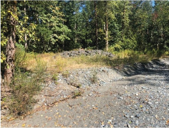
Photo 3: DNC Water Supply Well Head Protected by Riprap Adjacent to Side Channel
