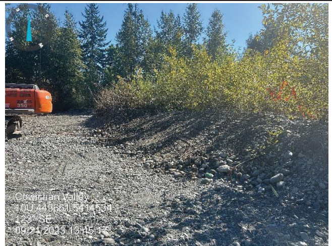
Photo 4: Transition between gravel bar and excavated area at 2:1 slope
