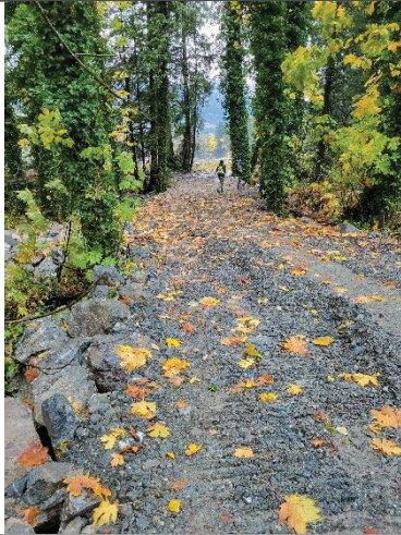
Photo 1 Completed riprap floodplain berm
