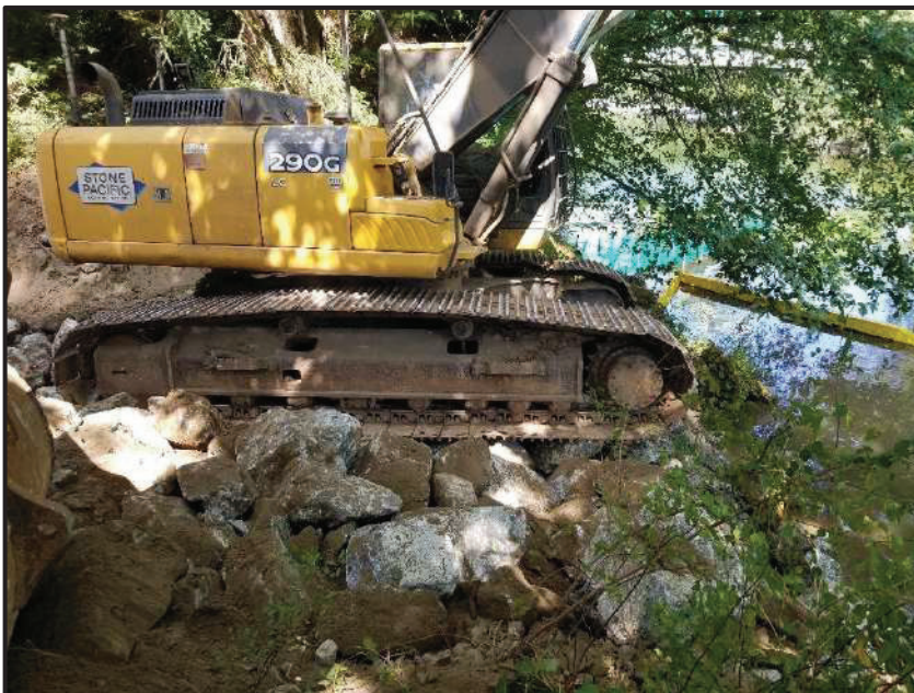
EXCAVATOR ATOP THE RIPRAP OF WEIR 1. THE KEYED IN RIPRAP WAS USED TO PROVIDE A STABLE WORKING PLATFORM DURING THE EXCAVATION PROCESS.
