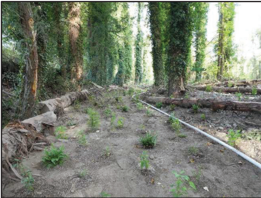
LOOKING WEST ALONG A FULLY REPLANTED SECTION OF THE ROAD. AFTER THE PLANTS WERE PUT IN, GRASS SEED WAS APPLIED OVER THE SOIL TO REDUCE EROSION.
