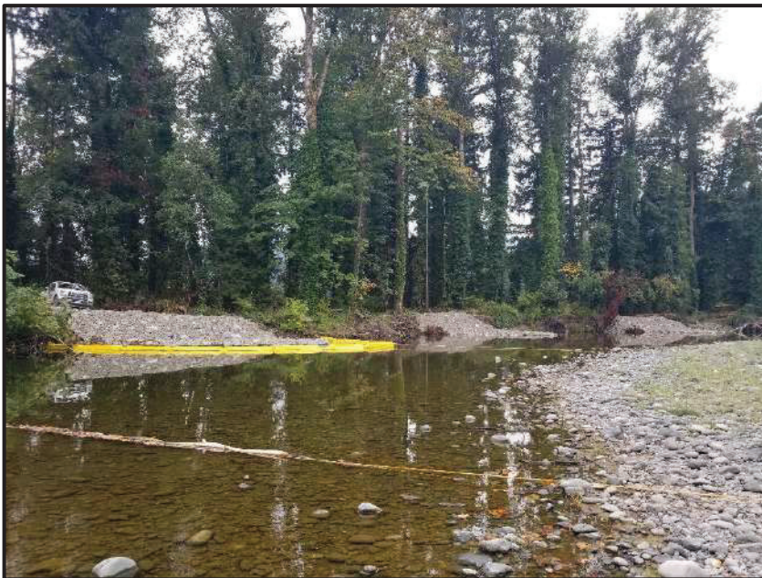
LOOKING UPSTREAM AT COMPLETED WEIRS 3, 4 AND 5.
