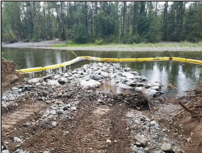
LOOKING TOWARDS WEIR 4 DURING THE CONSTRUCTION PROCESS.
