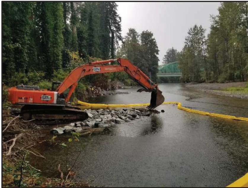
PLACEMENT OF RIPRAP AT THE OUTER EXTENT OF WEIR 4. THE PORTION OF THE WEIR CLOSEST TO THE RIVERBANK WAS USED AS A PLATFORM FOR THE EXCAVATOR TO ENSURE ADEQUATE REACH.
