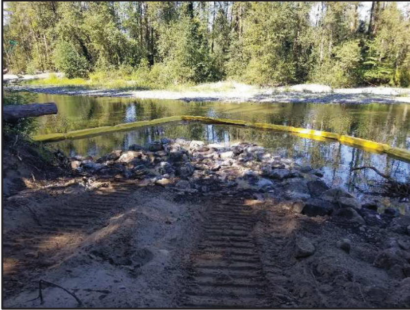
THE EXTENT OF WEIR 5.
