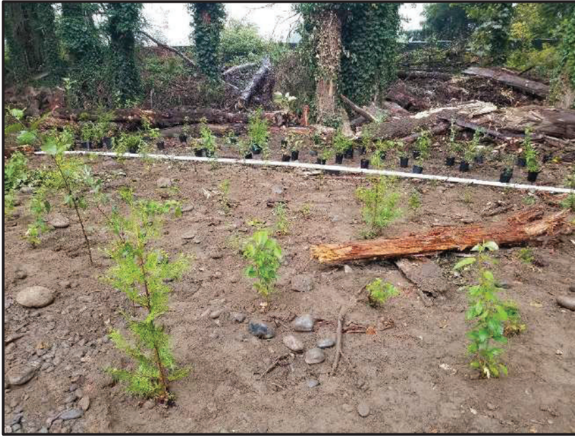
A PORTION OF THE TEMPORARY ACCESS ROAD CORRIDOR DURING THE REPLANTING PROCESS. NOTE THAT THE CREW DISTRIBUTED AND POSITIONED THE PLANTS IN APPROXIMATE LOCATIONS PRIOR TO PLANTING. THE WHITE PIPE IS PART OF THE TEMPORARY IRRIGATION SYSTEM THAT WAS INSTALLED.
