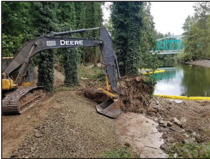
DRAIN ROCK PLACEMENT. RIPRAP WAS PLACED OVER THE BANK, LEADING DOWN TO THE WEIR.
