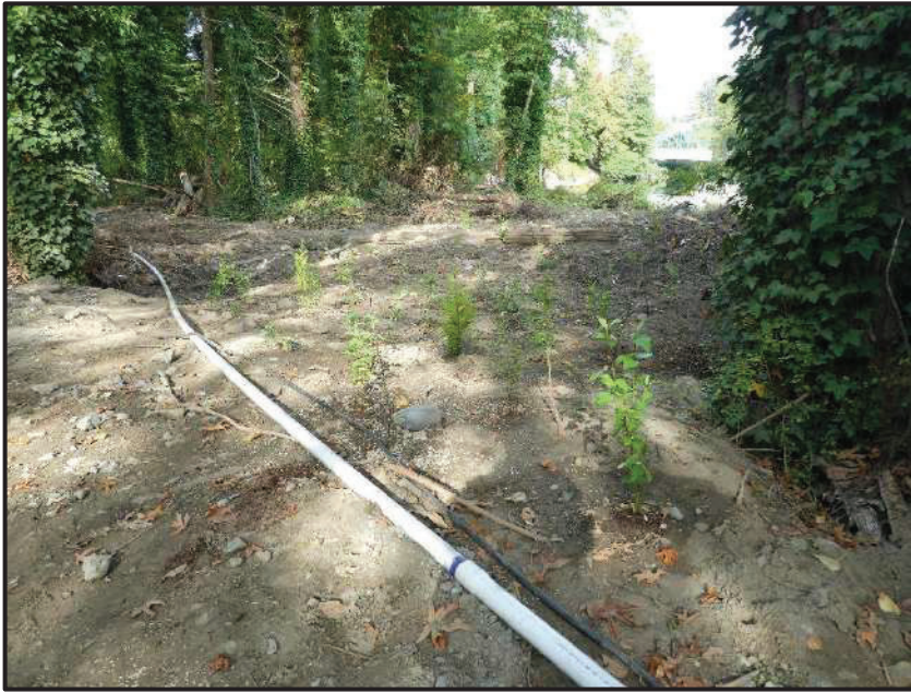
WEIR 5 AFTER UPON COMPLETION OF REPLANTING.
