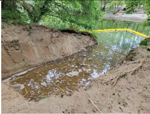
Photo 2: Weir #1 nearing completion
