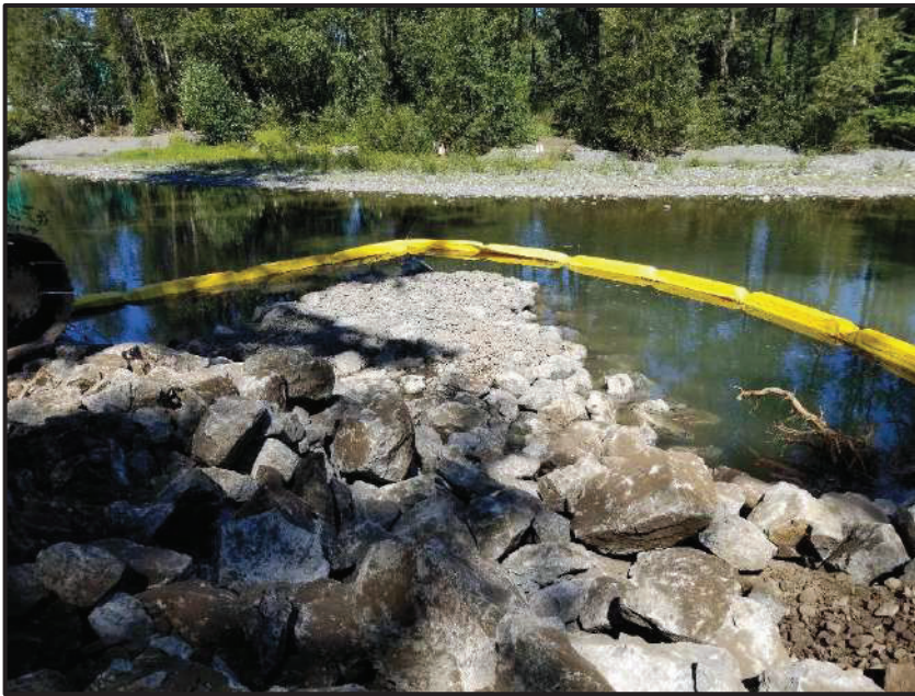
WEIR 5 UPON COMPLETION OF RIPRAP PLACEMENT AND LWD.
