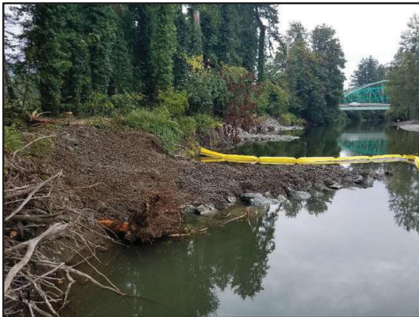
WEIR 4 UPON COMPLETION.
