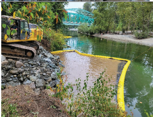
Photo 5: Weir #2 under construction
