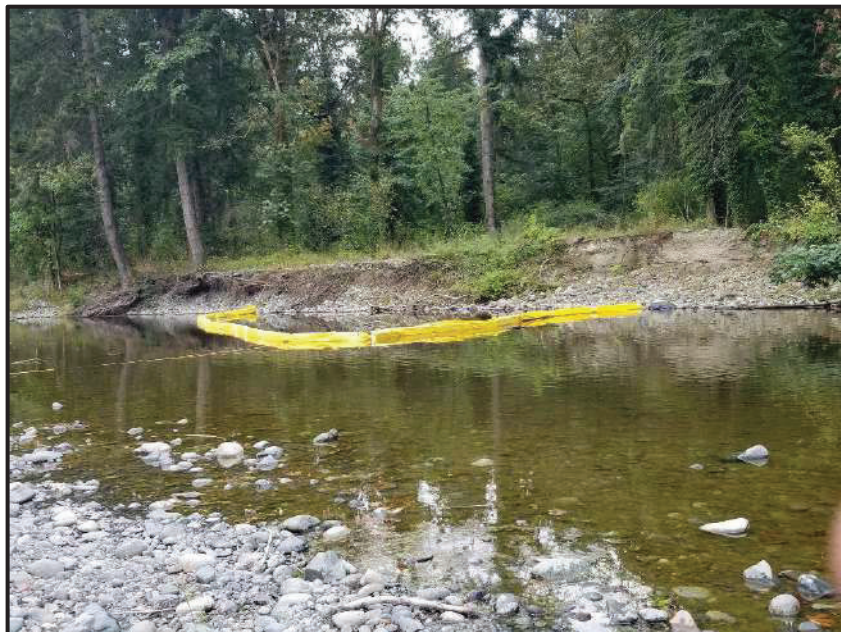
THE WEIR 6 ENCLOSURE PRIOR TO INITIATION OF BANK EXCAVATIONS.
