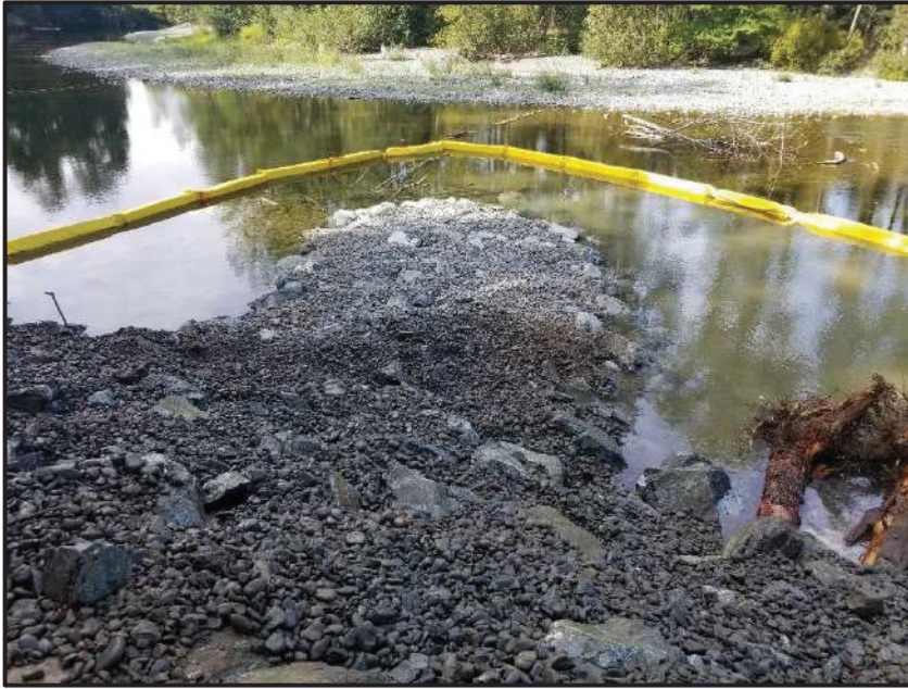
LOOKING DOWN AT WEIR 6 AFTER RIPRAP WAS CAPPED WITH D95 COBBLES.
