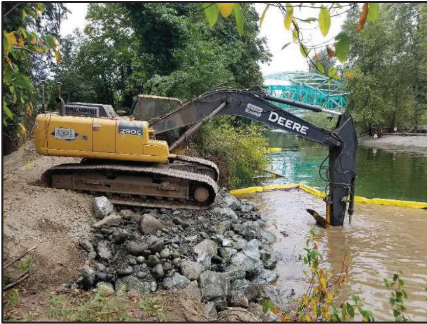
INSTREAM EXCAVATIONS THAT WERE REQUIRED TO CONSTRUCT THE BASE LAYER OF WEIR 2. NOTE THAT THE ROCK PLACED ALONG THE BANK WAS USED AS A PLATFORM FOR THE EXCAVATOR.
