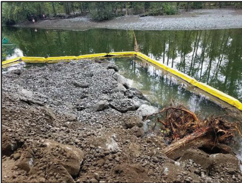
LOOKING DOWN AT WEIR 2 AFTER CONSTRUCTION WAS COMPLETED.
