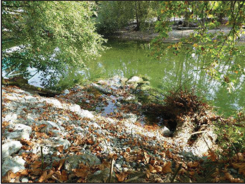
LOOKING DOWN AT WEIR 1 AFTER CONSTRUCTION WAS COMPLETED.
