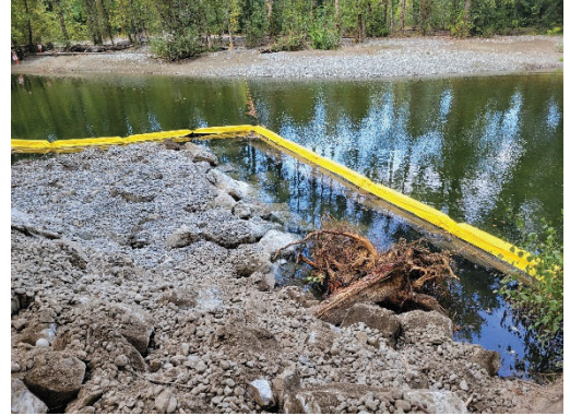
Photo 2: D84 on top of Weir #2
