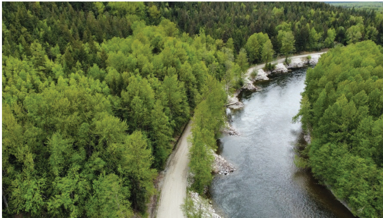
Photo 16: Example of Combination of Riparian Habitat with Rock Hard Points for Erosion
