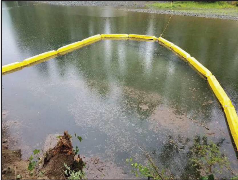
THE ENCLOSED WORK AREA FOR WEIR 3.
