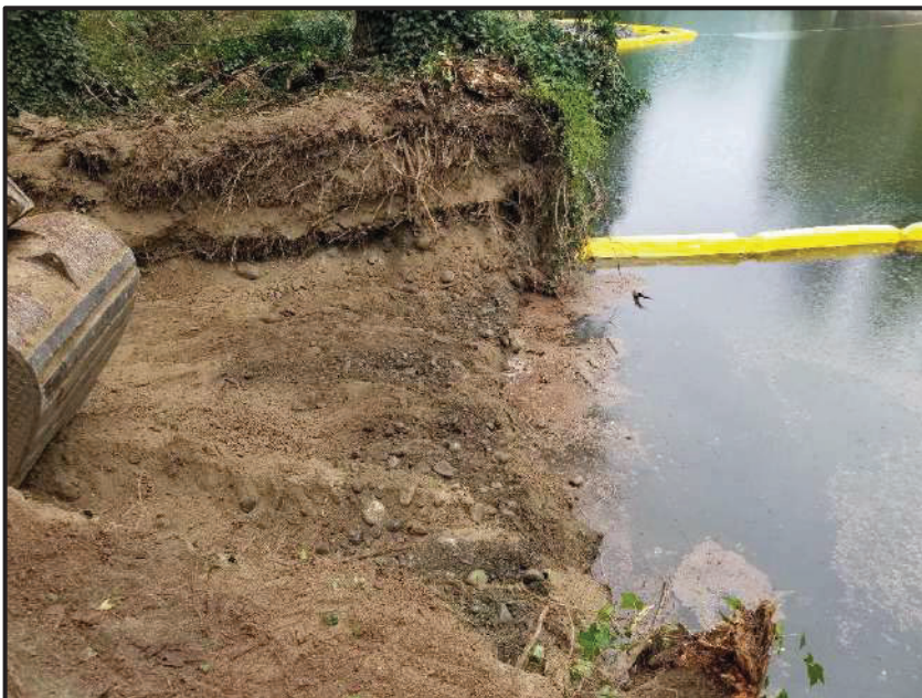
EXAMPLE OF DEPTH OF BANK EXCAVATION FOR WEIR 3. THE PURPOSE OF THE EXCAVATION WAS TO KEY RIPRAP INTO THE RIVERBANK.
