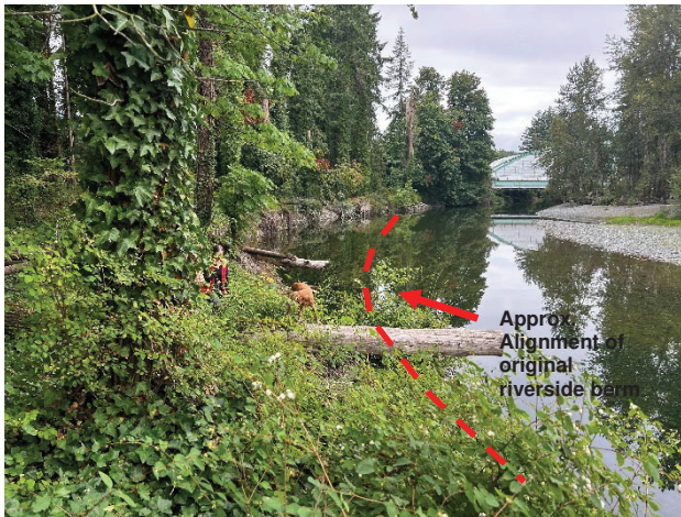
Photo 7: Right Bank of Chemainus River Downstream of Highway 1 Bridge Showing Approximate Alignment of Original Berm
