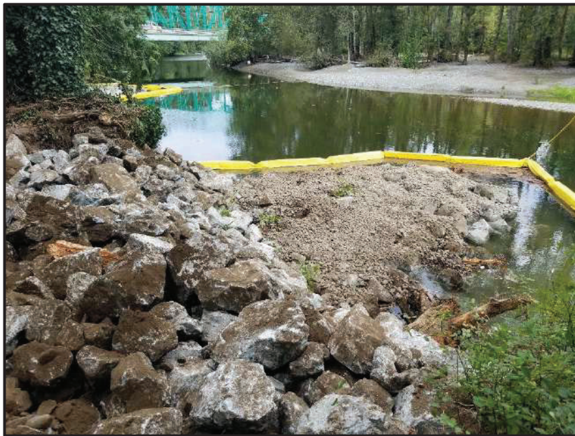
LOOKING DOWN AT THE COMPLETED WEIR 3 STRUCTURE.
