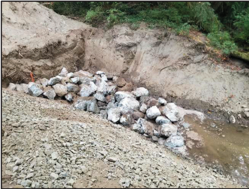
PLACEMENT OF RIPRAP IN THE EXCAVATED TRENCH.
