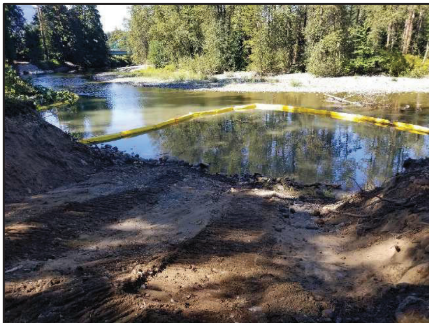
LOOKING DOWN THROUGH THE BANK EXCAVATION OF WEIR 6.
