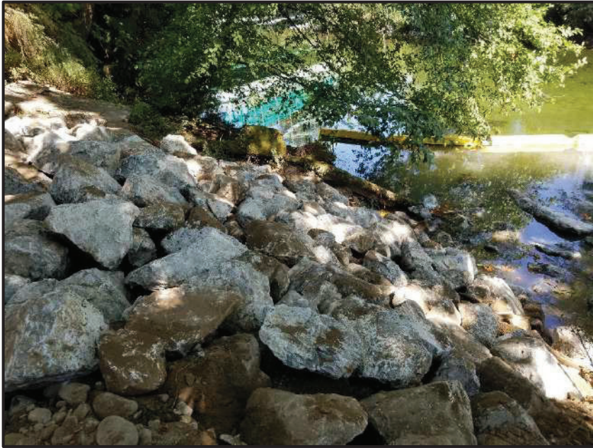
THE FACE OF WEIR 1 PRIOR TO BEING CAPPED WITH D95 COBBLES.
