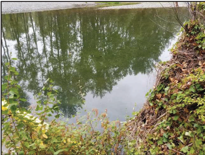
LOOKING DOWNSTREAM IMMEDIATELY BELOW THE ENCLOSED WORK ZONE. THE WATER OUTSIDE THE ISOLATED AREA REMAINED CLEAR FOR THE DURATION OF WEIR 2 CONSTRUCTION.
