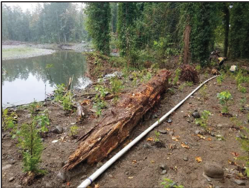
A FULLY RESTORED SECTION OF THE TEMPORARY ACCESS ROAD AREA ABOVE WEIR 2. NOTE THAT COARSE WOODY DEBRIS WAS ALSO DISTRIBUTED IN THE PLANTING AREA.
