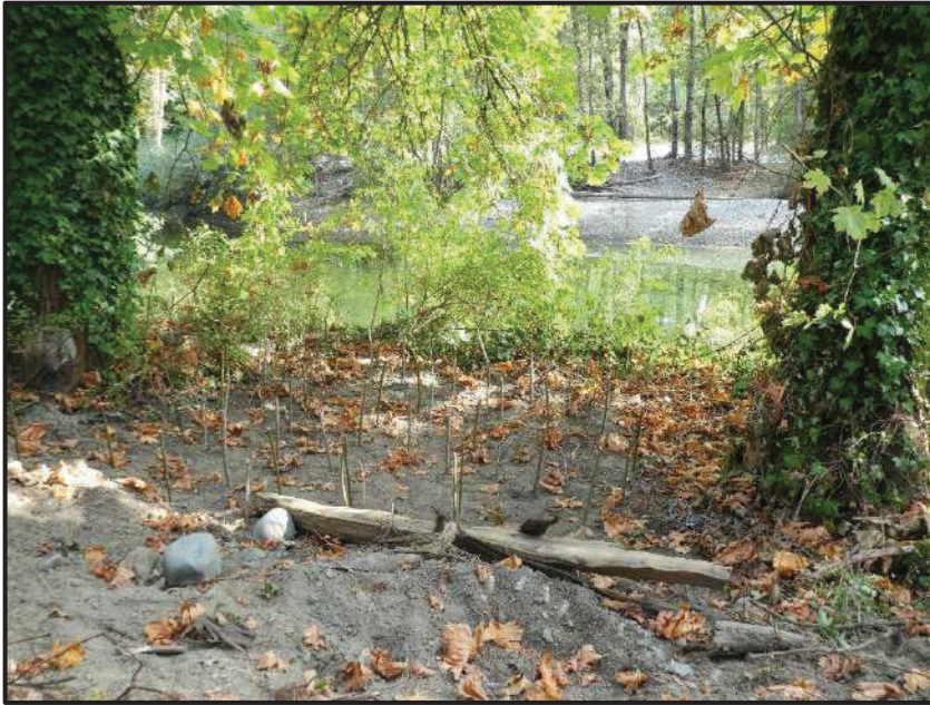
LIVE WILLOW LIVE STAKES THAT WERE INSTALLED ALONG THE UPPER EDGE OF WEIR 1.
