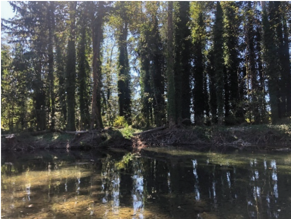
Photo 6: Right Bank of Chemainus River Downstream of Highway 1 Bridge Showing Mature Riparian Trees and Exposed Roots
