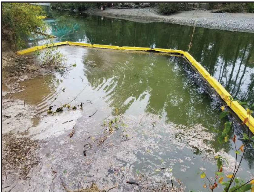
THE ENCLOSED WORK AREA FOR WEIR 2. TO ENSURE ADEQUATE WORKING AREA, A THIRD SILT CURTAIN WAS ATTACHED. NOTE THE SILT CURTAIN WAS EFFECTIVE IN CONTAINING TURBID WATER THAT WAS GENERATED DURING EXCAVATIONS.
