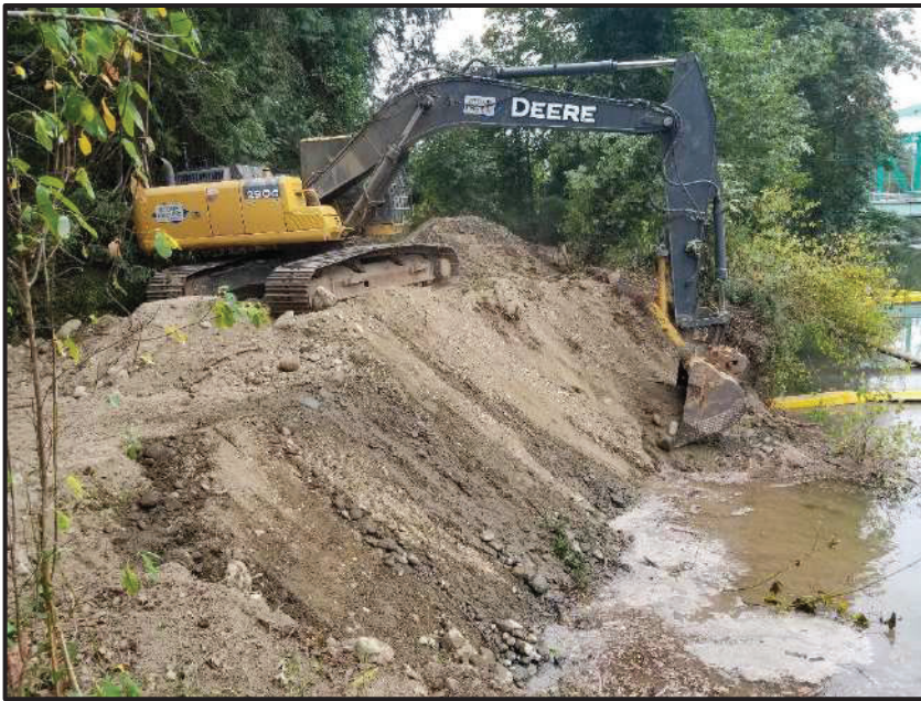
PREPARATION OF THE BANK FOR CONSTRUCTION OF WEIR 2. EXCAVATIONS WERE REQUIRED TO ACHIEVE THE REQUIRED SLOPE PRIOR TO PLACEMENT OF RIPRAP.
