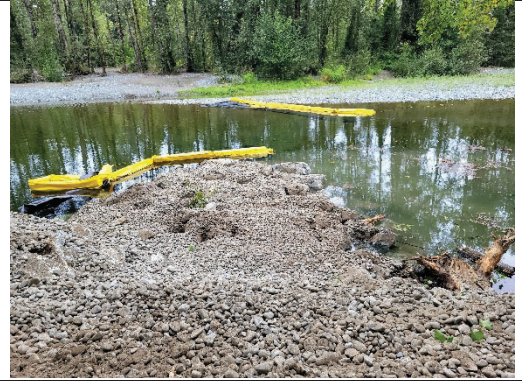
Photo 4: Weir #3 completed with D84 and LWD, isolation being removed
