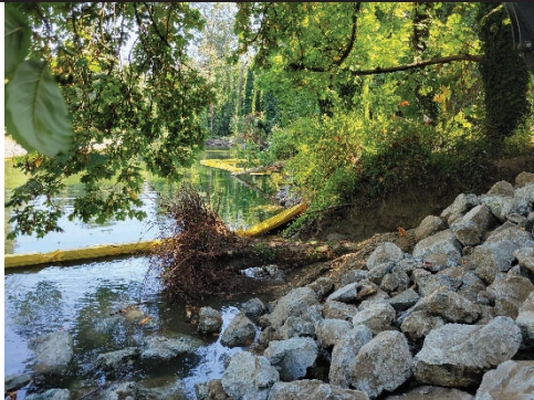
Photo 4: D84 material install
