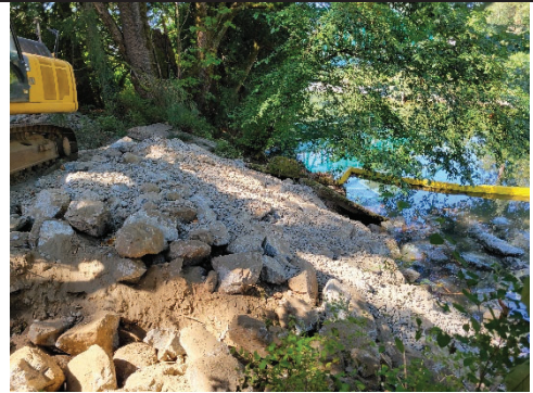
Photo 4: D84 material install
