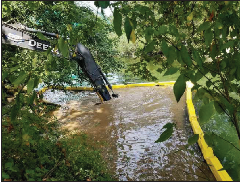
EXCAVATIONS AS PART OF WEIR CONSTRUCTION. A TRENCH WAS DUG OUT TO ALLOW FOR THE BASE LAYER OF RIPRAP TO BE PLACED AND CREATE STABILITY FOR THE WEIR.
