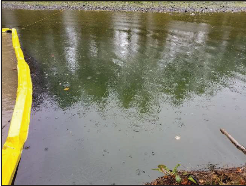
SILT CURTAIN DURING CONSTRUCTION OF WEIR 4. NOTE THAT THE DIRTY WATER WAS CONTAINED BY THE CURTAIN.
