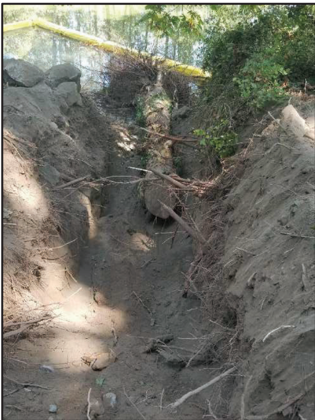
LOOKING DOWN AT THE LWD THAT WAS PLACED IMMEDIATELY DOWNSTREAM OF THE WEIR TO INCREASE AQUATIC HABITAT COMPLEXITY.
