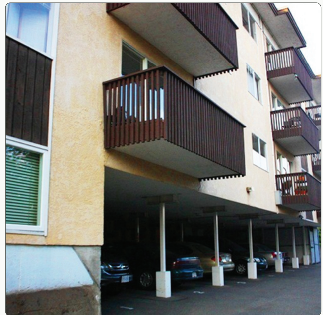
Figure 5.6.3: Apartment buildings with tuck-under parking are especially vulnerable to ground shaking and ground failure.
