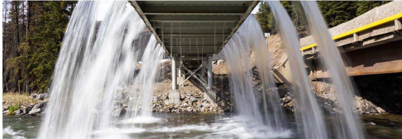
Figure 6. Swift and Cataract Creek Outfall Structure. This water is dosed with antiscalant to neutralize Swift and Cataract Creeks as a source of calcite to the Fording River.
