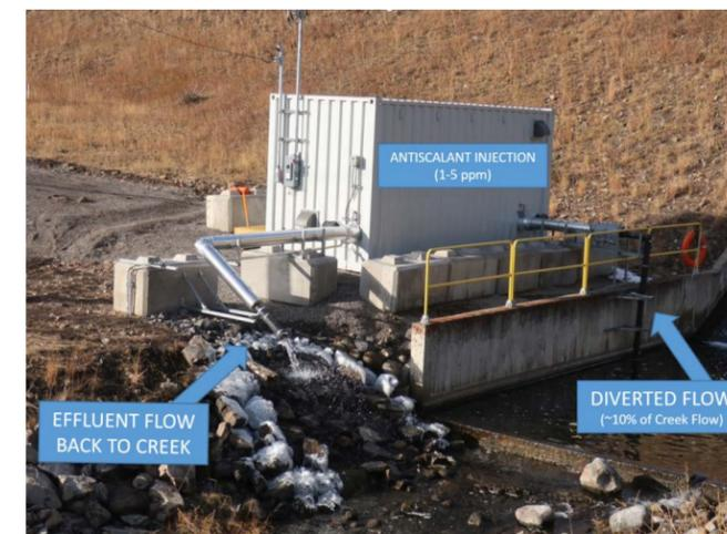
Figure 10. Antiscalant Addition Module at Lower Greenhills Creek.
